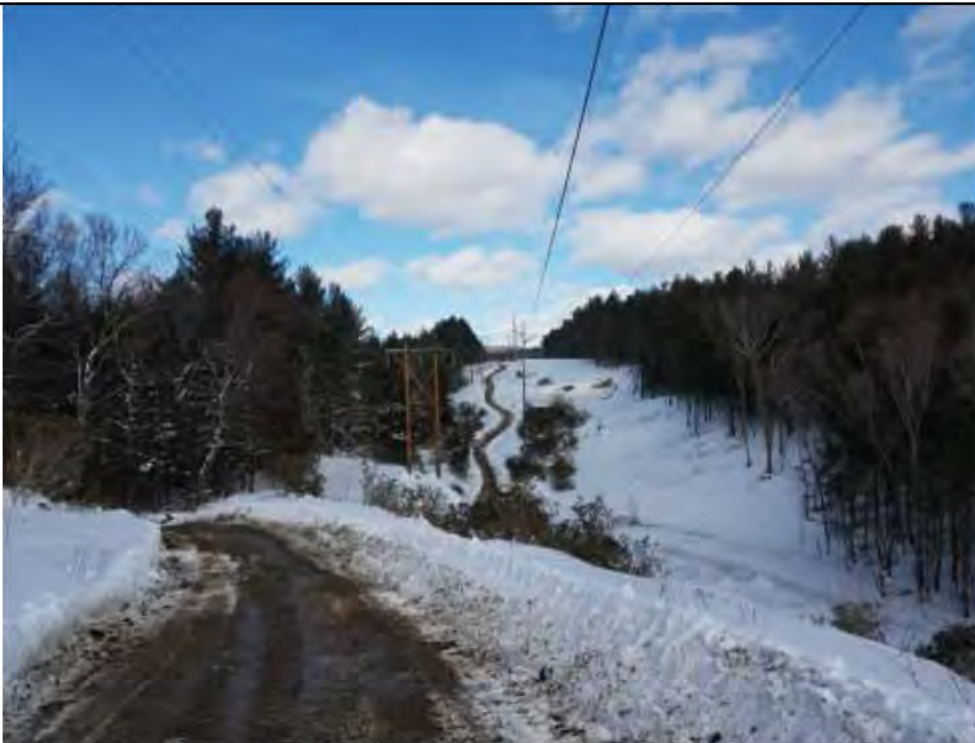
Photo 18: 2/10/2017, Harwinton: Access road snow clearing.
