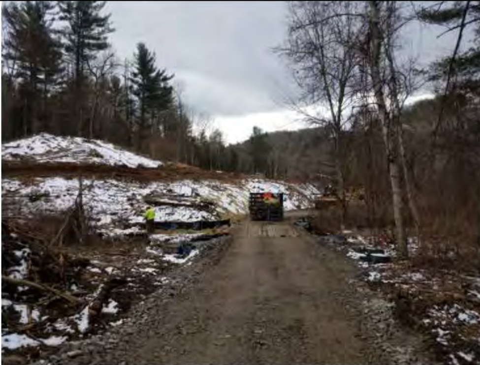
Photo 9: 2/2/2017, Harwinton: Access road construction and watercourse crossing (S-F10) completed.
