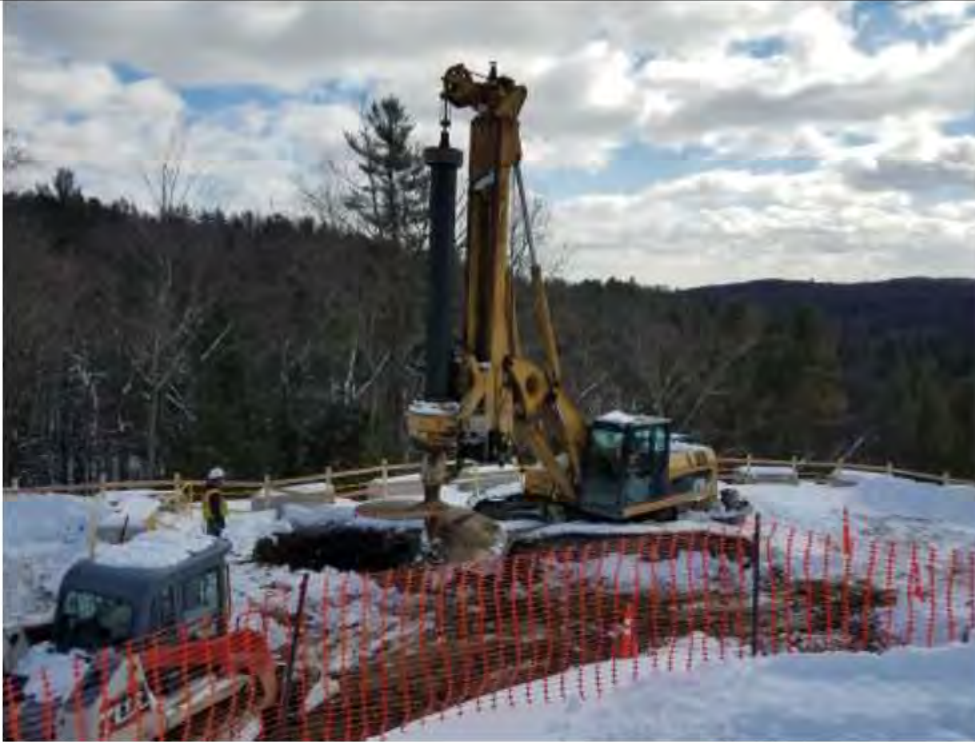
Photo 17: 2/10/2017, Harwinton: Str88 Pad drilling.
