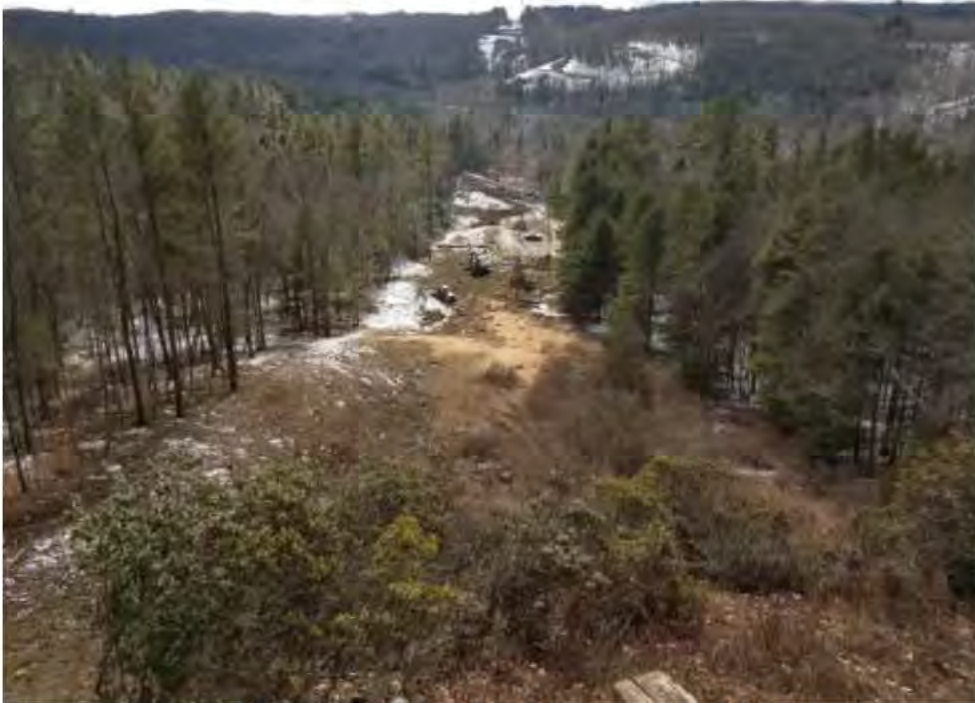
Photo 7: 2/2/2017, Harwinton: Clearing between Str88 and Str87 completed, Str87 in the distance.
