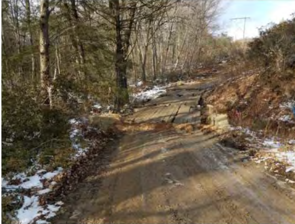
Photo 15: 2/2/2017, Watertown: Timber mats used to stabilize road at C-14.
