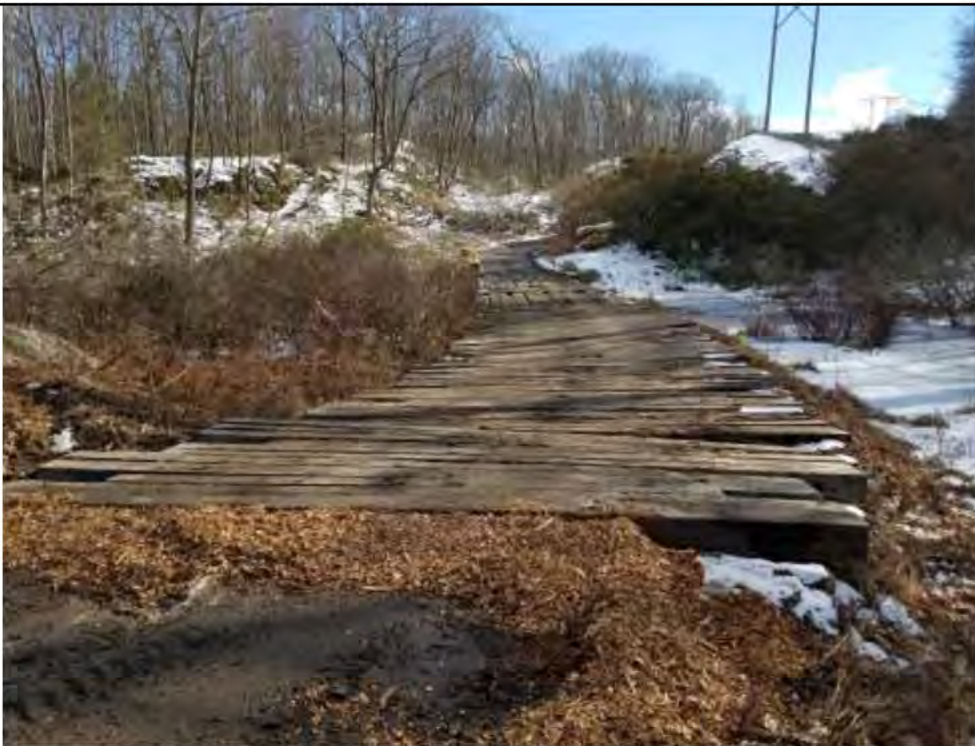
Photo 14: 2/2/2017, Watertown: Timber mats used to stabilize road at C-12-1.
