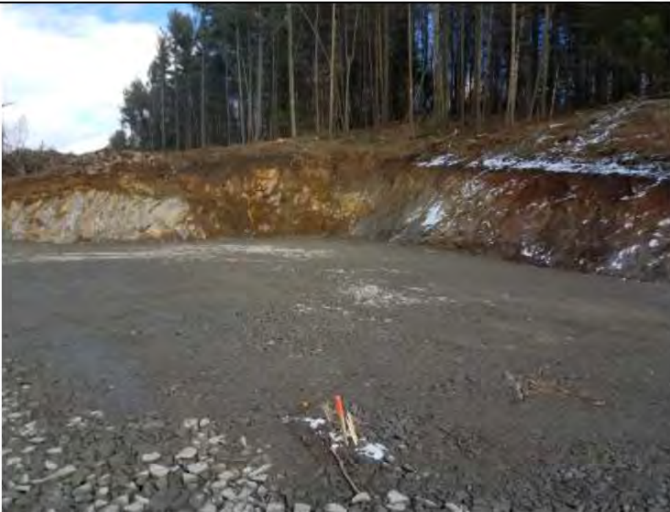
Photo 6: 2/2/2017, Harwinton: Str90 pad construction completed.
