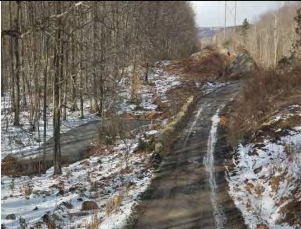
Photo 13: 2/2/2017, Watertown: Access road from Str24 through Str46 E&S controls.
