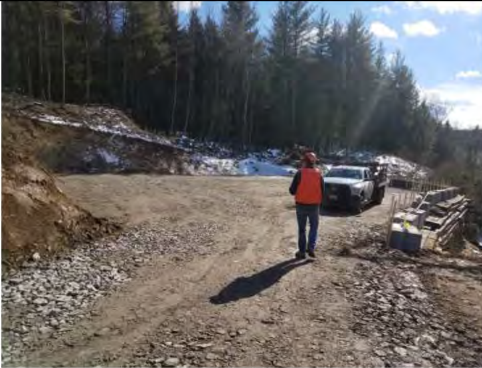
Photo 3: 2/2/2017, Harwinton: Str90 pad construction completed.
