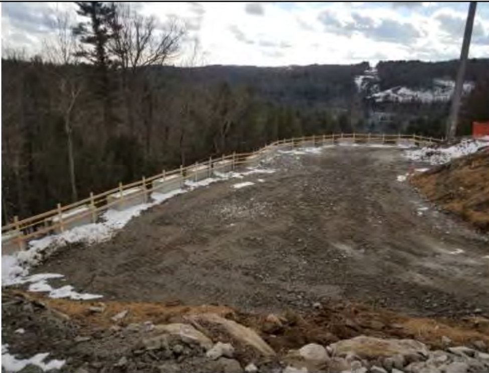
Photo 8: 2/2/2017, Harwinton: Str88 pad construction completed.
