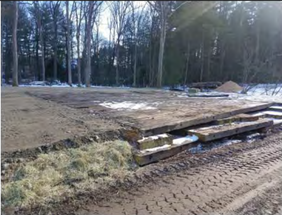
Photo 2: 2/2/2017, Harwinton: Str93 pad construction, timber mats placed over W-F14.
