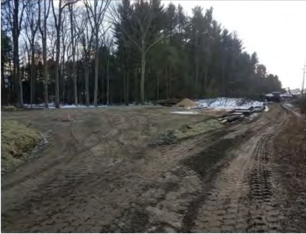
Photo 1: 2/2/2017, Harwinton: Str93 pad construction.
