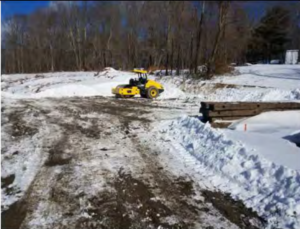
Photo 19: 2/10/2017, Litchfield: Str74 pad and access road snow clearing.
