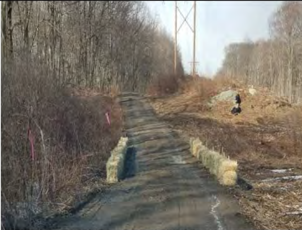
Photo 12: 2/2/2017, Watertown: Access road from Str24 through Str46 E&S controls.
