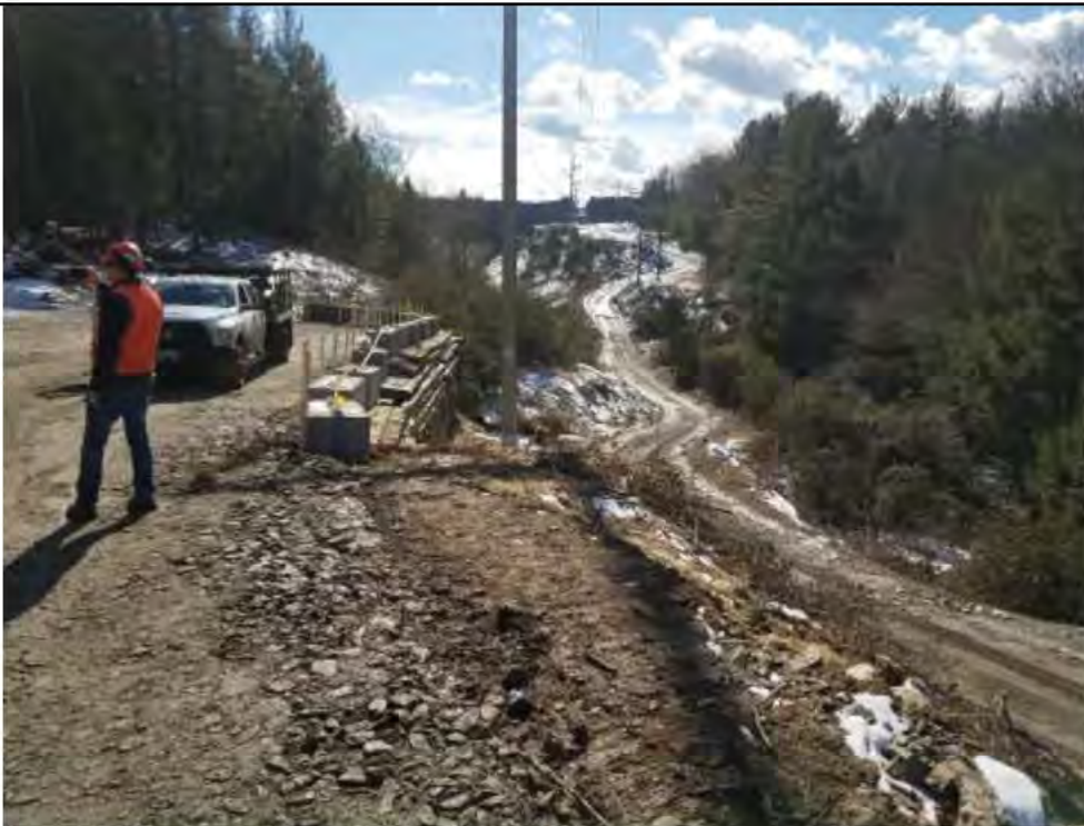
Photo 4: 2/2/2017, Harwinton: Str90 pad construction completed.
