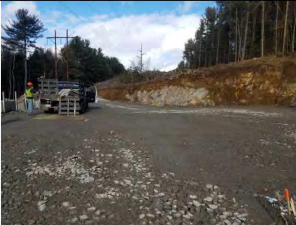
Photo 5: 2/2/2017, Harwinton: Str90 pad construction completed.
