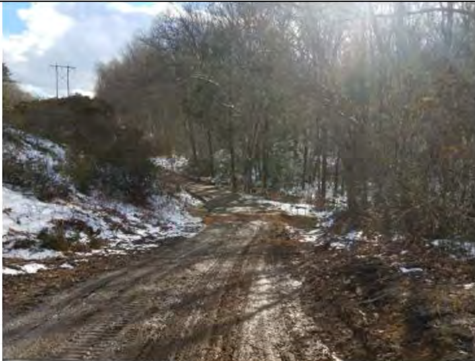
Photo 16: 2/2/2017, Watertown: Access road maintenance performed.
