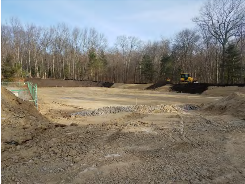
Photo #1: 1/5/17: Harwinton, Map 35, Campville Substation Expansion progress
