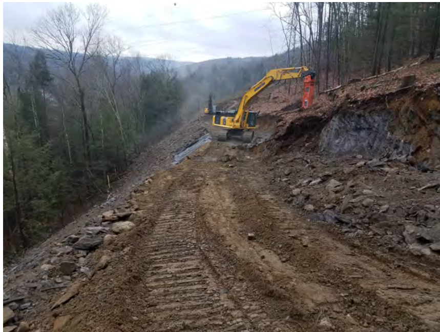
Photo #12: 1/12/2017: Litchfield, Map 31, access road construction to Str86
