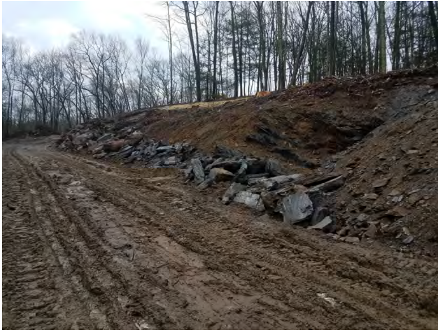
Photo #11: 1/12/2017: Litchfield, Map 31, access road construction to Str86
