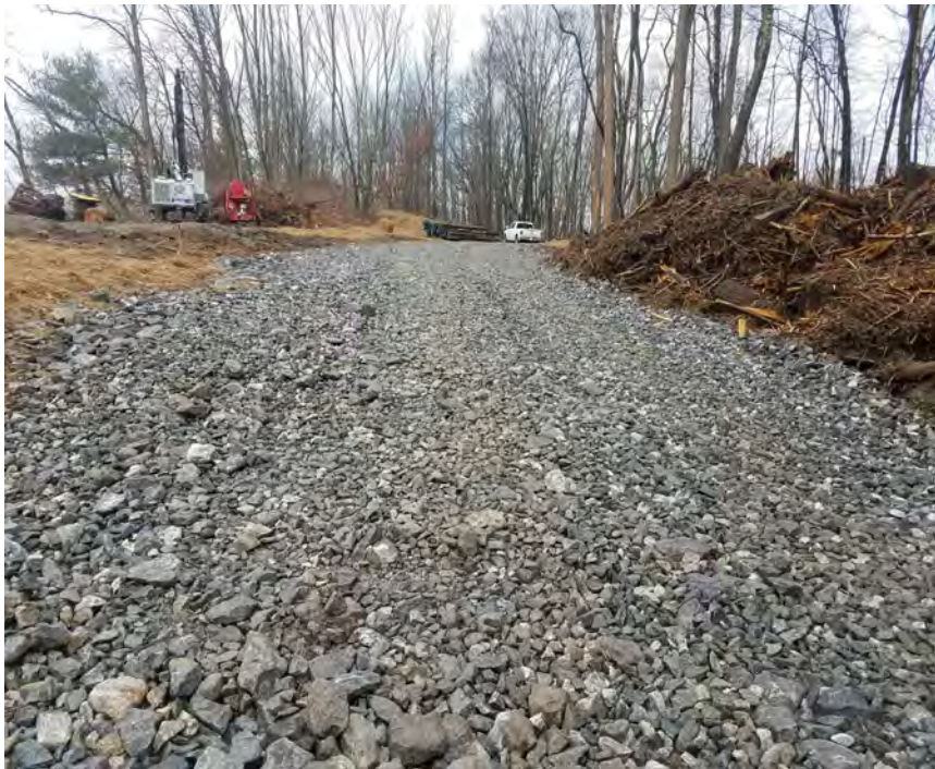
Photo #10: 1/12/2017: Litchfield, Map 31, access road construction to Str86
