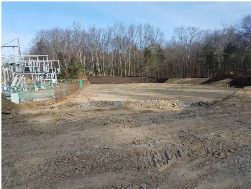
Photo #2: 1/5/2017: Harwinton, Map 35, Campville Substation Expansion progress
