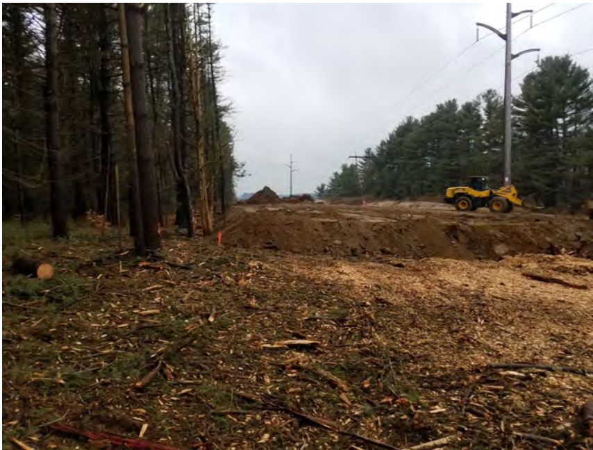
Photo #8: 1/12/2017: Harwinton, Map 33, Str90 pad construction in progress
