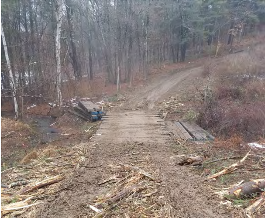
Photo #9: 1/12/2017: Harwinton, Map 32, temporary water crossing, proposed culvert area
