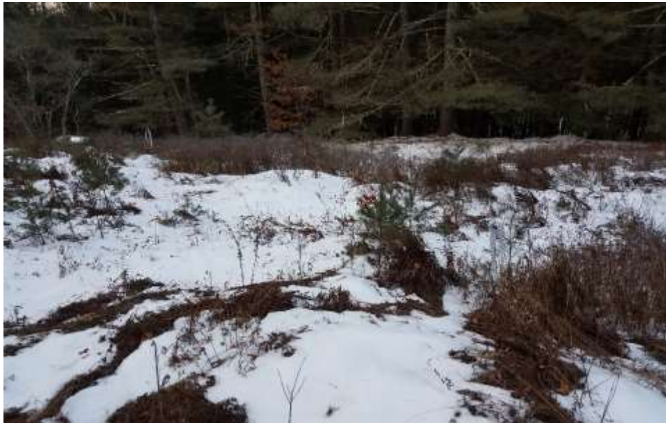
Photo #10: 12/21/16- ROW clearing, area of Str92 through Str95, flagged sensitive area
