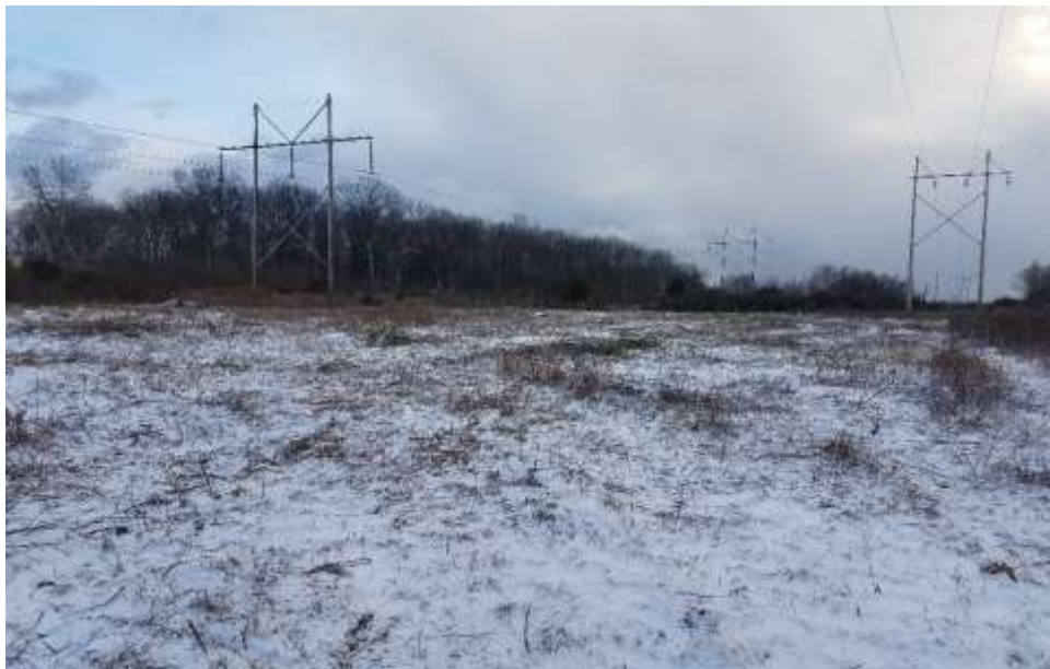
Photo #2: 12/15/16-ROW clearing, area of Str 16 through 18
