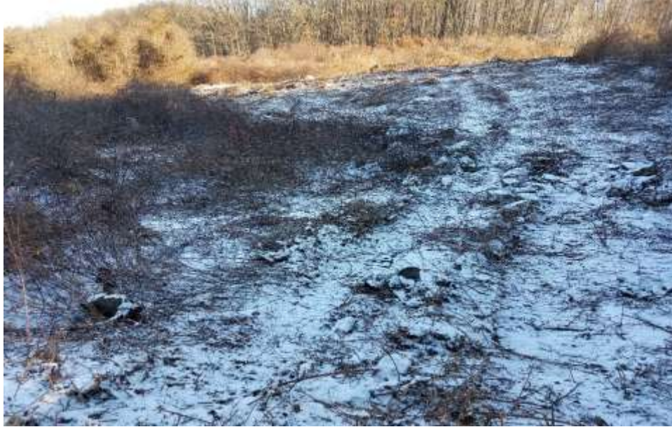
Photo #3: 12/15/16-ROW clearing, area of Str 21 through 23
