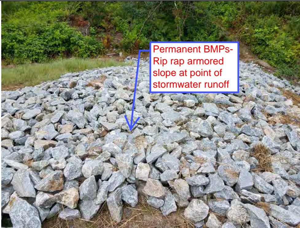
Photo 21: 08/17/2018: Thomaston, Map 18, Structure Str 51, Permanent BMPs- rip rap armored slope at point of stormwater runoff.
