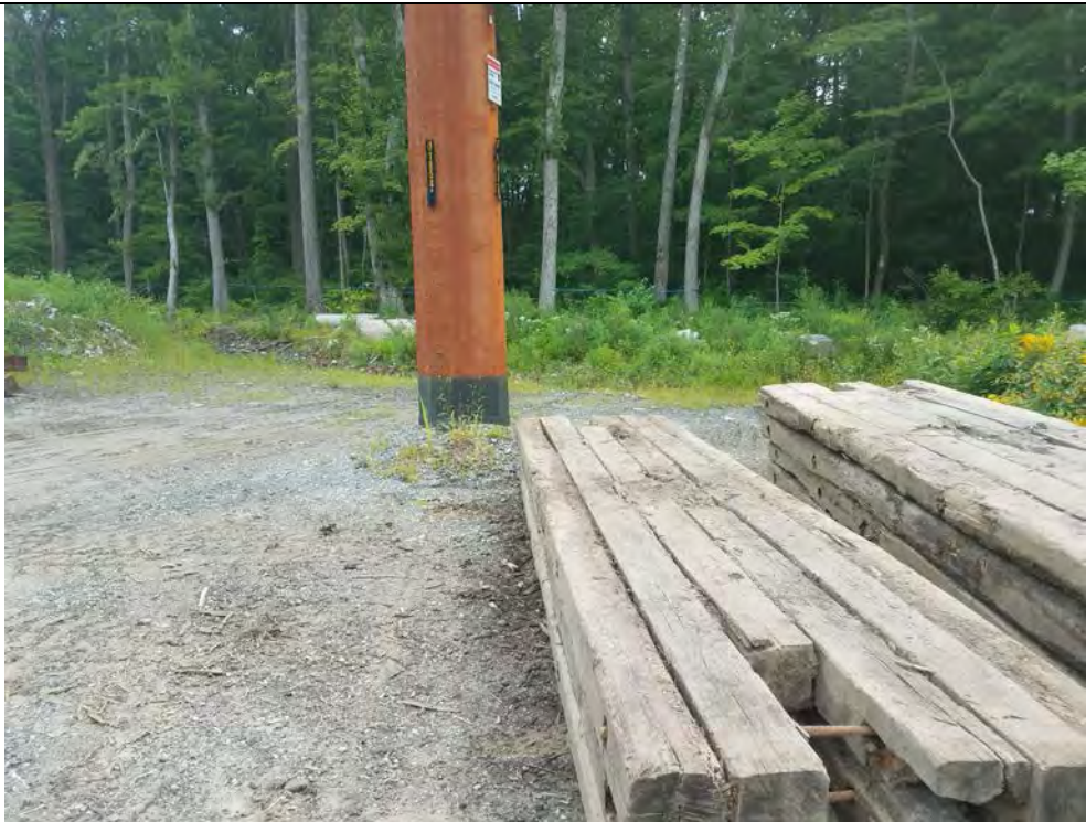
Photo 32: 08/17/2018: Litchfield, Map 26, Structure Str 75, timber mats left behind after removal at water crossing.
