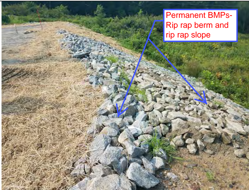
Photo 2: 08/16/2018: Watertown, Map 03, Structure Str 7, Permanent BMPs- rip rap berm and rip rap armored slope at point of stormwater runoff.
