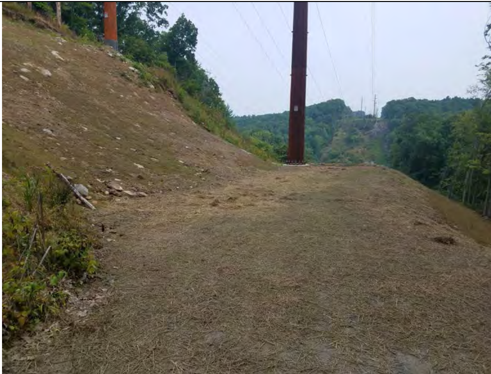
Photo 28: 08/17/2018: Thomaston, Map 24, Structure Str 69, seeding and straw mulch cover on pad.
