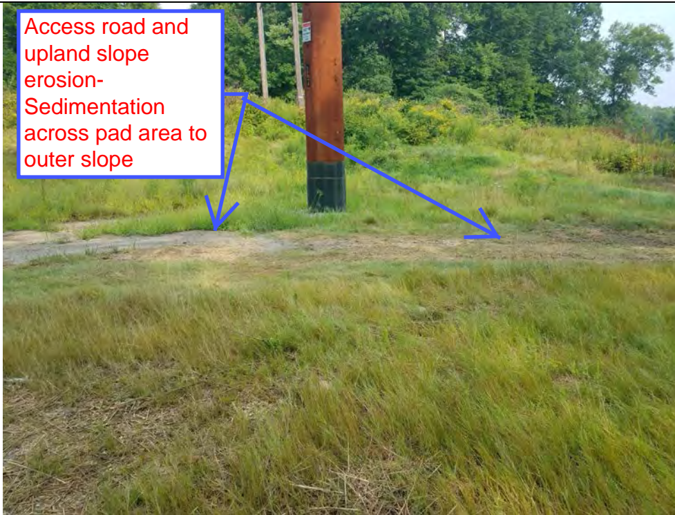
Photo 22: 08/17/2018: Thomaston, Map 20, Structure Str 57, erosion area and vegetation growth on pad, permanent BMP- rip rap slope (not shown) at point of stormwater runoff.
