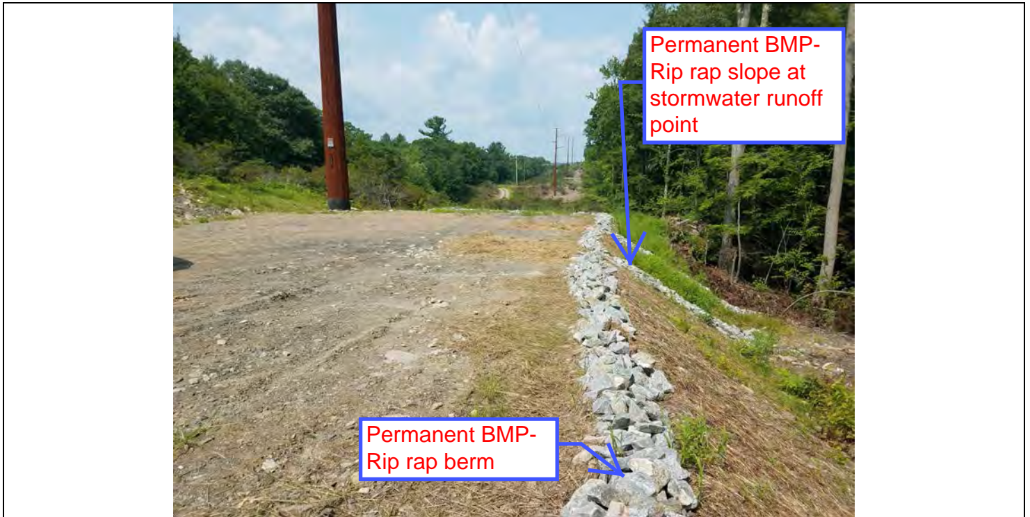
Photo 11: 08/16/2018: Watertown, Map 12, Structure Str 34, implemented Permanent BMPs- rip rap berm and rip rap armored slope at points of stormwater runoff.
