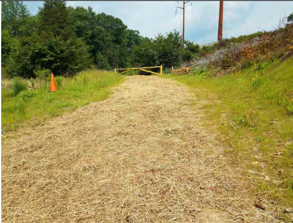
Photo 37: 08/17/2018: Litchfield, Map 30, Structure Str 85, seeding and straw mulch on access road.
