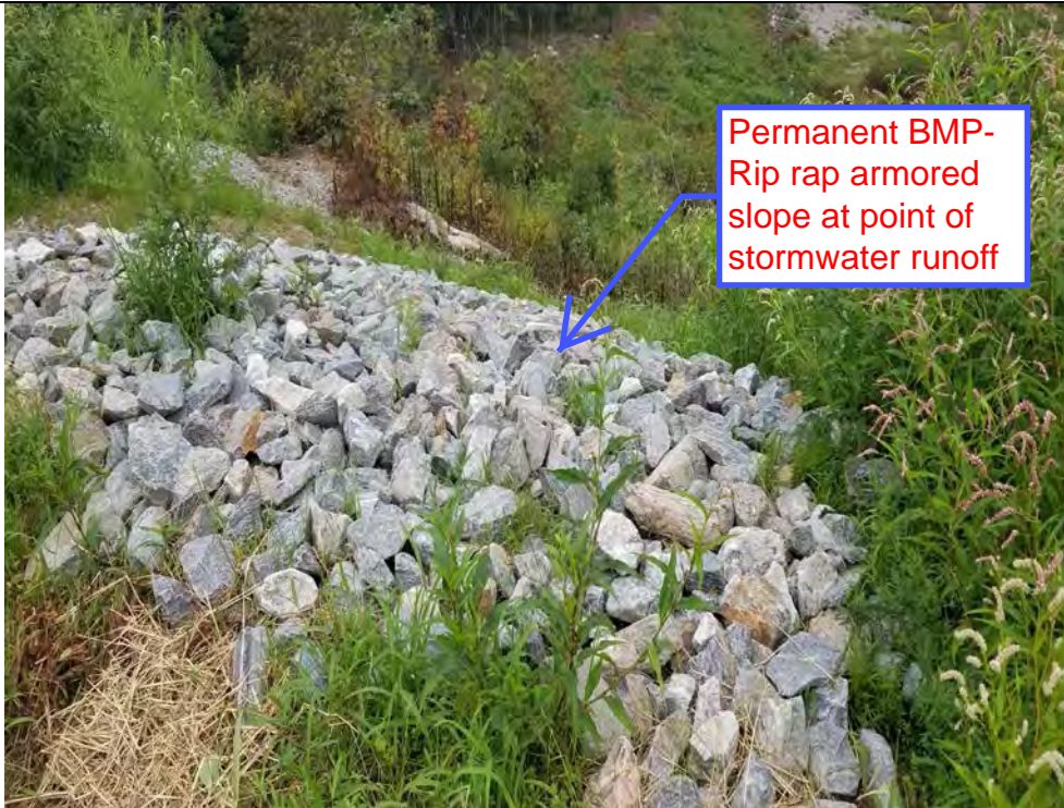
Photo 43: 08/17/2018: Harwinton, Map 32, Structure Str 88, Permanent BMPs- rip rap armored slope at points of stormwater runoff, vegetation growth.
