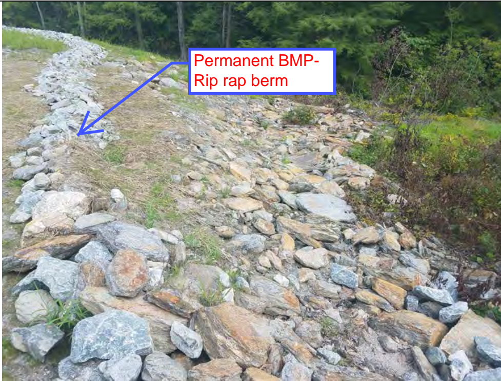
Photo 13: 08/16/2018: Watertown, Map 11 Structure, Str 38, implemented Permanent BMPs- rip rap berm.
