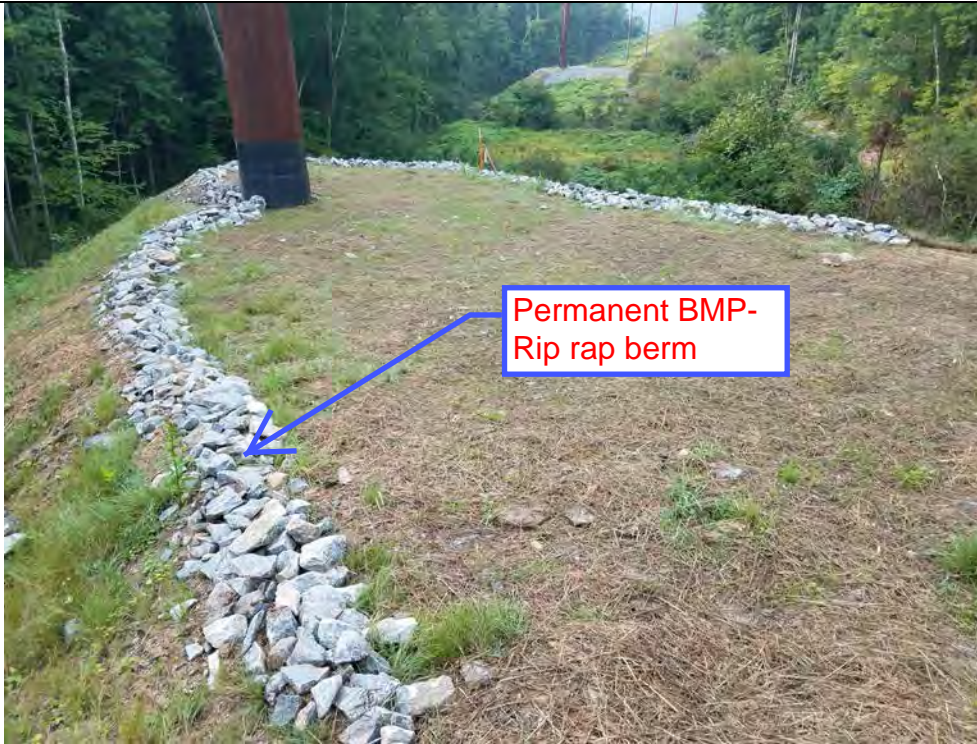
Photo 19: 08/17/2018: Thomaston, Map 18, Structure Str 51, permanent BMPs- rip rap berm.
