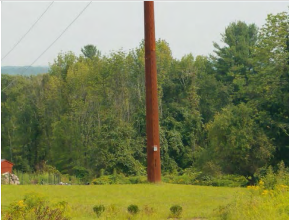
Photo 34: 08/17/2018: Litchfield, Map 29, Structure Str 82, vegetation growth.
