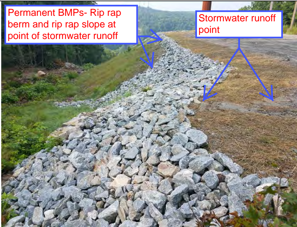
Photo 18: 08/17/2018: Thomaston, Map 17, Structure Str 49, Permanent BMPs- rip rap berm and rip rap armored slope at point of stormwater runoff.
