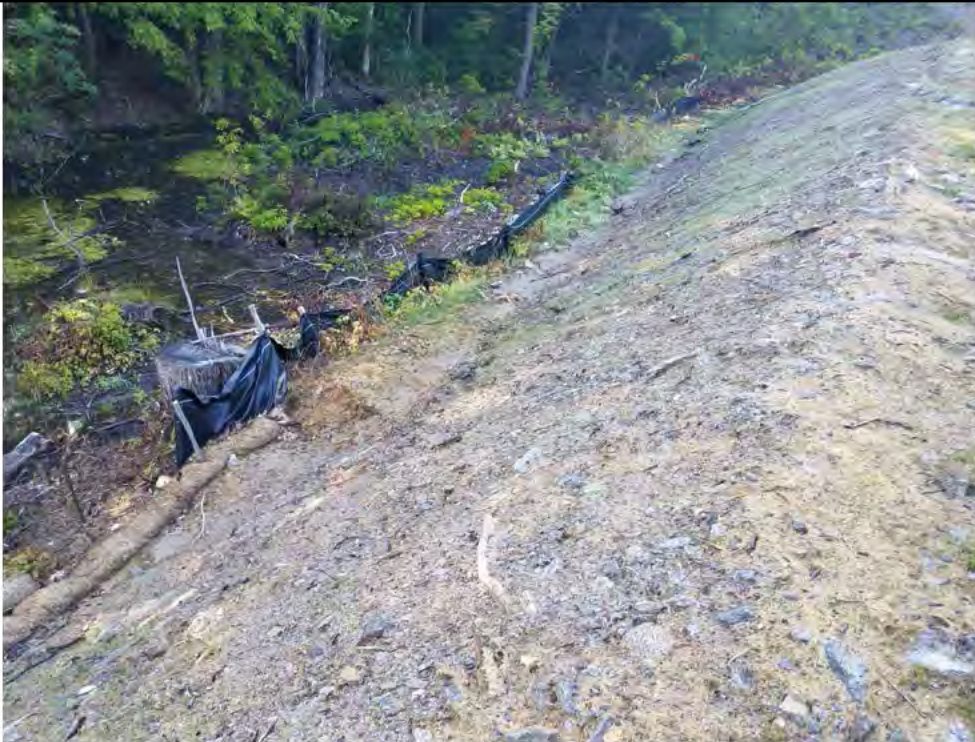
Photo 29: 07/27/2018, Watertown: Map 14, Str39, continued erosion of east slope abutting wetland/vernal pool W-C20/VP-C20-1. Photo taken facing east. Silt Fence Maintenance is needed per the BMPs. See Photo 30 for additional view.
