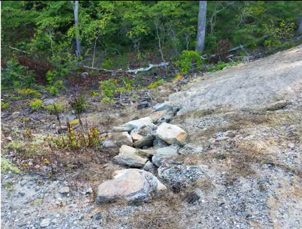
Photo 27: 07/27/2018, Watertown: Map 13, Str38, continued erosion of north slope and sediment buildup at toe of slope. Photo taken facing east from the access road toward wetland south end of W-C20. See Photo 28 for additional view.
