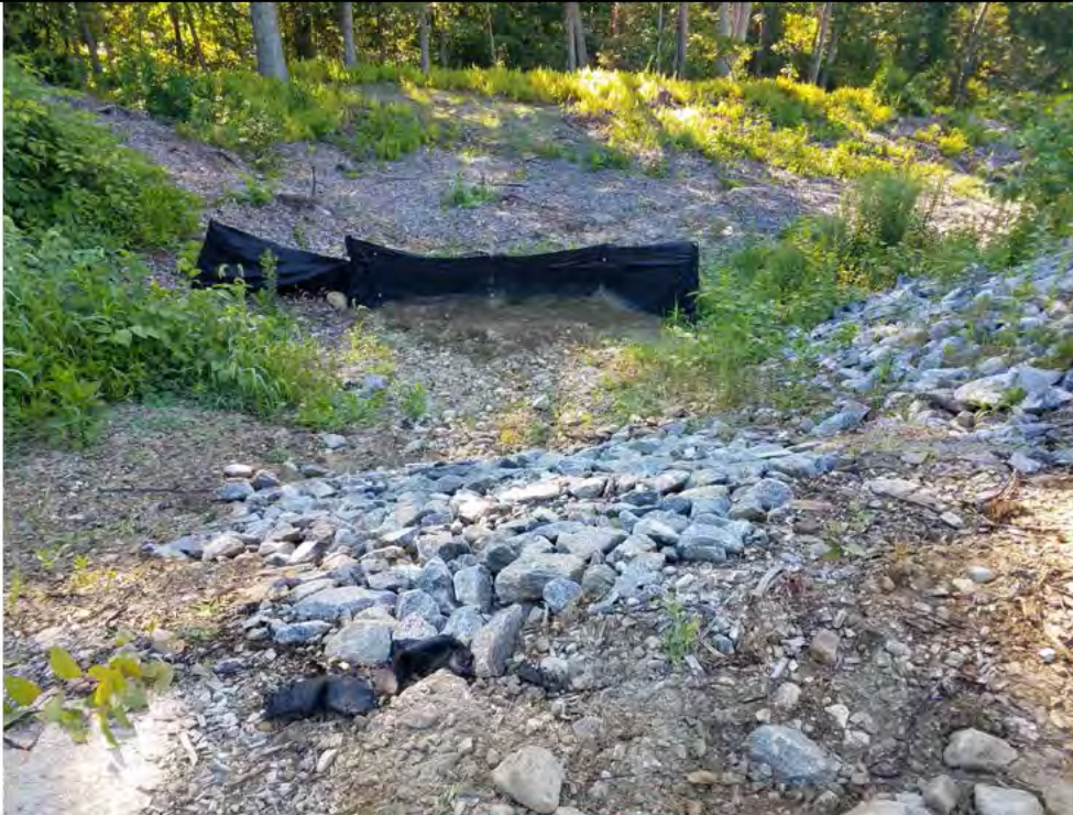
Photo 1A: 07/20/2018, Watertown: Map 01, Str1A, CORRECTIVE ACTION - Rip rap armored slope in erosion area shown in Photo 1, cleared sediment buildup on silt fence and reset silt fence.
