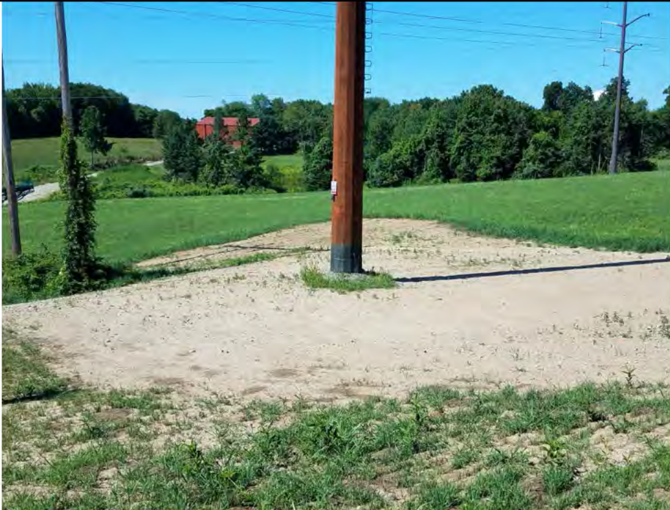
Photo 5: 07/20/2018, Watertown: Map 05, Str13, property owner interference with initial restoration/stabilization measures. This area is reportedly not going to be restored by the project.
