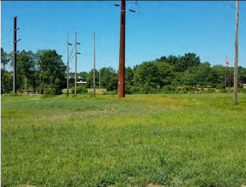
Photo 4: 07/20/2018, Watertown: Map 06, Str14, stabilization measures successful, no erosion visible.
