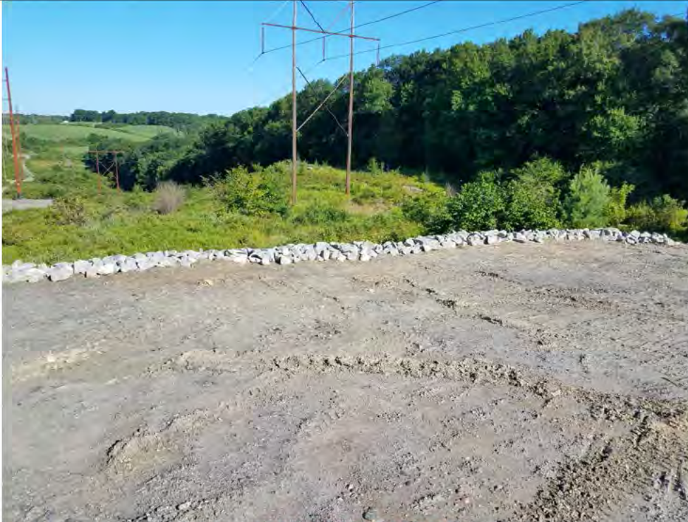
Photo 2D: 07/20/2018, Watertown: Map 03, Str07, CORRECTIVE ACTION - Rip rap berm along top of pad, upland of slope erosion shown in Photos 2 and 2B.
