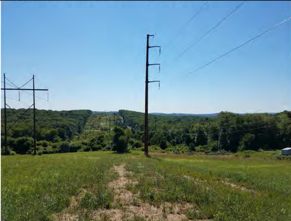
Photo 6: 07/20/2018, Watertown: Map 02, Str12, stabilization measures in progress, no erosion visible.
