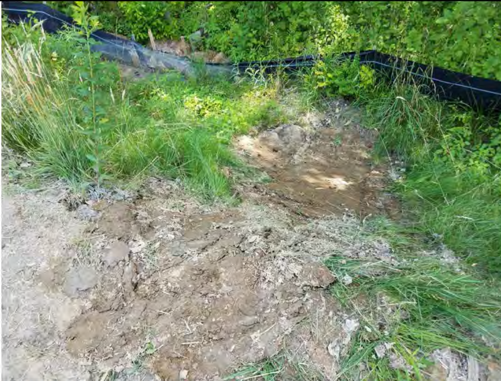
Photo 32: 07/13/2018, Litchfield: Map 29, Str83, erosion area graded but not stabilized on the down gradient slope (east side of work pad). Photo taken facing east towards W-F4 from the Str8 work pad.
