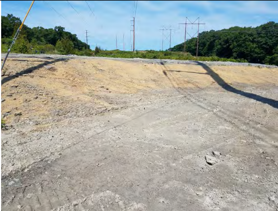
Photo 23: 07/13/2018, Watertown: Map 04, Str05 slope stabilization. Hydro seed applied to the upland slope, erosion area shown previously in Photo #3. Photo taken facing south (opposite view of Photo 3).
