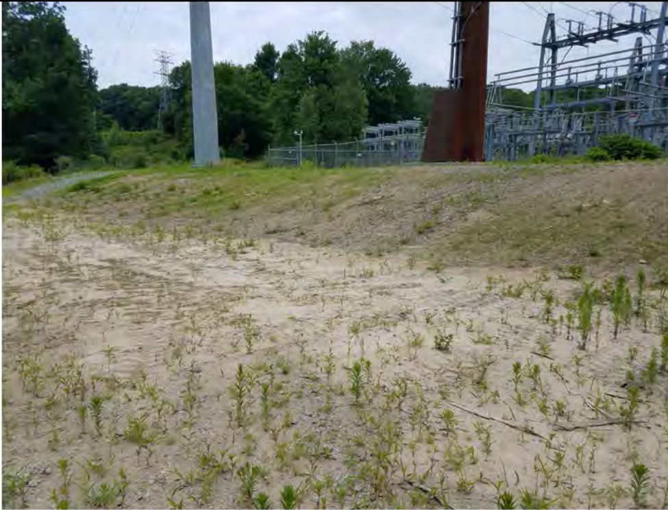
Photo 1: 07/06/2018, Watertown: Map 01, Str1A pad and pad slope erosion, minimal vegetation cover. Photo taken facing southeast toward Str1A.
