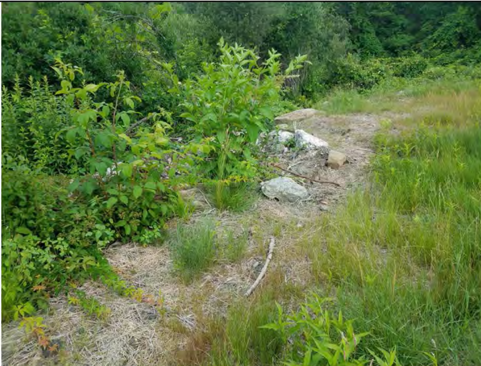
Photo 12: 07/06/2018, Watertown: Map 09, Str23 pad stabilization. Photo taken facing north.
