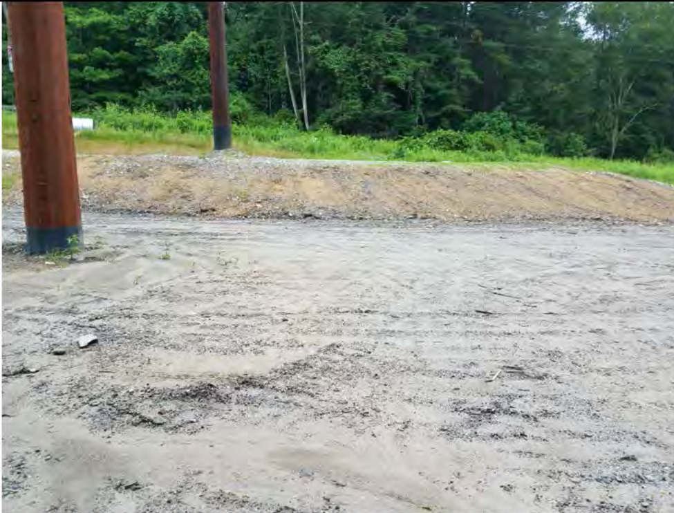
Photo 15: 07/06/2018, Litchfield: Map 29, Str83, fine sediments continue to wash out of exposed, unstabilized/unvegetated soils during rain events. Photo taken facing west.
