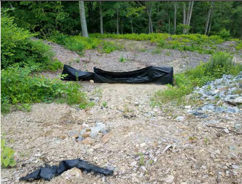
Photo 2: 07/06/2018, Watertown: Map 01, Str1A pad slope erosion, no stabilization. Photo taken facing north CT wetland.
