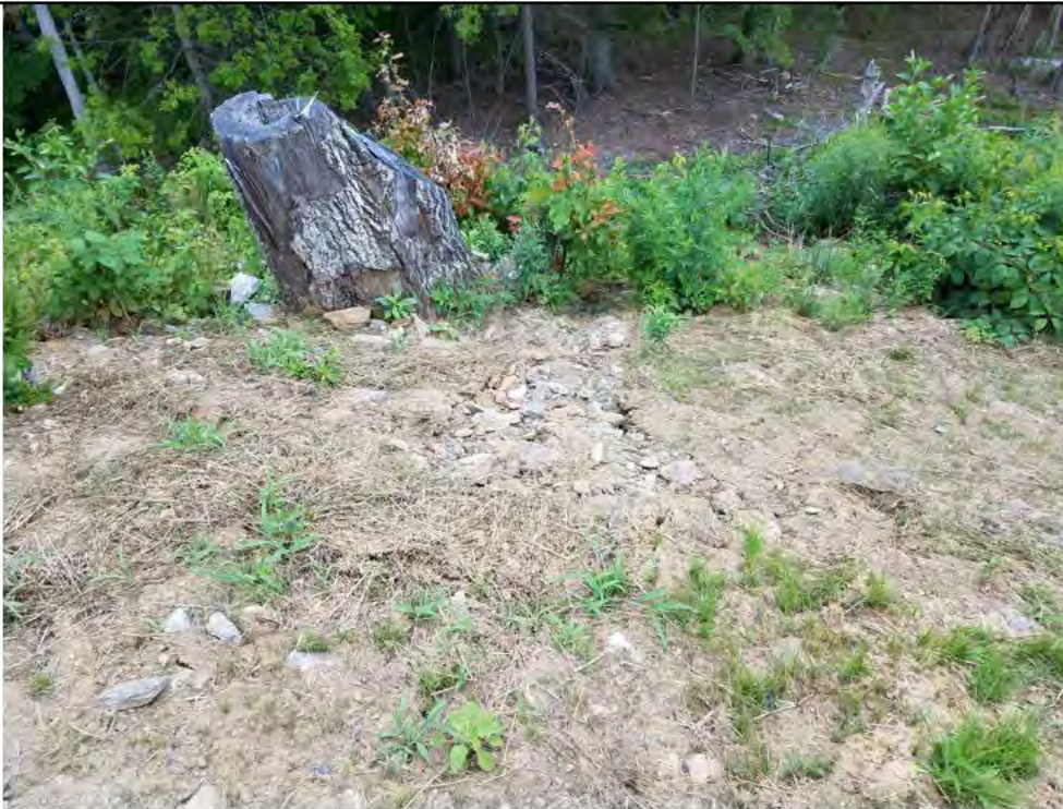
Photo 33: 07/13/2018, Harwinton: Map 32, Str88 eastern slope, visible erosion occurring.
