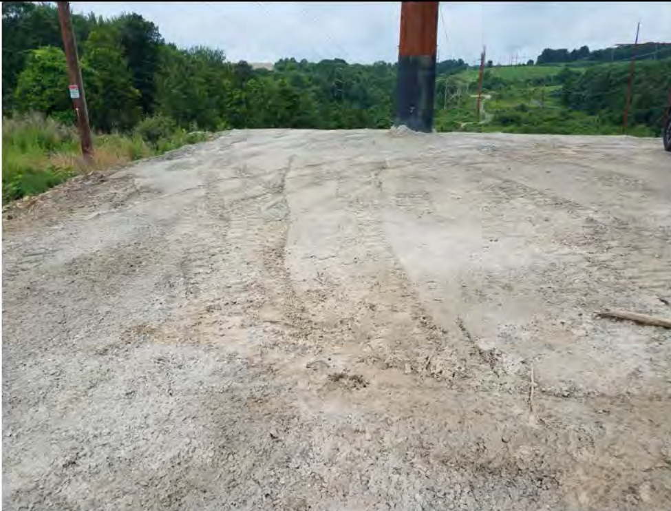
Photo 7: 07/06/2018, Watertown: Map 04, Str08, fine sediments continue to wash out of exposed, unstabilized/unvegetated soils during rain events. Photo taken facing west.
