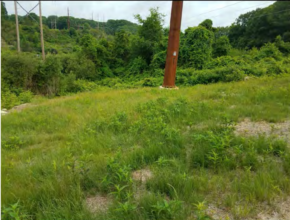
Photo 11: 07/06/2018, Watertown: Map 09, Str23 pad stabilization. Photo taken facing north.
