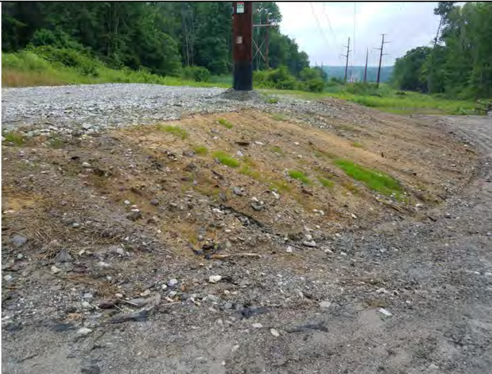
Photo 16: 07/06/2018, Litchfield: Map 29, Str83 Pad and upland slope erosion, no stabilization. Photo taken facing north.
