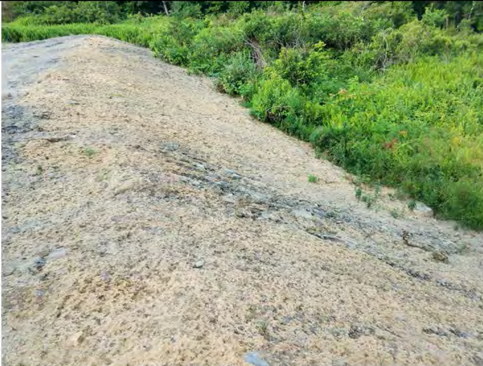
Photo 6: 07/06/2018, Watertown: Map 03, Str07 slope erosion, hydro seed application last fall, no visible growth. Photo taken facing east off of the south slope of pad.
