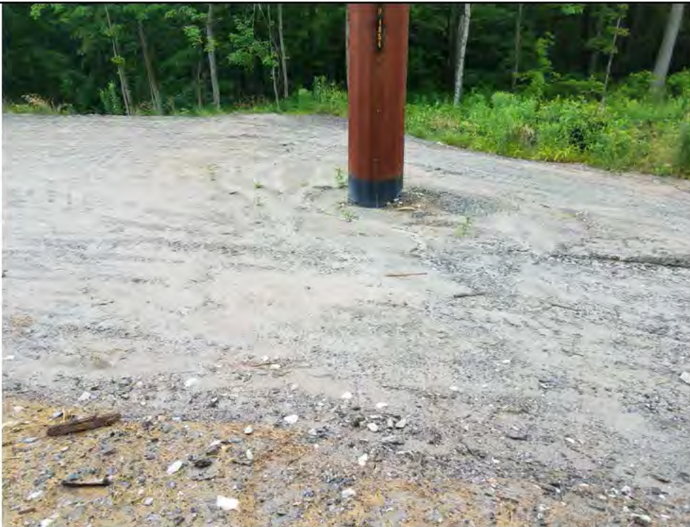
Photo 18: 07/06/2018, Litchfield: Map 29, Str83, fine sediments continue to wash out of exposed, unstabilized/unvegetated soils during rain events. Photo taken facing east.
