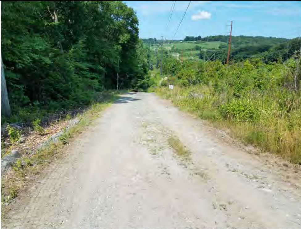
Photo 30: 07/13/2018, Watertown: Map 03, access road between Str07 and Str08, water bars and sediment basin will be installed to help control surface water flow. Photo taken facing north, from Str7 towards Str8.
