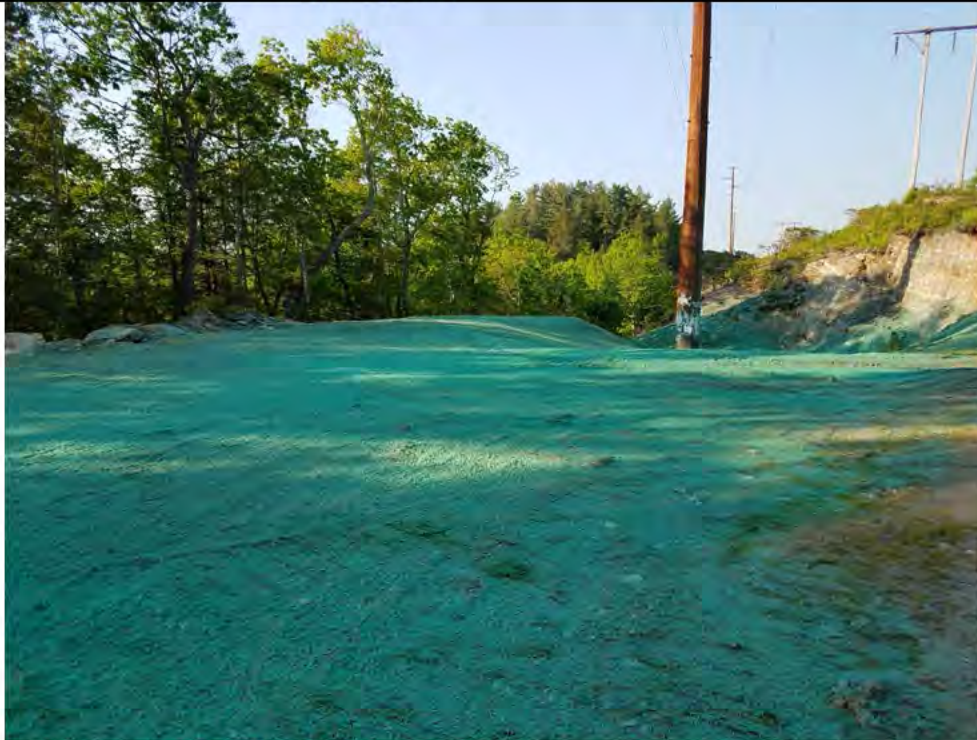
Photo 4: 05/25/2018, Watertown: Map 15, Str42, pad stabilization measures (graded and hydro seeded). Photo taken facing south along the access road and work pad, Str42 in the distance.
