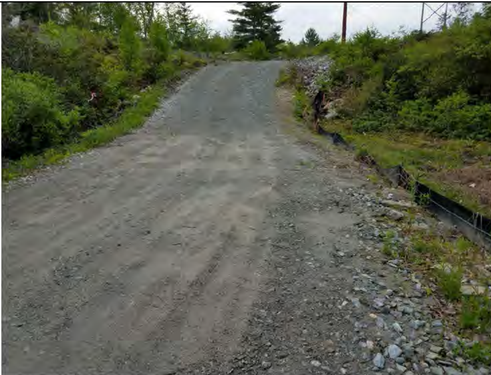
Photo 10: 05/18/2018, Watertown: Map 13, access road south of Str36, failing silt fence abutting wetland W-C15. Photo taken facing north along the access road toward Str36.
