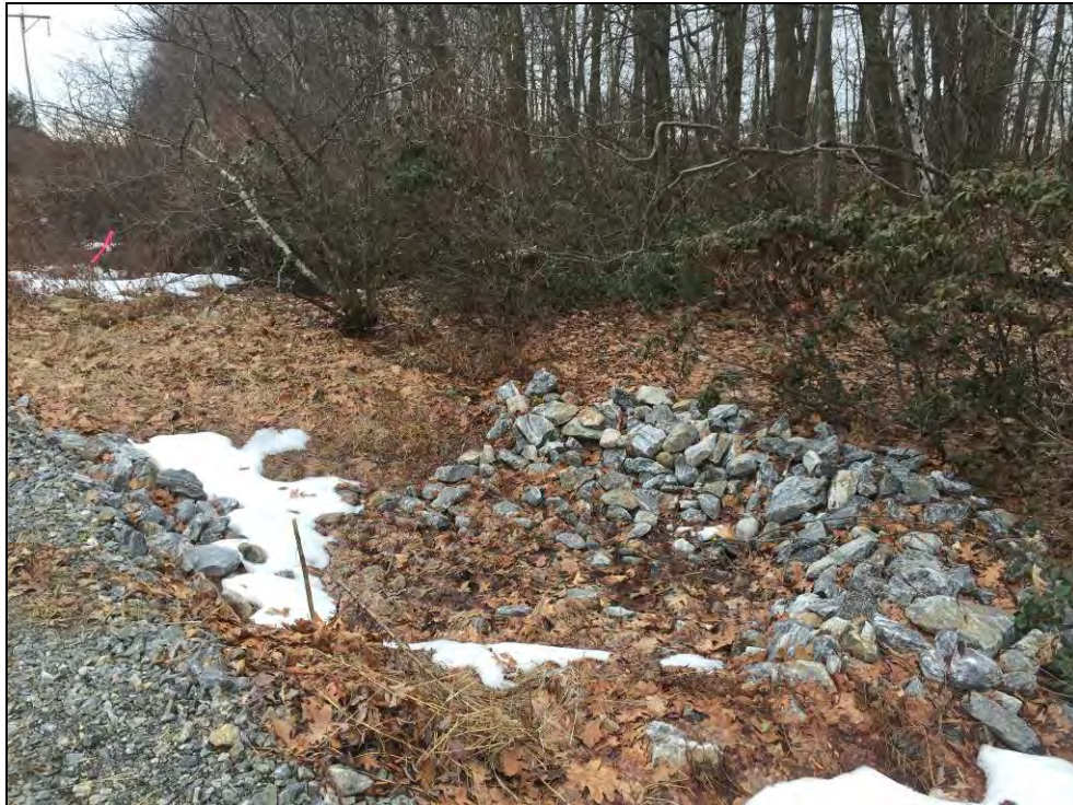
View of Wetland C16 and riprap swale. View facing southwest.
