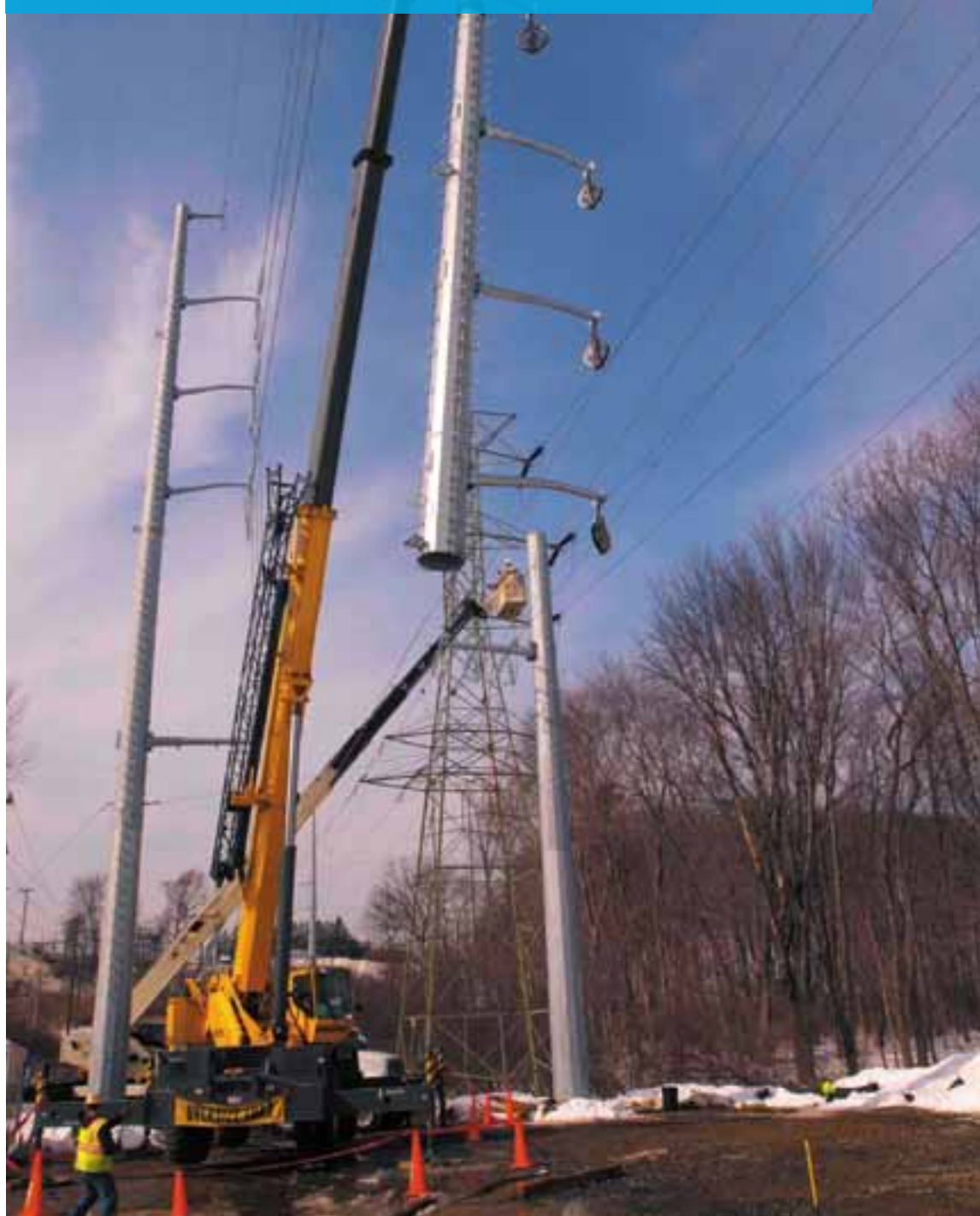
4. New Structure Installation
