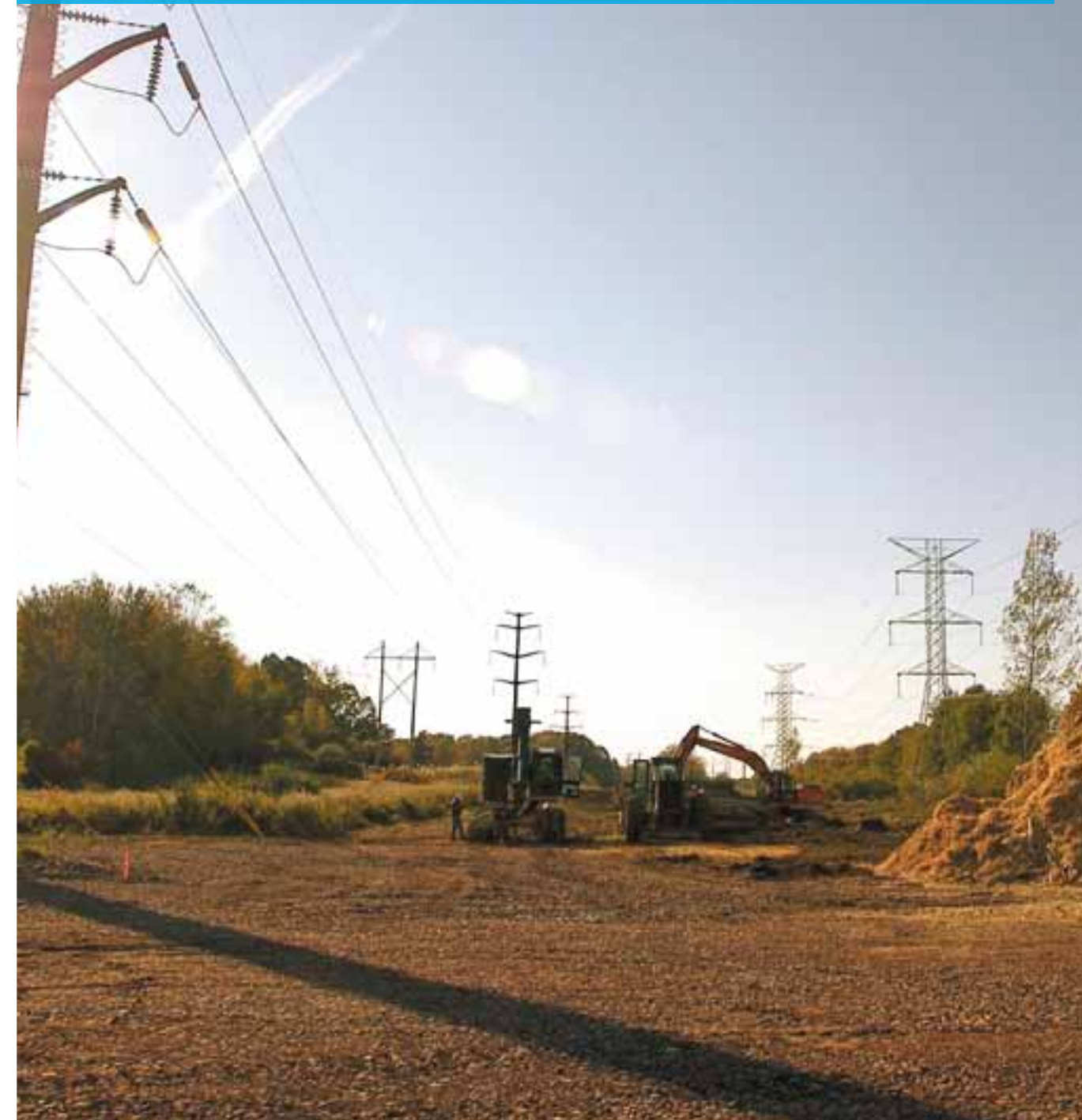
2. Work Area Prep
