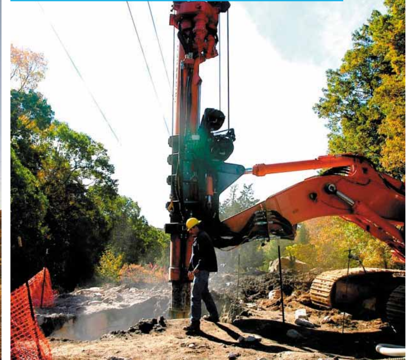
3. Structure Foundation Installation
