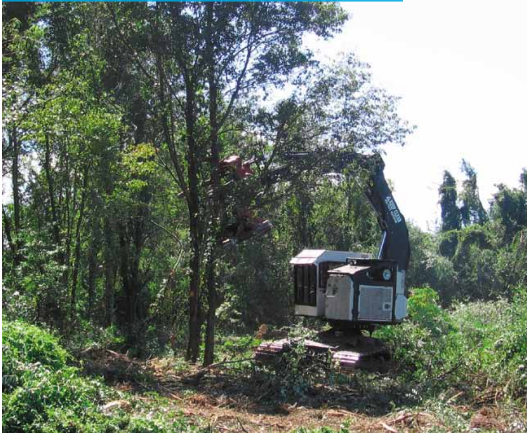
1. Right Of Way Clearing
