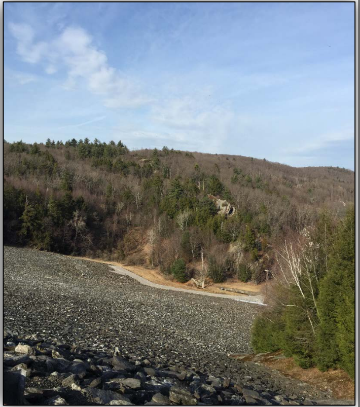
Photo 14: Black Rock Lake Dam, Watertown/Thomaston. View from dam overlook to northeast toward view of ROW traversing hillside north of State Route 109.
