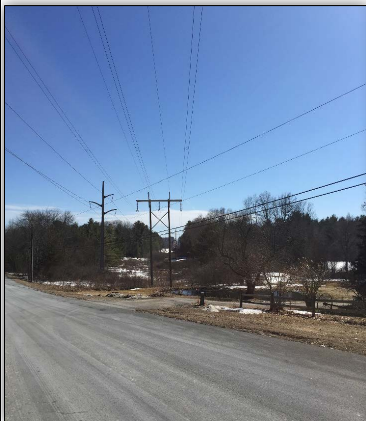
Photo 11: Wildcat Hill Road, Harwinton. View to south along ROW.
