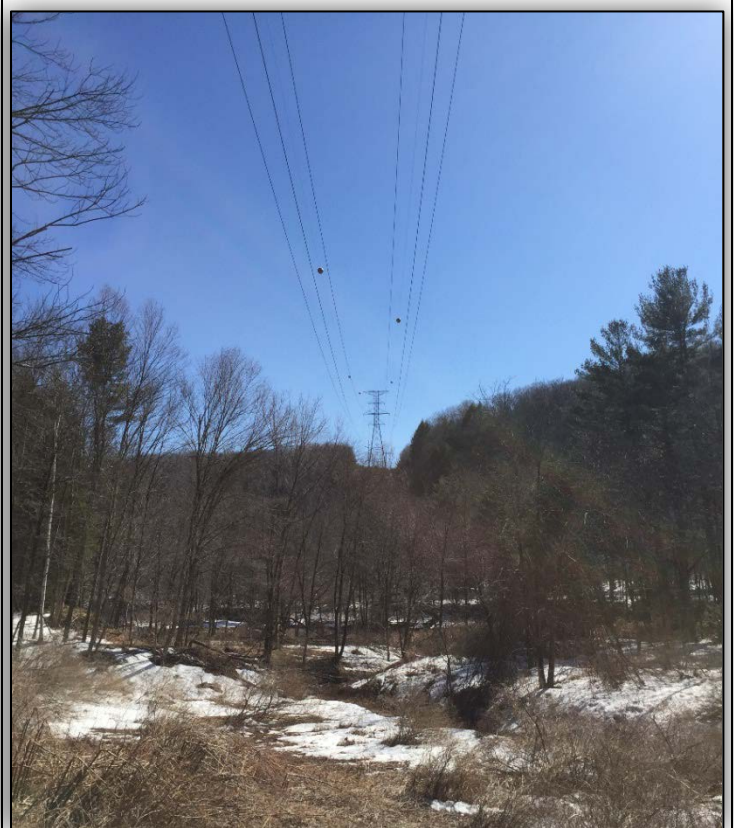
Photo 20: Valley Road, Harwinton. View to southwest of existing transmission line ROW, looking across Naugatuck River toward State Route 8.
