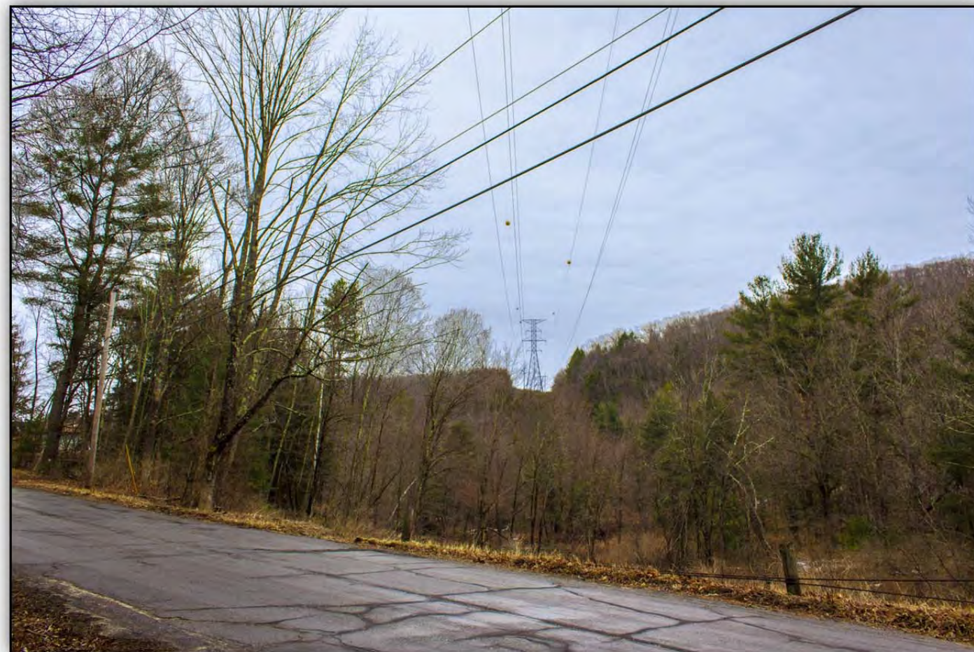
(Existing Transmission Right-of-Way – Leaf-off Condition)
