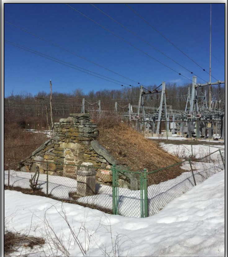
Photo 24: Campville Substation, Harwinton. Grave marker (and burial site) fenced off in front of substation entrance.
