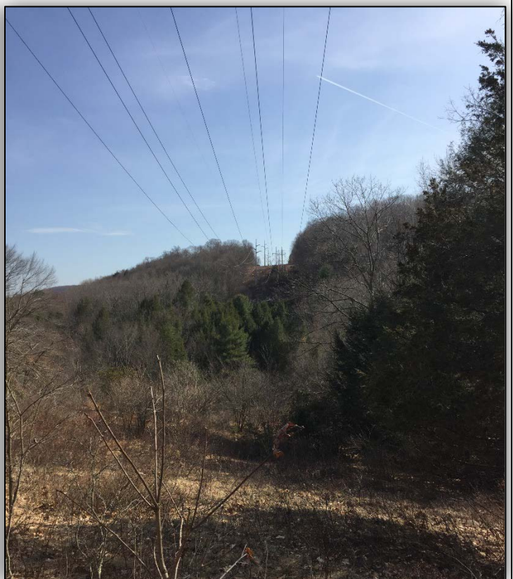
Photo 16: Northfield Brook Recreation Area, Thomaston. View to south (toward Walnut Hill Junction) from "Yellow" hiking trail crossing of Eversource ROW.
