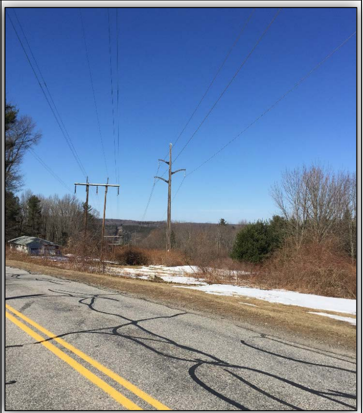
Photo 10: Campville Road, Litchfield. View to the north.
