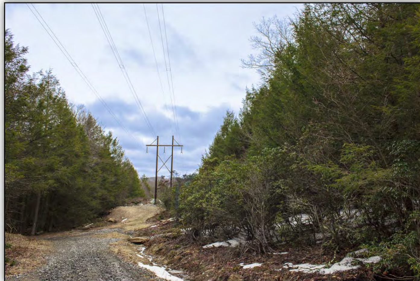
(Existing Transmission Right-of-Way – Leaf-off Condition)
