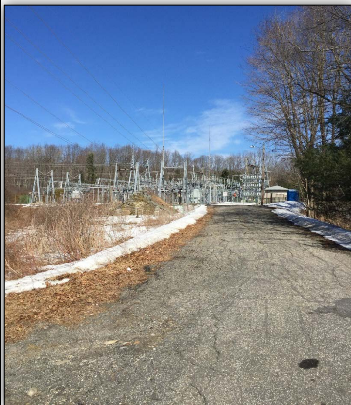
Photo 23: Campville Substation, Harwinton. View to east, substation access road entrance off Wildcat Hill Road.
