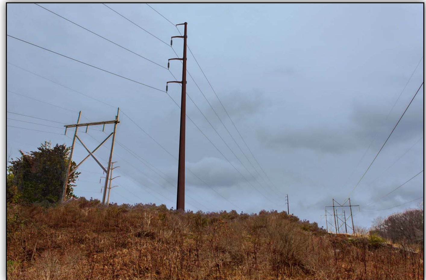
(Simulation of the Existing Transmission Right-of-Way – Leaf-off Condition)
