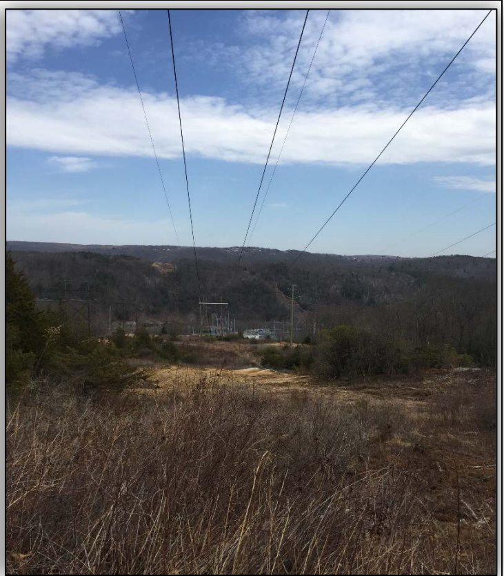
Photo 2: View of Frost Bridge Substation from Jericho Trail, Watertown. View to east along ROW from Trail crossing.
