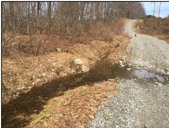
Photo 5: C4-1 is formed by the maintenance road embankment
