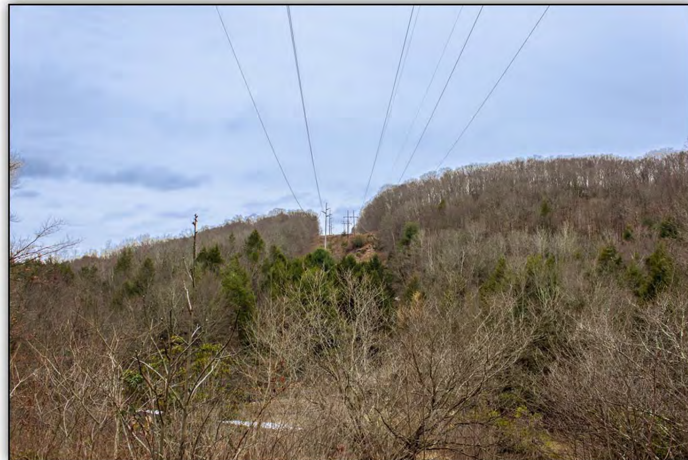
(Existing Transmission Right-of-Way – Leaf-off Condition)
