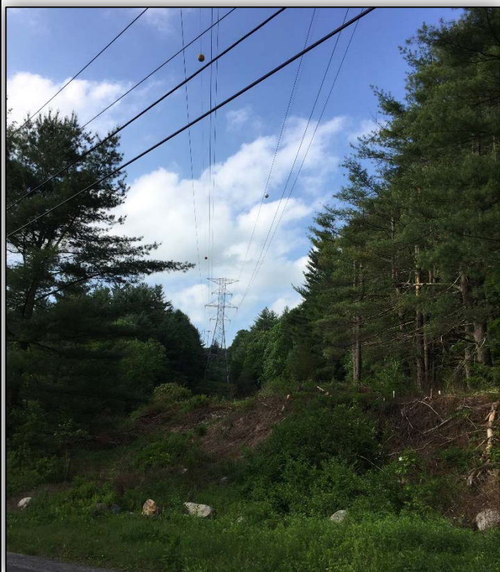
Photo 15: Valley Road, Harwinton. View to northeast of existing transmission line ROW and double-circuit steel lattice tower to be replaced.
