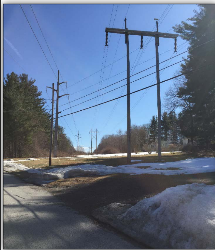
Photo 9: Campville Road, Litchfield. View to the south.
