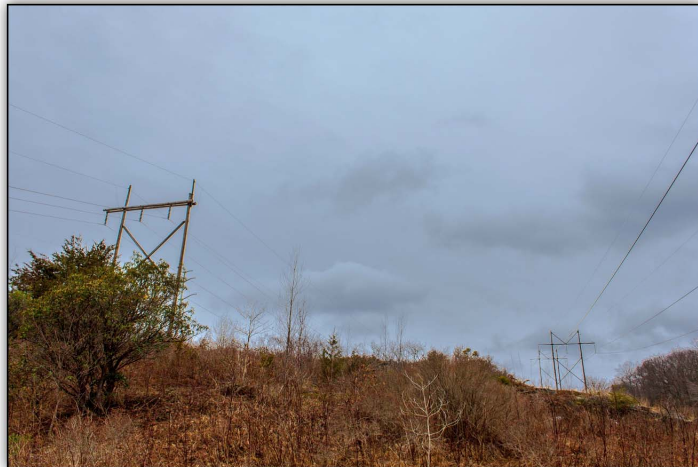
(Existing Transmission Right-of-Way – Leaf-off Condition)
