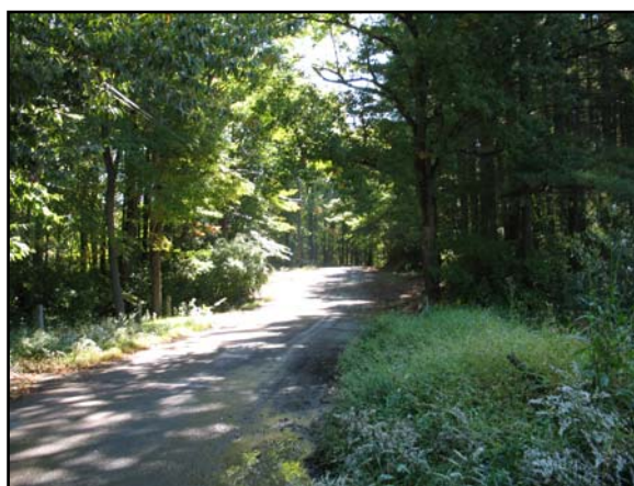
Main entrance to Roosevelt Forest along Peters Lane. The road is narrow & needs improvement.
