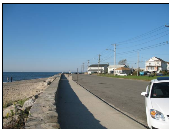
Seawall & Beach along Beach Drive
