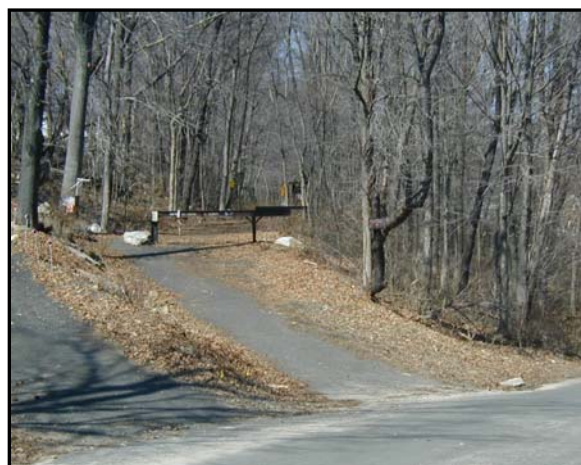
Housatonic Railroad Trail – timber bridge over Pequonnock River in Monroe (upper); start of Pequonnock Valley in Trumbull (lower).
