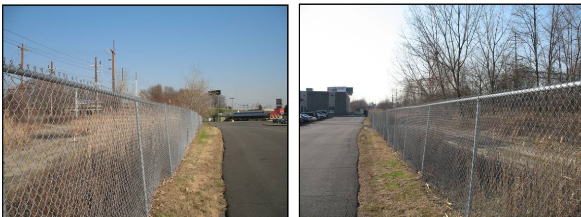
Parking lot of Stratford Square shopping center along New Haven rail line.
