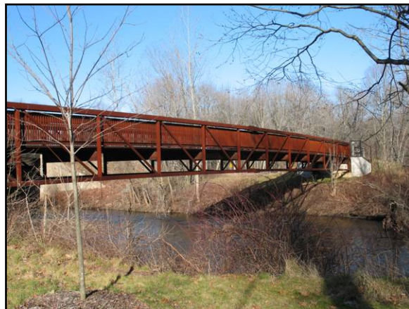
Illustrative bridge that would be built over the mouth of Marine Basin
