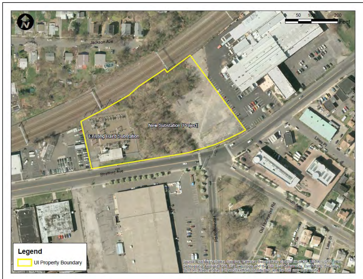
Figure 1-1 Aerial view of the existing substation and Project
