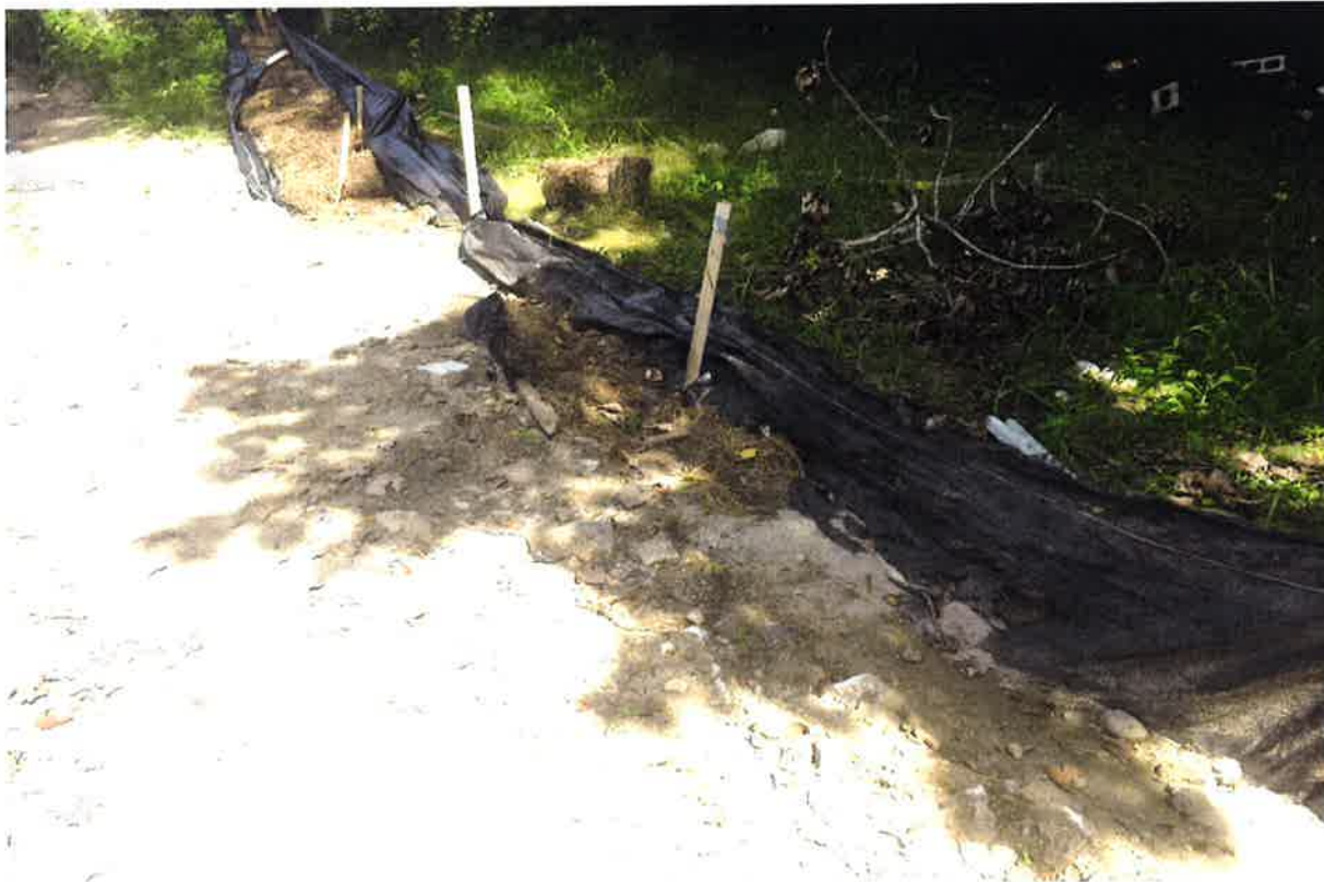
Photo 4: View of CA #5, repair perimeter controls, looking west.
