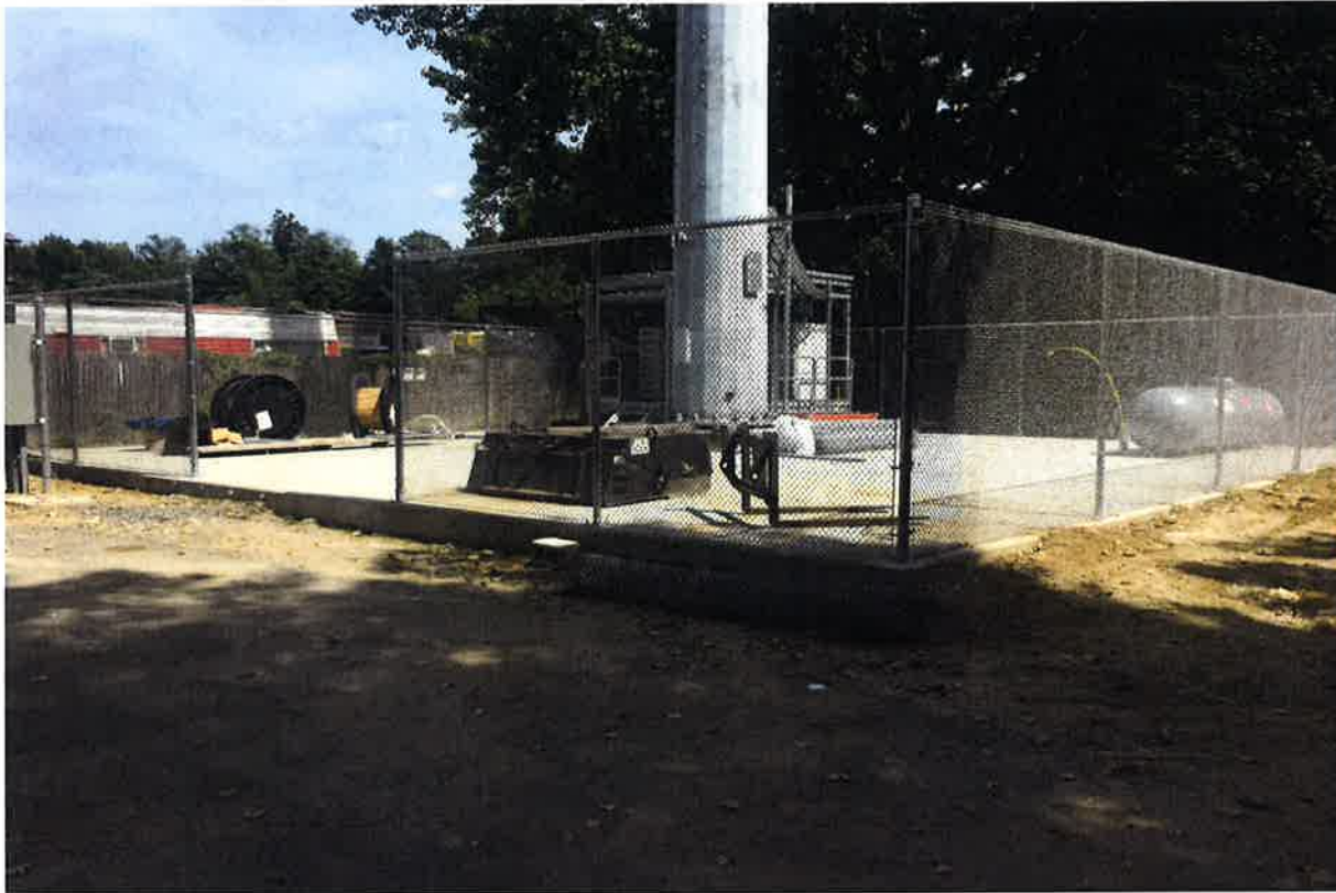
Photo 1: View of compound area looking south.
