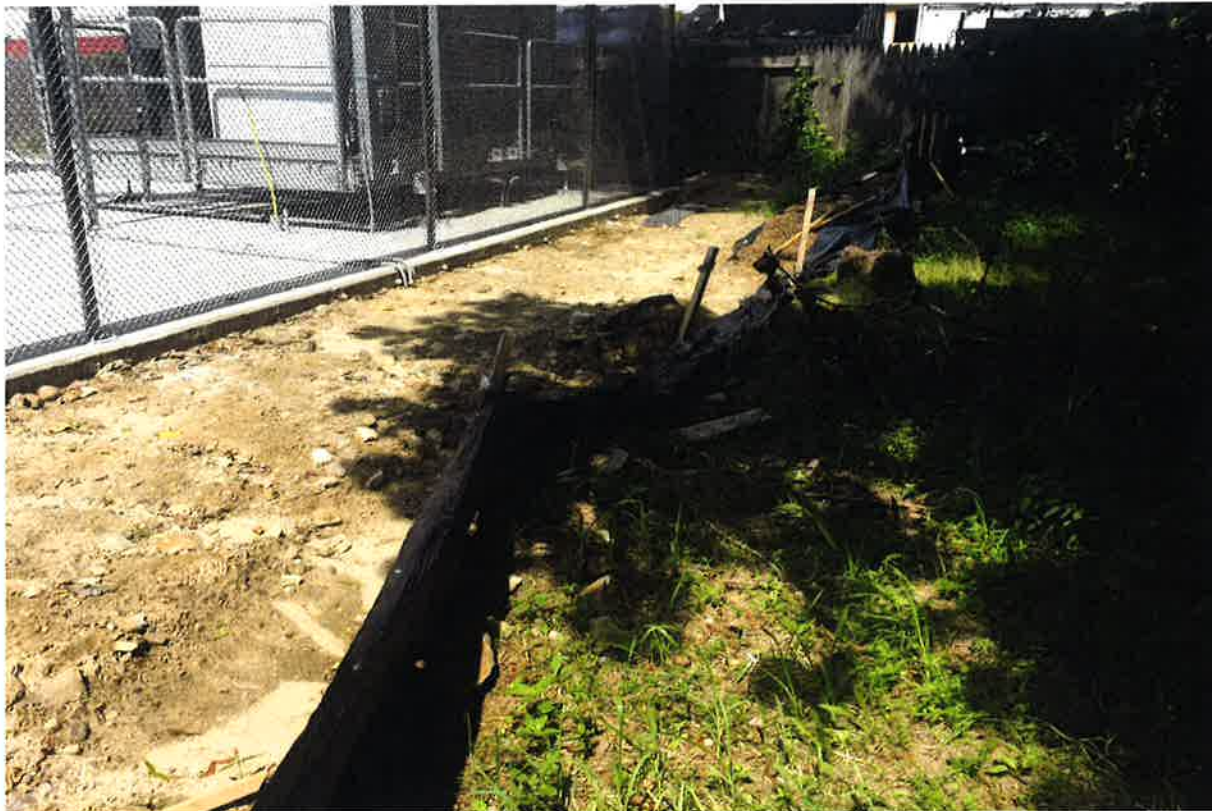
Photo 5: View of CA #5, repair perimeter controls, looking west.
