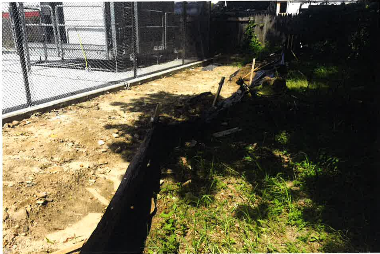
Photo 3: View of CA #5, repair perimeter controls, looking west.
