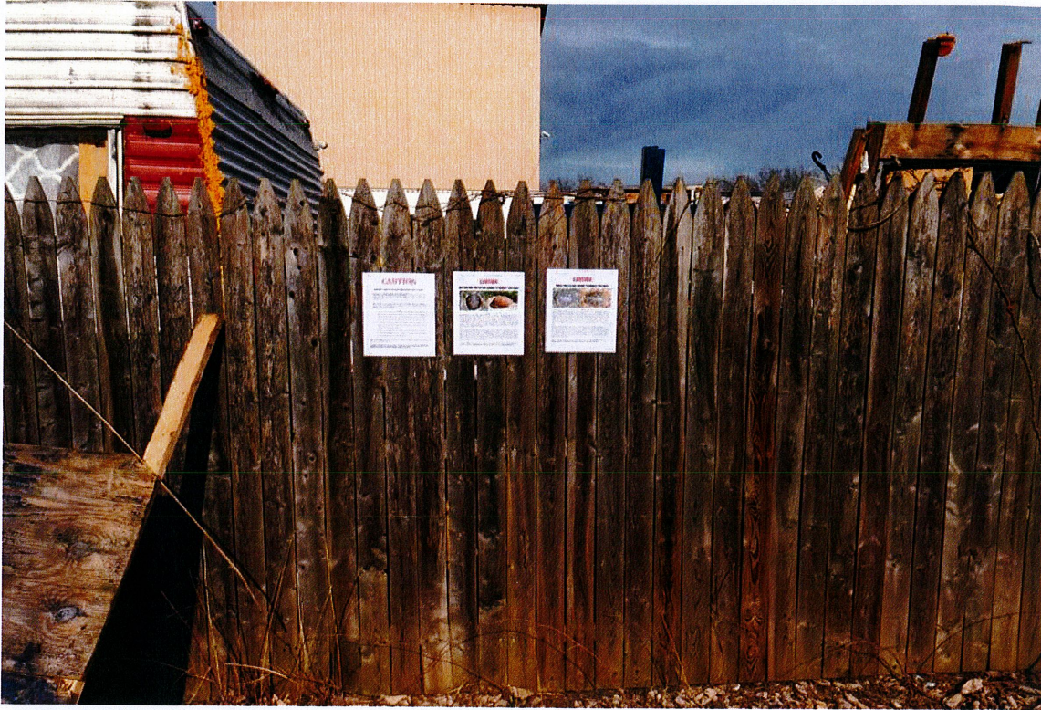
Photo 9: View of rare turtle and wetland protection signs installed at site, looking north. Photo taken April 3, 2017.
