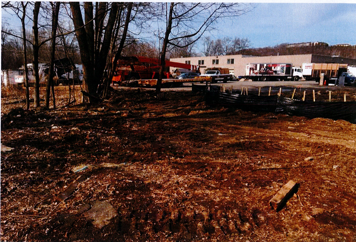
Photo 4: View of CA #3 - seed and mulch exposed soils outside of erosion controls, looking north.
