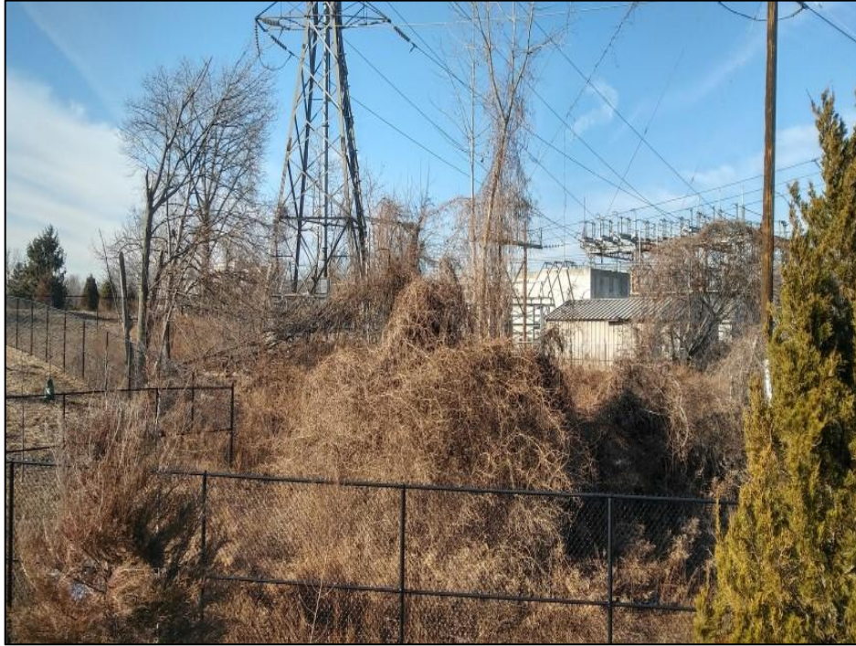
Photo 15. Overview photo of eastern termination point of the proposed transmission line within the substation that currently exists at the former site of the Cos Cob Power Station facing northwest.
