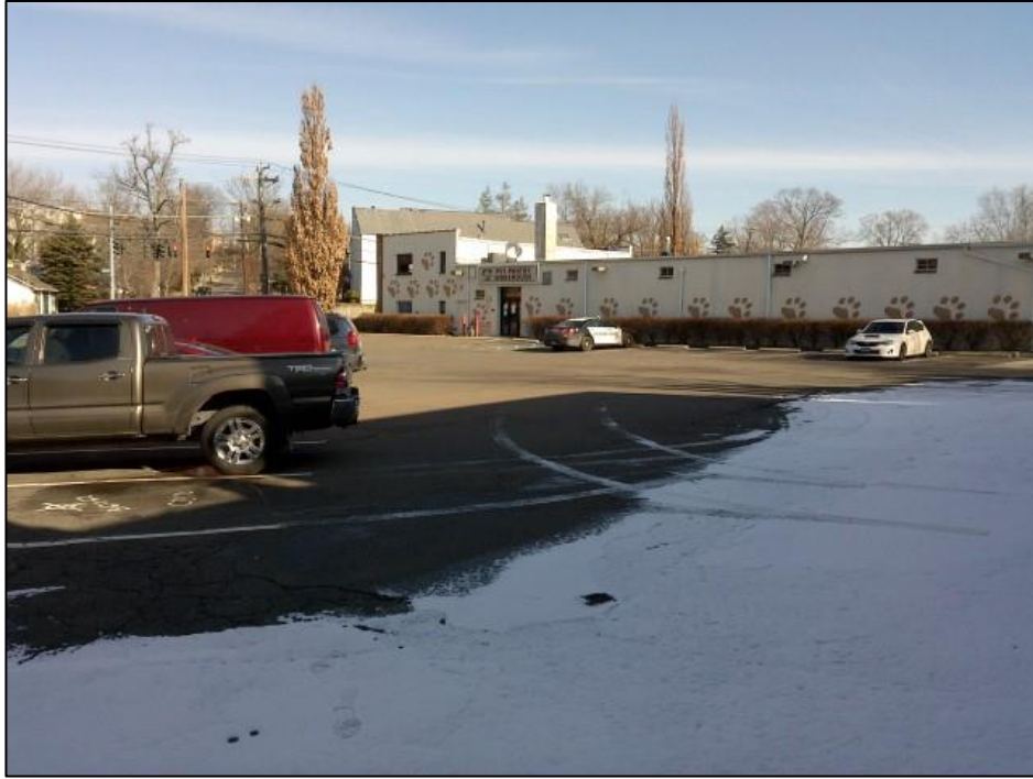
Photo 1. Overview photo from the proposed Greenwich Substation area at 290 Railroad Avenue facing northeast.
