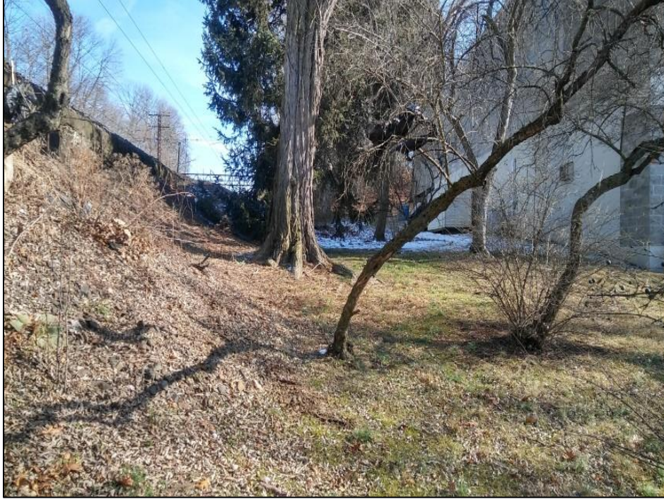
Photo 7. Overview photo of the area where the transmission line transitions from underground to overhead facing east.
