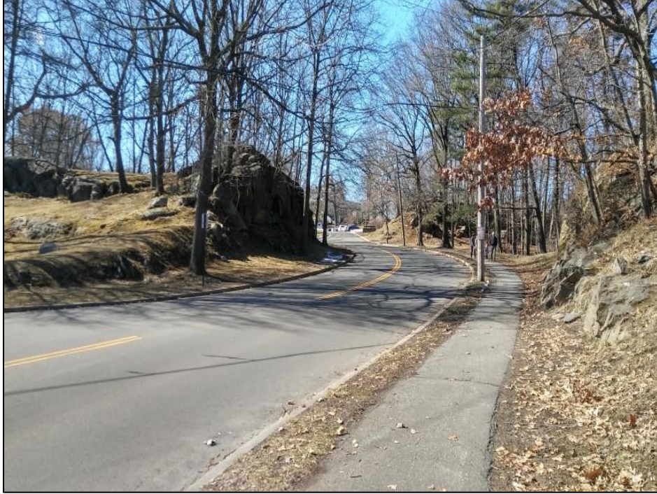
Photo 5. Overview photo of the proposed underground transmission line facing west along Museum Drive.
