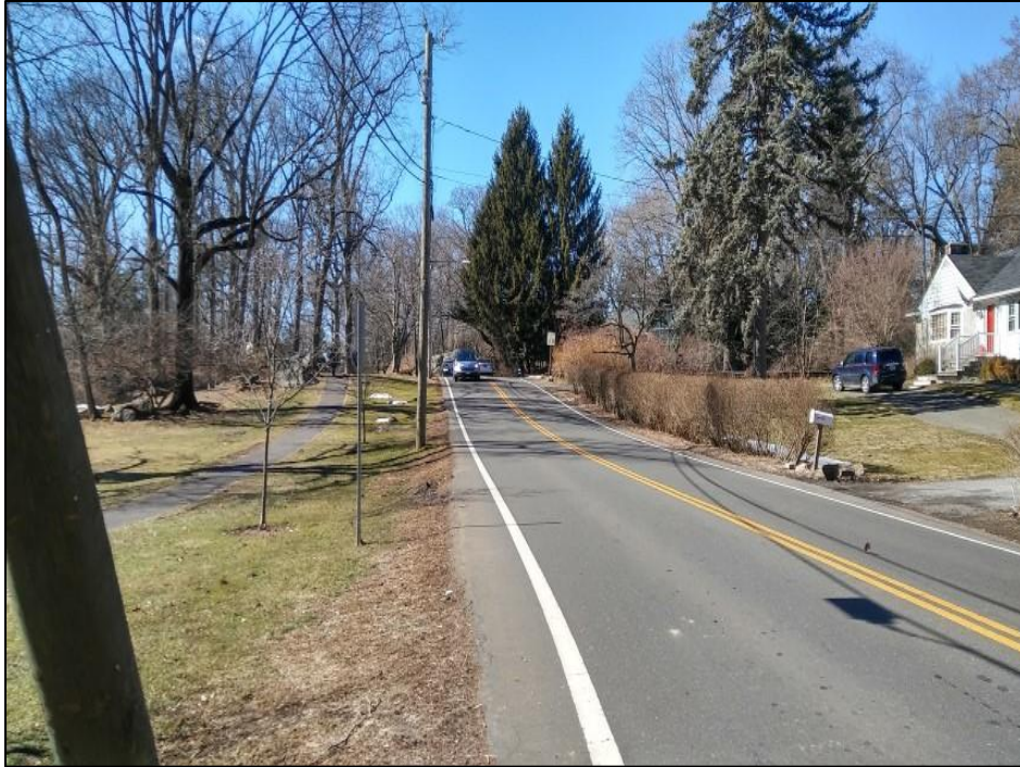
Photo 9. Overview photo of the proposed underground transmission line facing west along Bruce Park Avenue.
