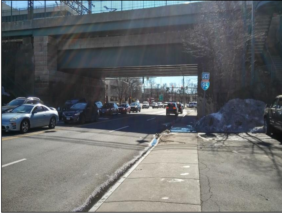
Photo 3. Overview photo of the proposed underground transmission line facing south along Arch Street.
