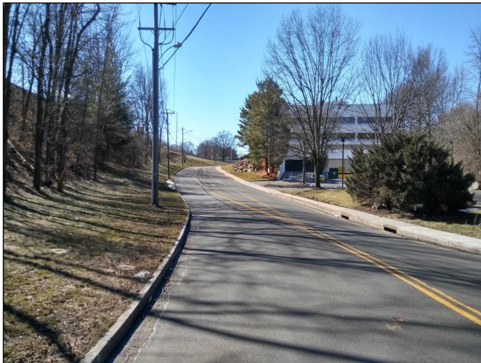
Photo 12. Overview photo of the proposed underground transmission line facing west along Sound Shore Drive from Sachem Road.
