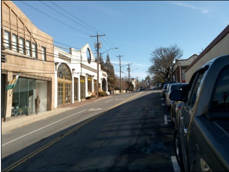
Photo 3. Overview photo of the underground portion of the proposed transmission line facing east along Railroad Avenue.
