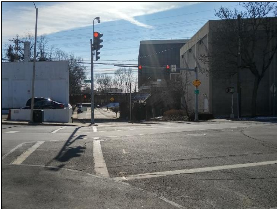
Photo 6. Overview photo towards the underground portion of the proposed transmission line facing south away from the Greenwich Avenue Historic District.
