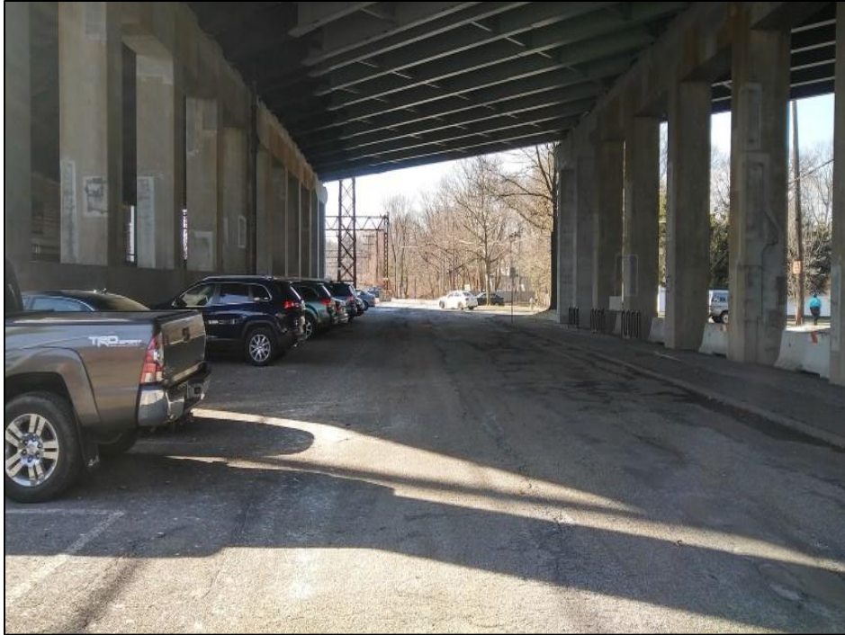
Photo 11. Overview photo of the work area to the west of the Cos Cob Train Station facing west.
