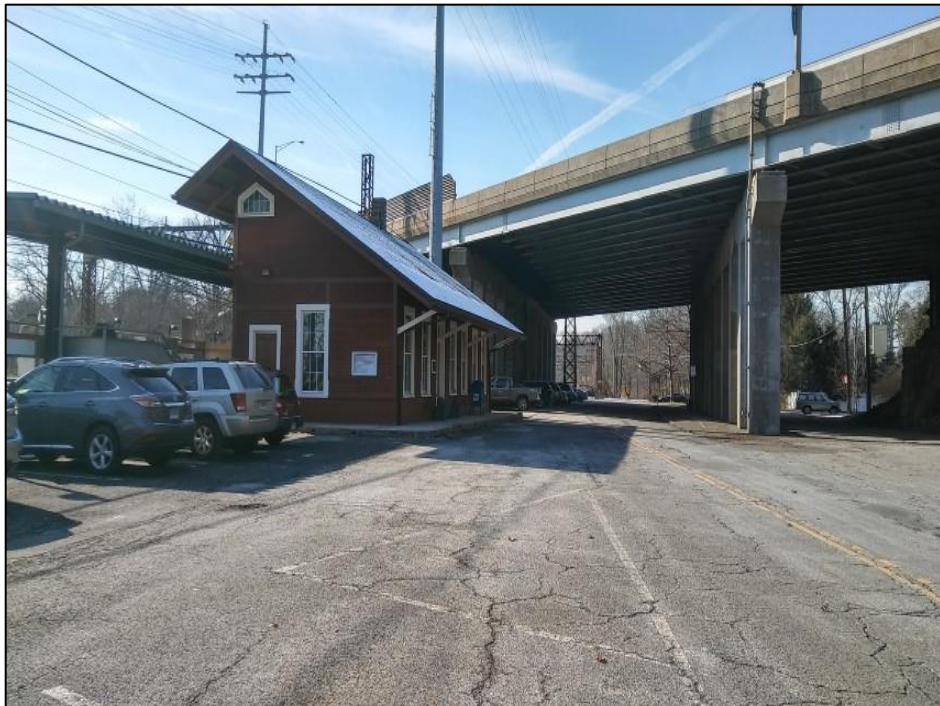
Photo 12. Overview photo of the project area, including the Cos Cob Train Station facing west.
