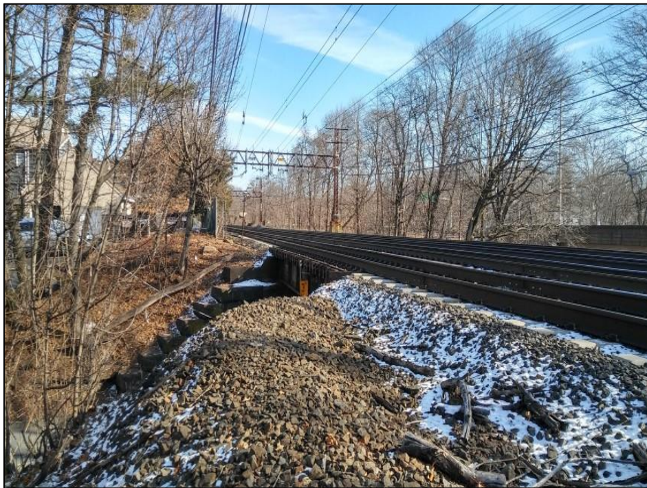
Photo 8. Overview photo of the central portion of the overhead transmission line facing east.
