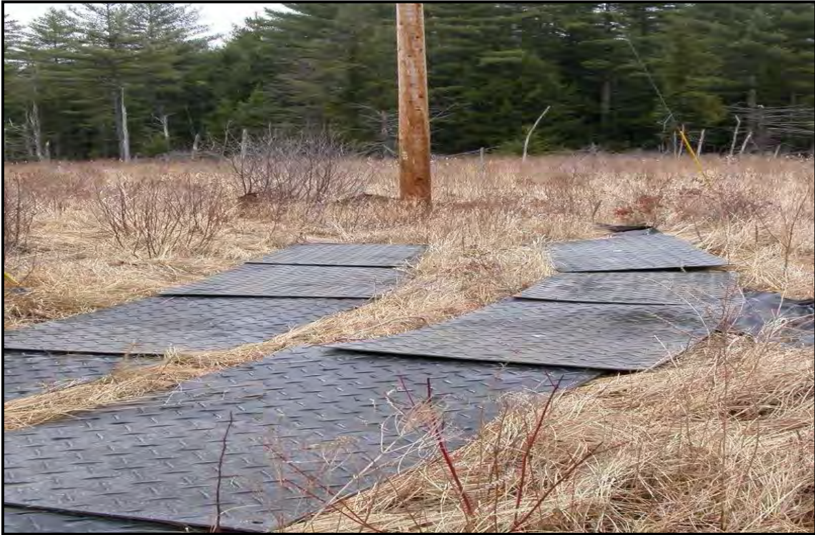
AlturnaMAT® tracks to utility pole in wetland.
