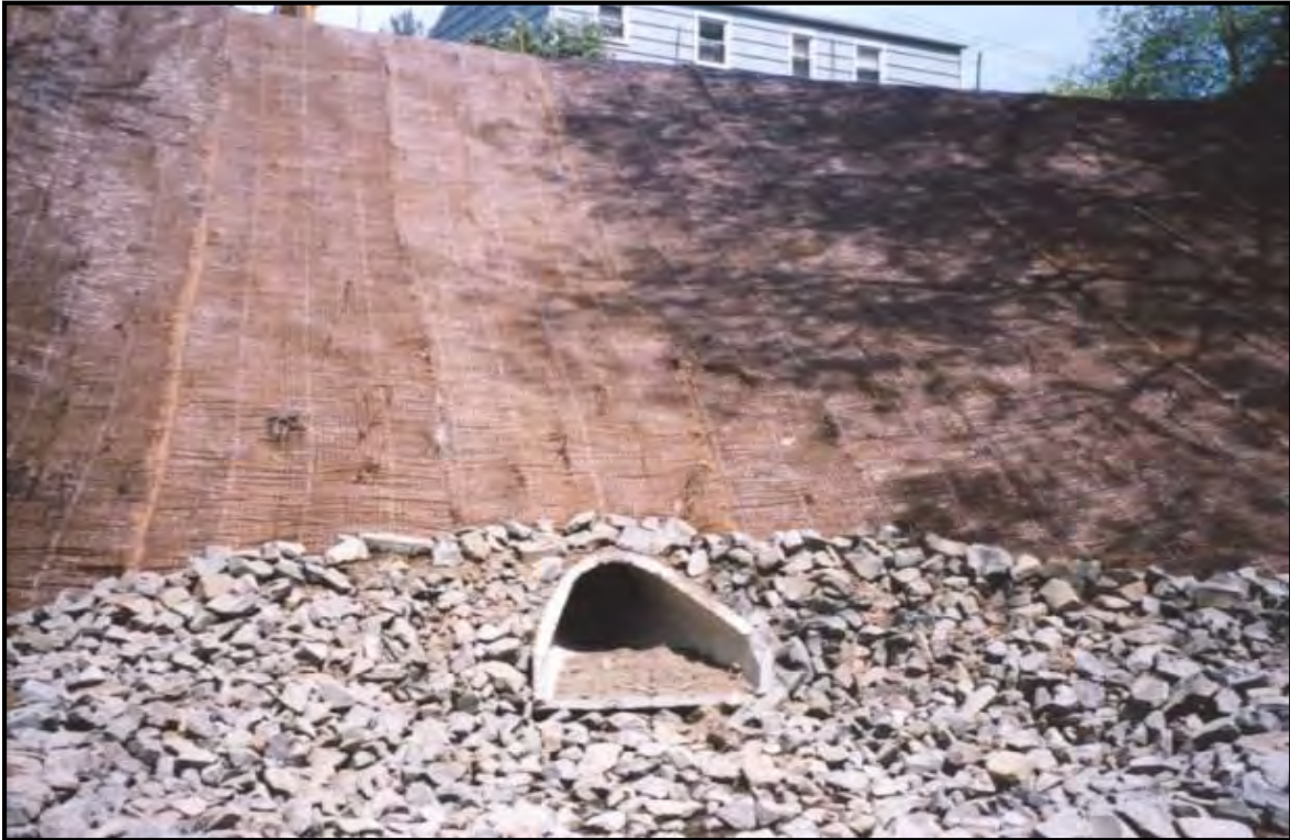
Pipe arch culvert.
