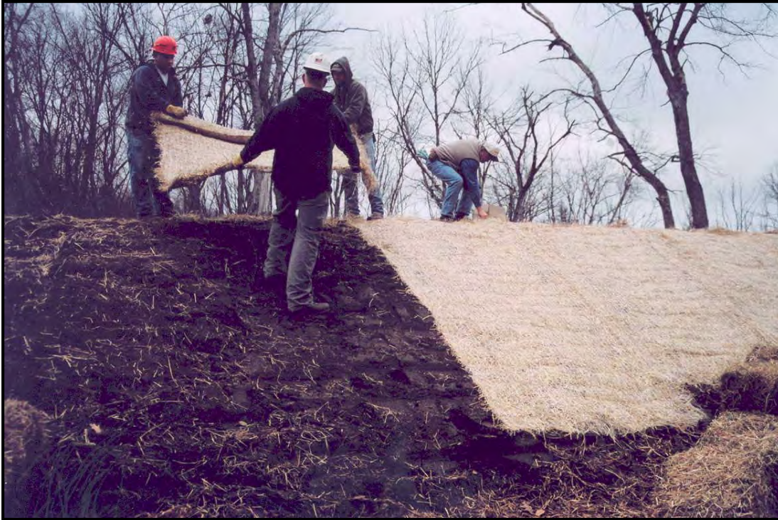
Installing erosion control blanket on an unstable slope.
