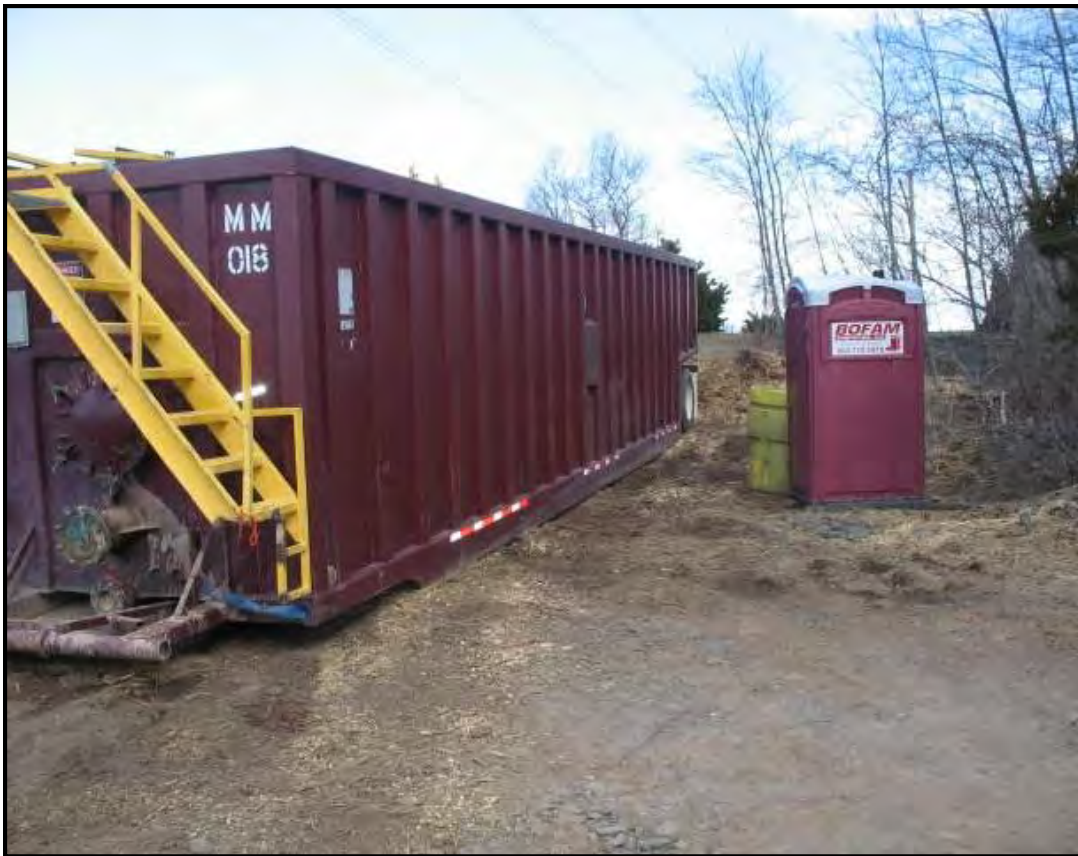
Frac tank on-site for dewatering activities.
