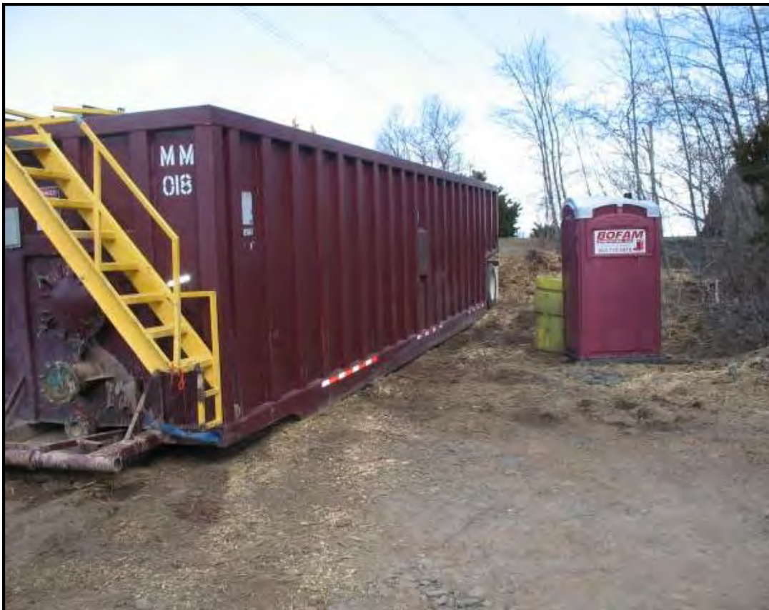
Frac tank on-site for dewatering activities.
