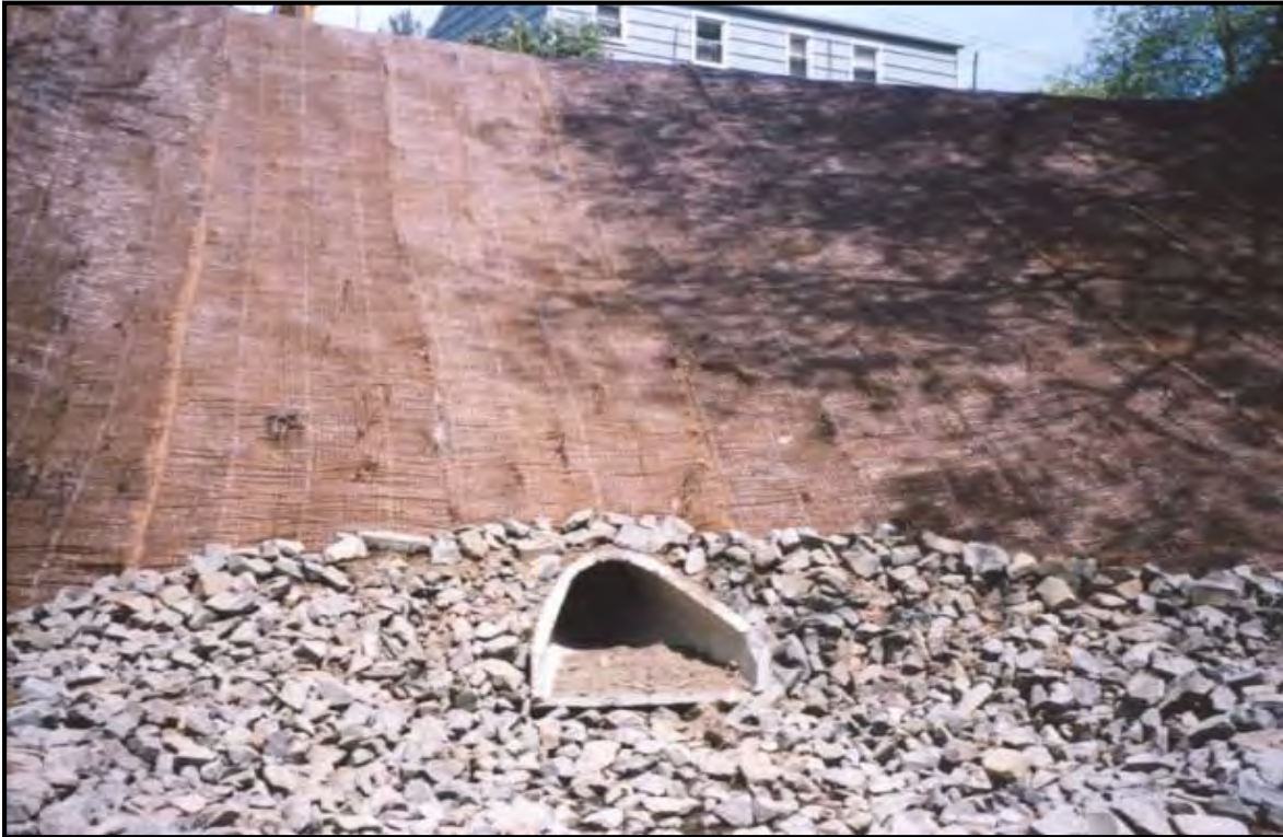
Pipe arch culvert.
