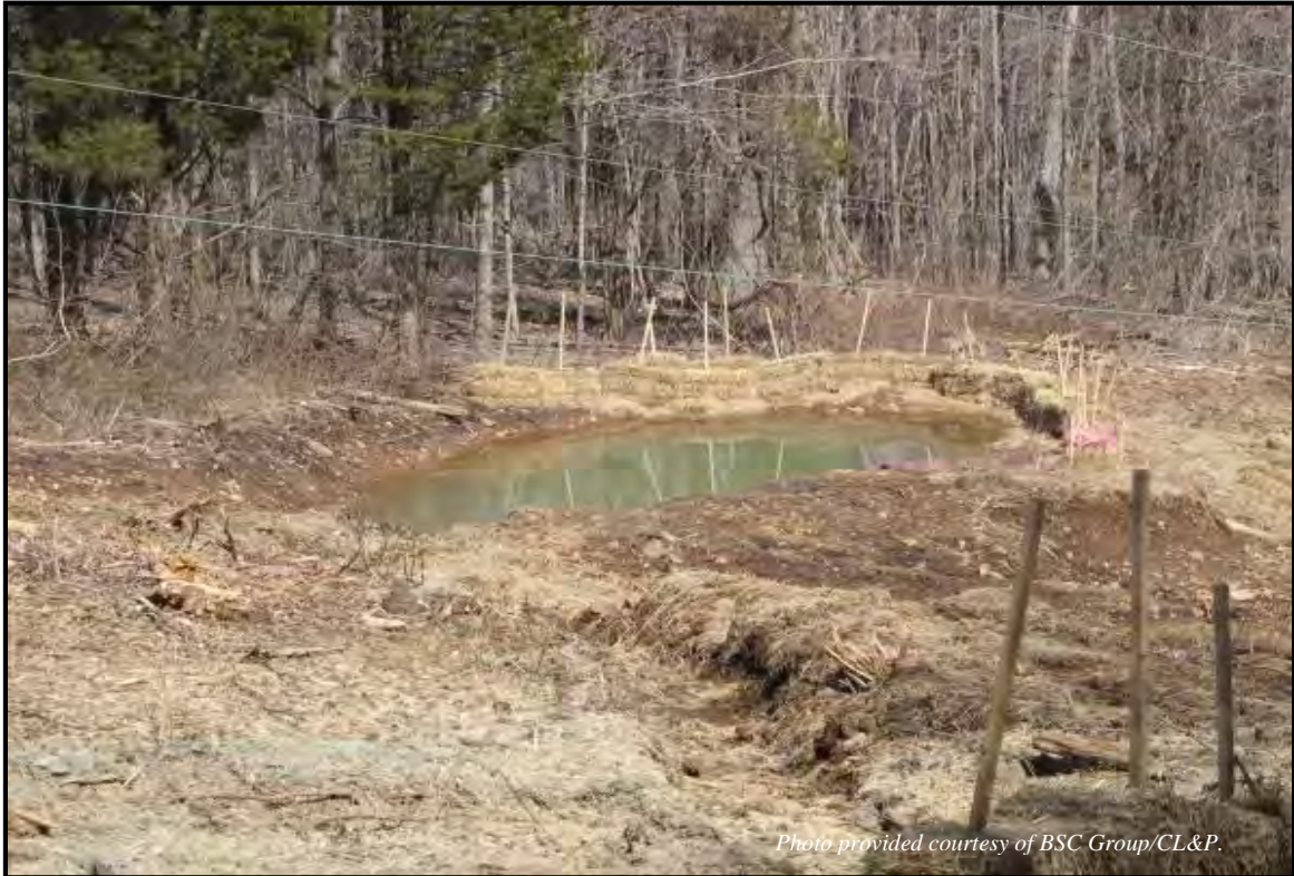
Sedimentation basin with hay bale filters.
