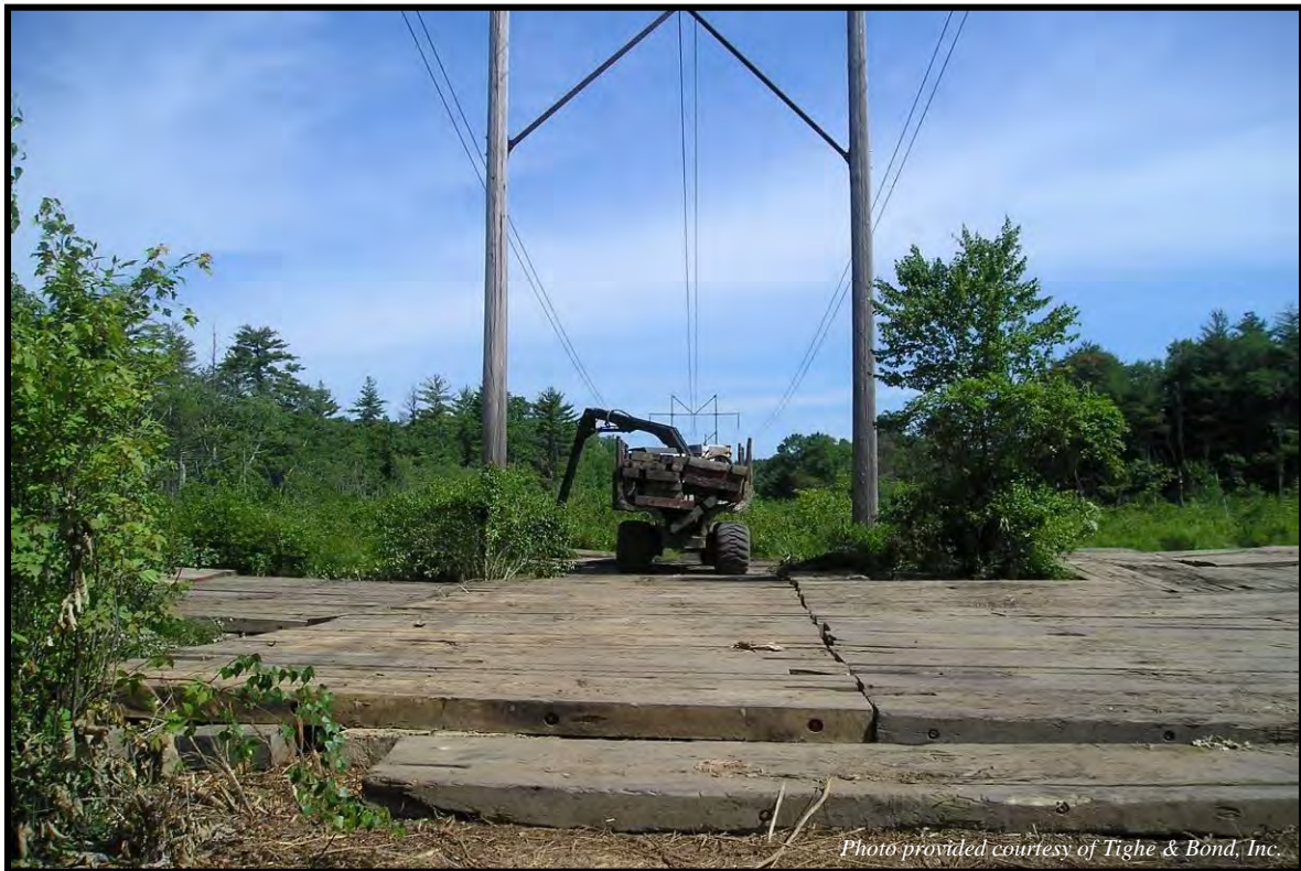
Construction mat wetland workpad for live line work.
