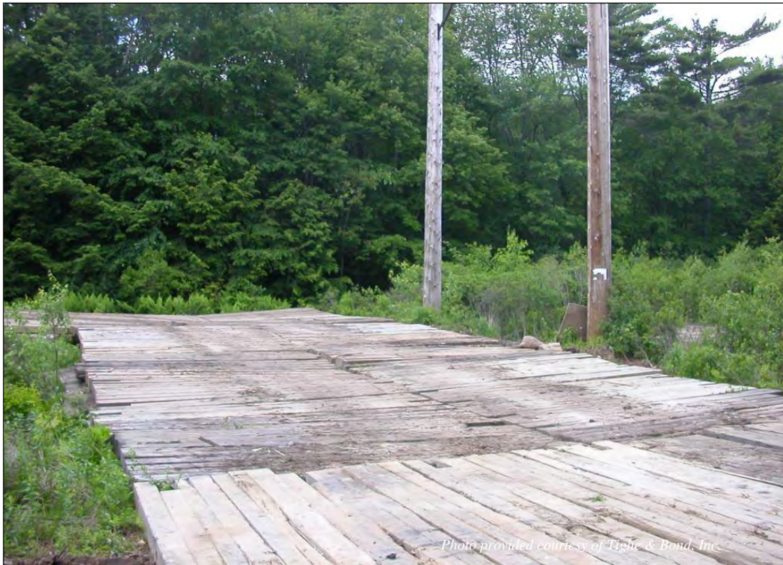
Construction mat wetland work-pad for de-energized work.
