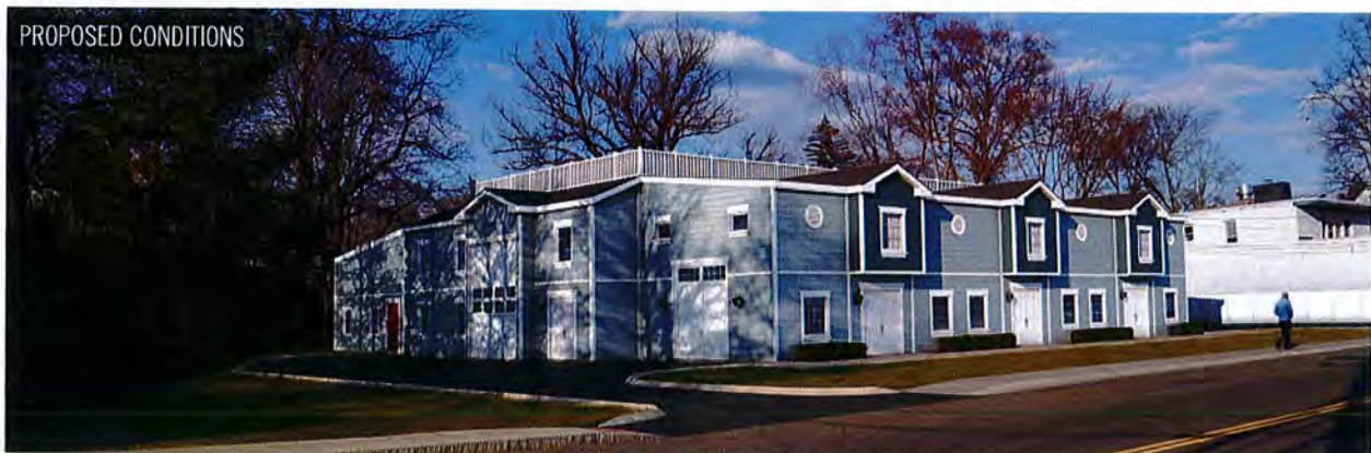
View north from Railroad Avenue.
