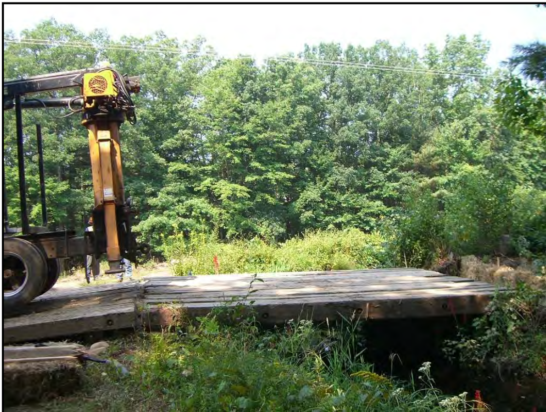
Construction mat bridge.
