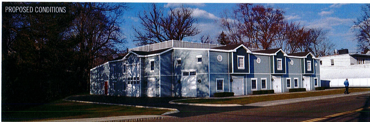
View north from Railroad Avenue.
