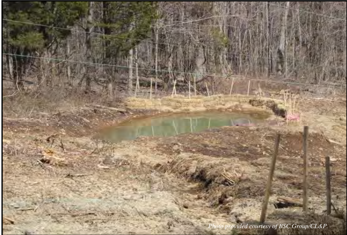
Sedimentation basin with hay bale filters.
