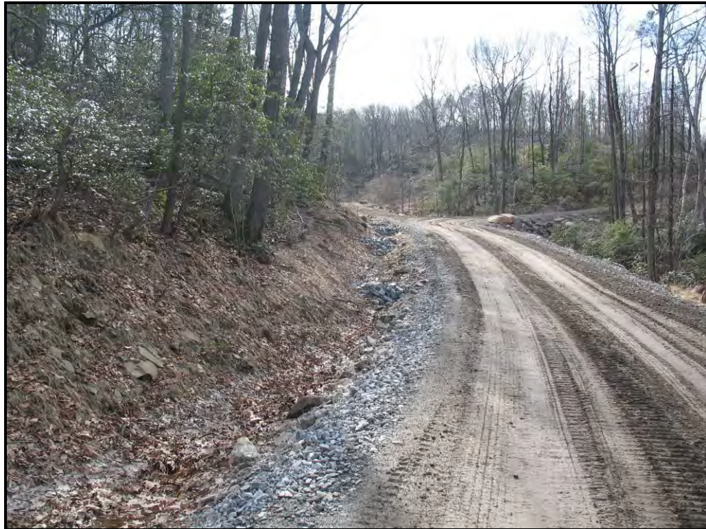
Stone check dams at construction site.
