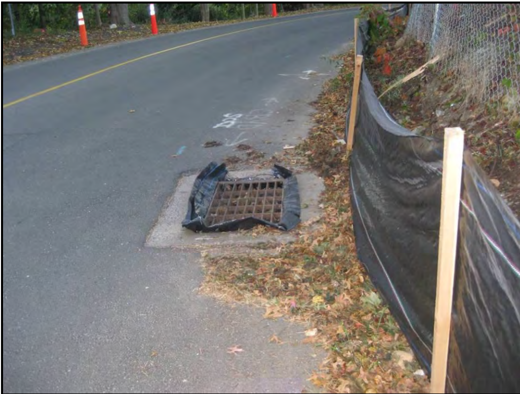
Catchbasin protected from sedimentation by filter fabric.
