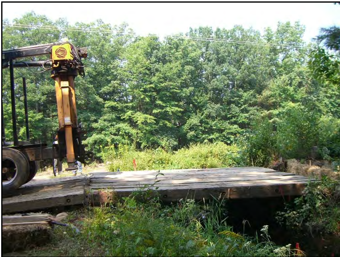
Construction mat bridge.
