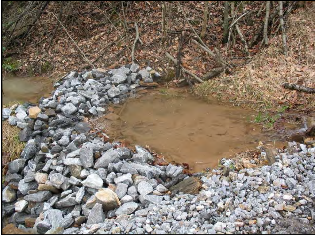
Stone check dam at construction site.
