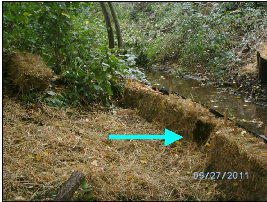
Properly installed hay bale barrier with silt fence.
