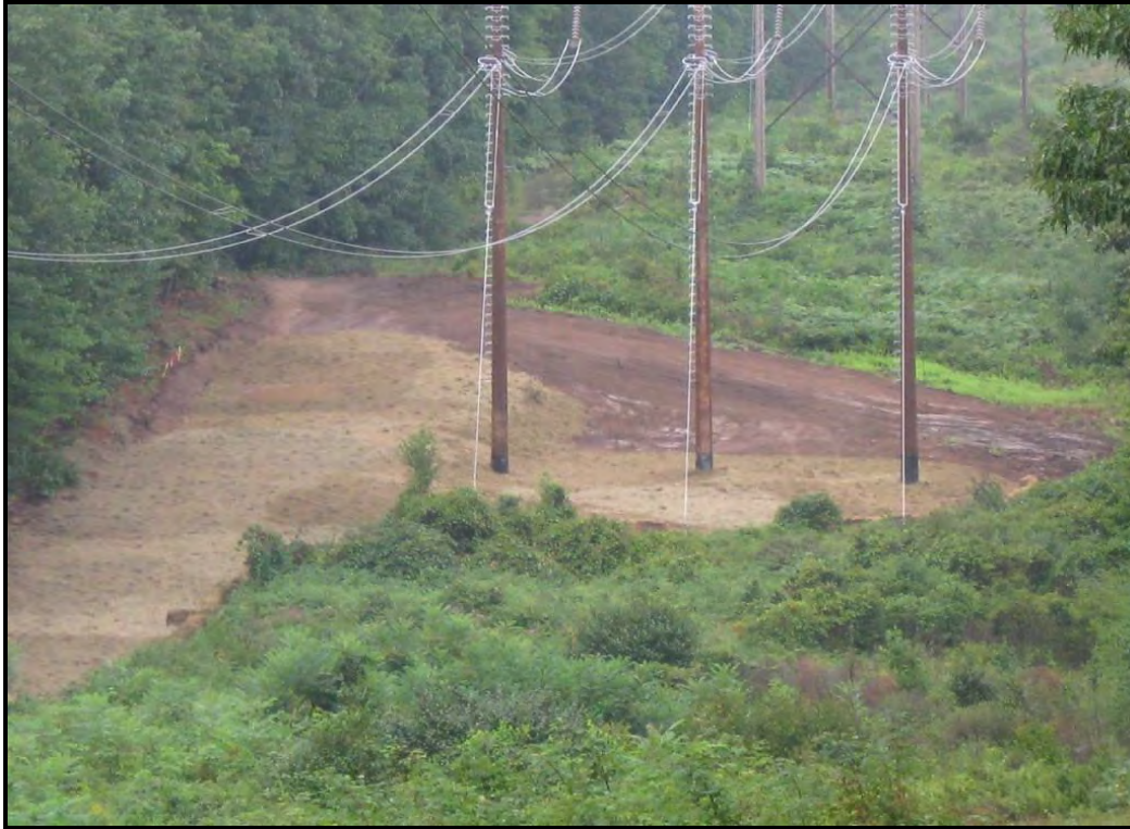
Loaming and seeding of recently disturbed right of way.
