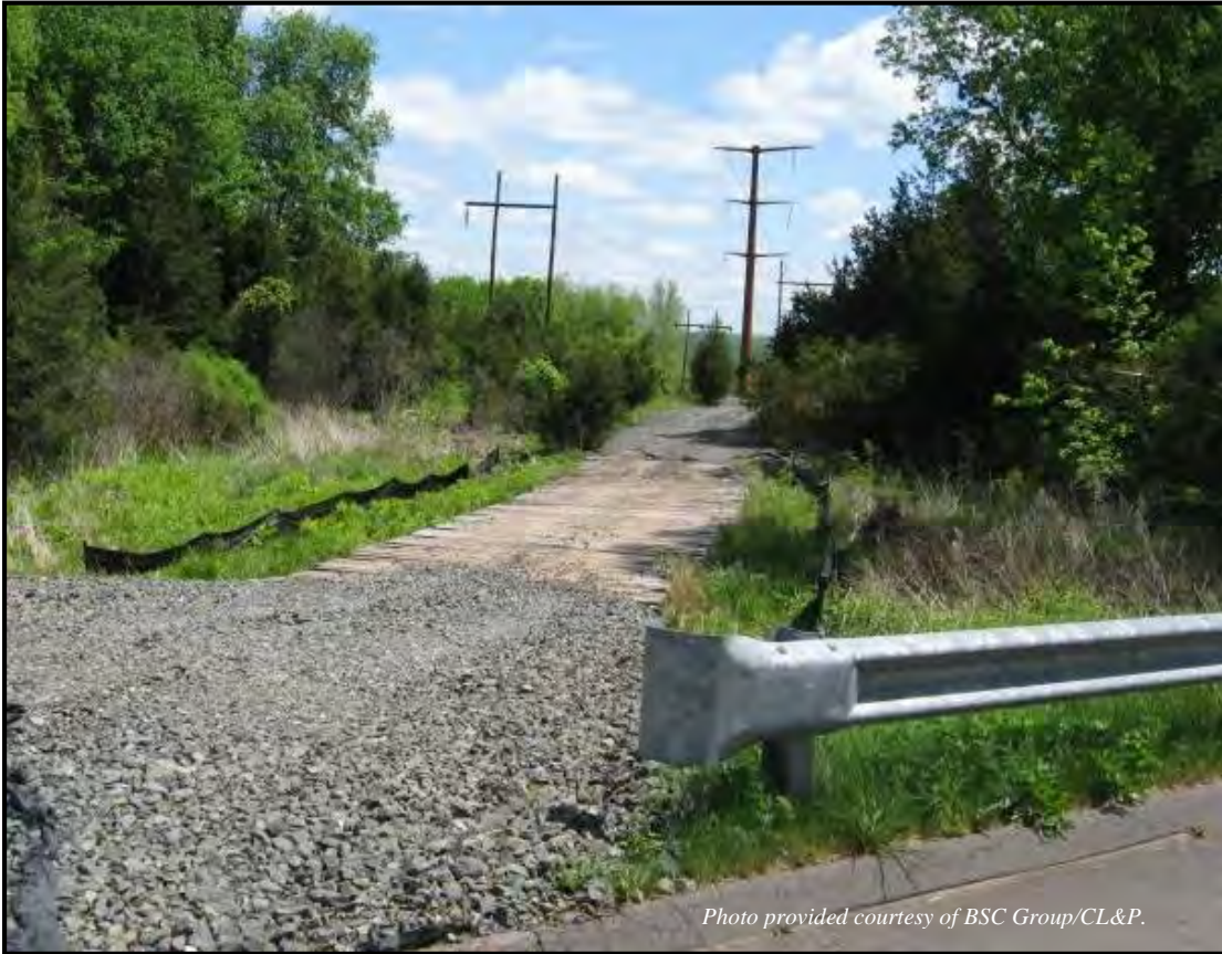
Construction entrance track pad.
