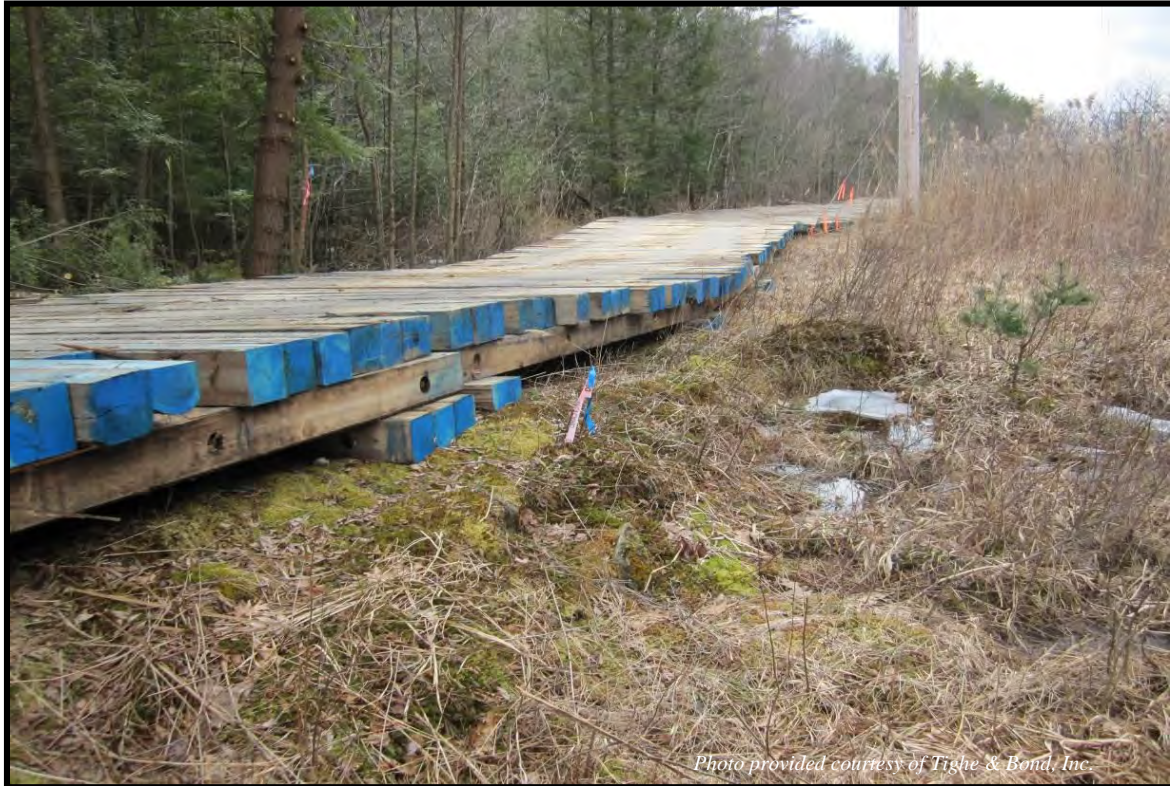
Elevated construction mat road with bridging for animal crossing.
