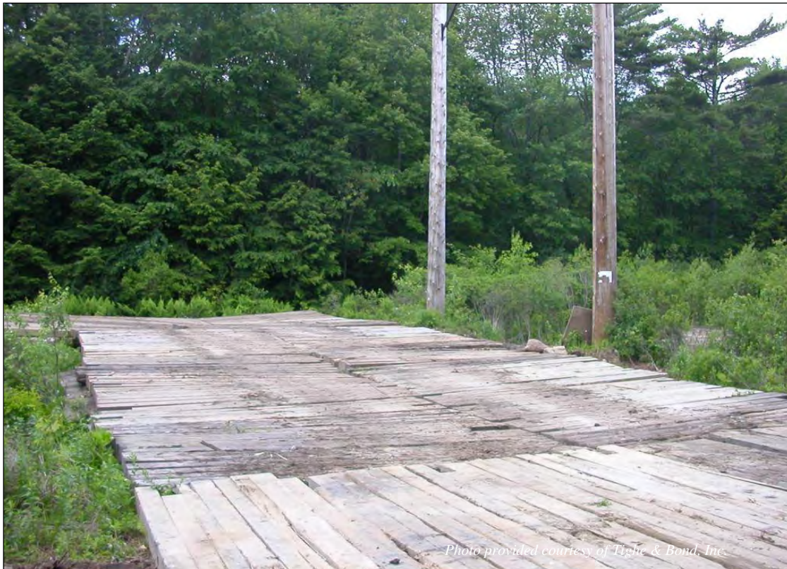
Construction mat wetland work-pad for de-energized work.
