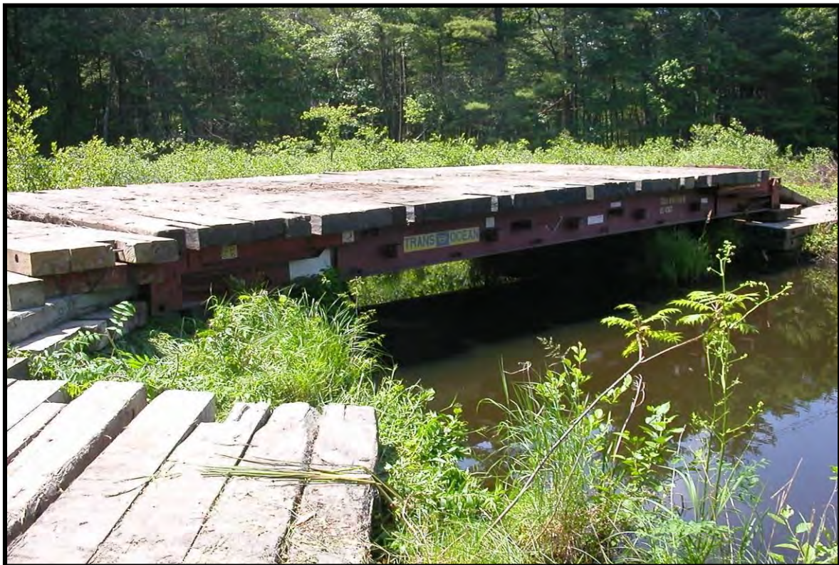
Rail car frame bridge crossing.
