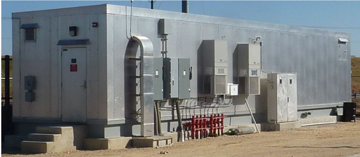
Figure G-3 Typical HPFF Pump House
