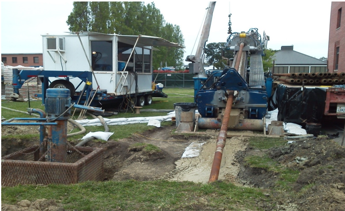
Figure K-2 Typical HDD Setup – Entry Location
