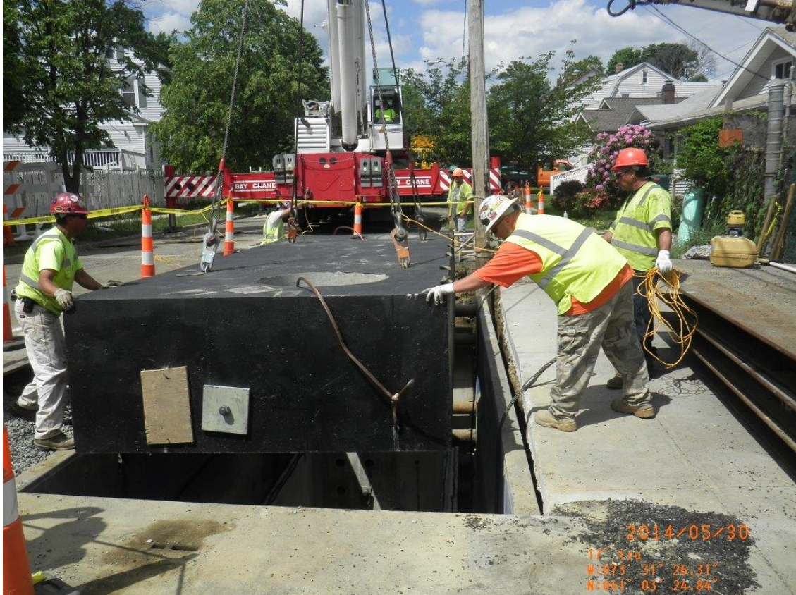
Figure G-7 Typical Splice Vault Installation
