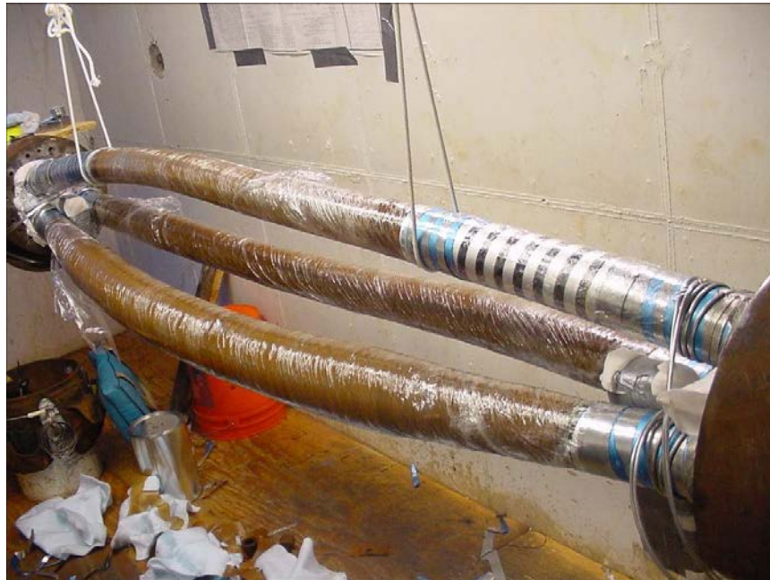
Figure K-4 Typical 115-kV HPFF Splice Assembly
