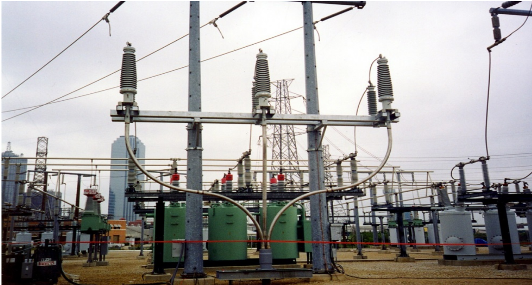
Figure K-5 Typical 115-kV HPFF Termination Structure
