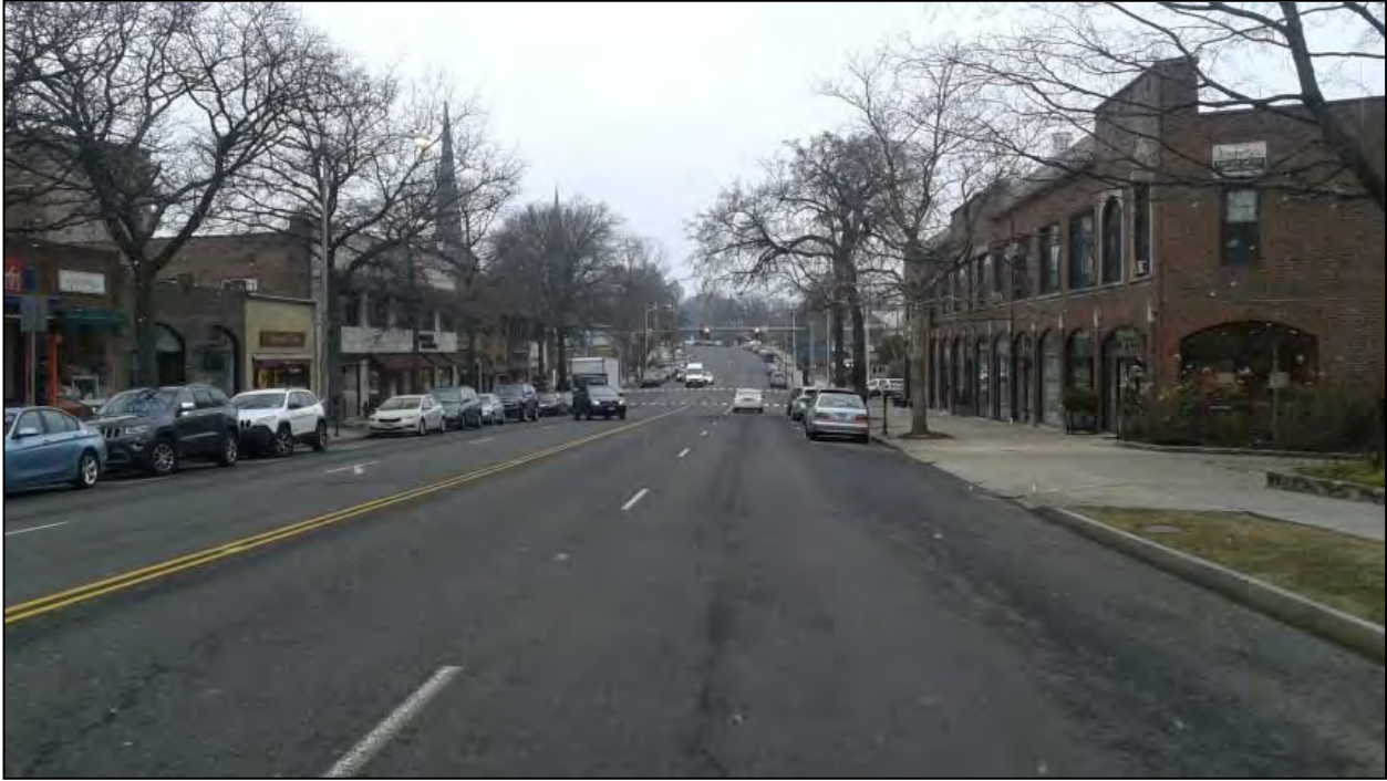
Photo 30. Overview photo of the project corridor along East Putnam Avenue facing northeast toward the Fourth Ward and Putnam Hill Historic Districts.
