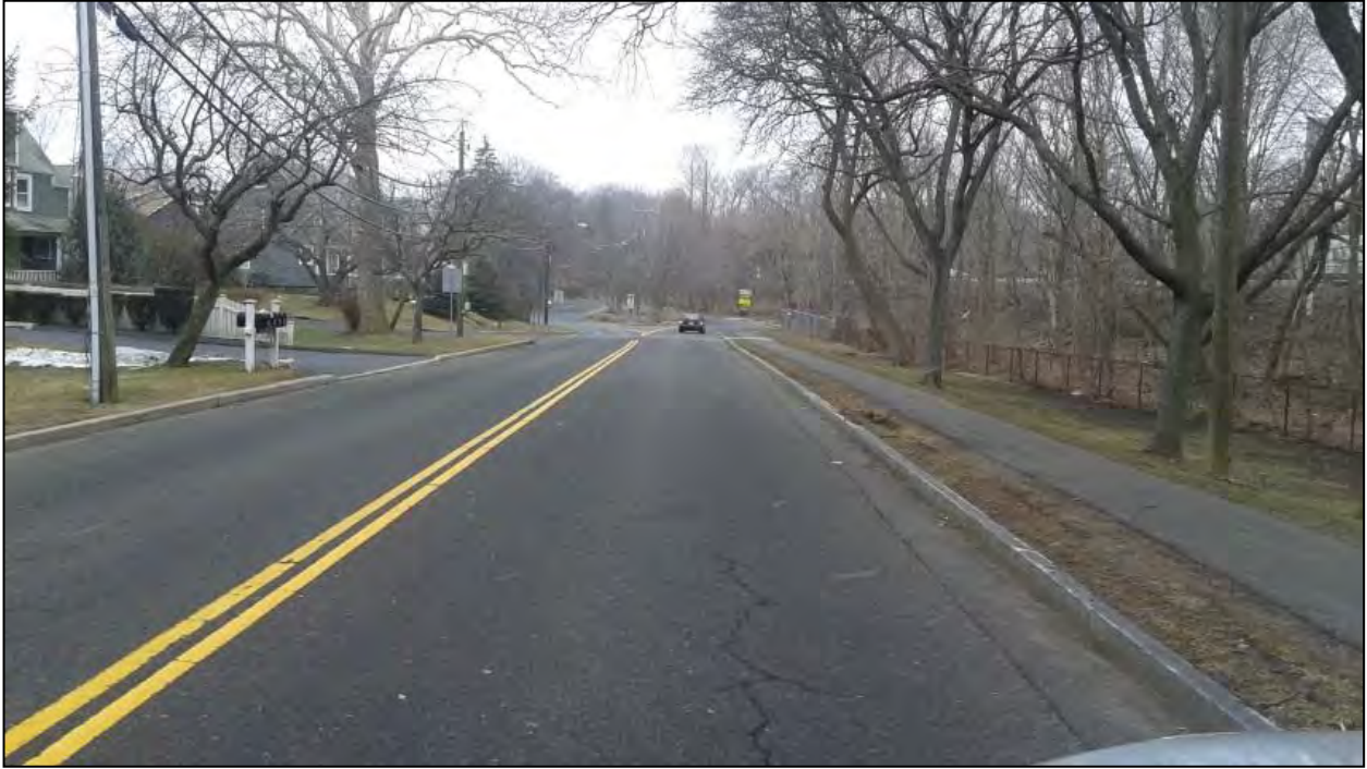
Photo 17. Overview photo of the project corridor along Davis Avenue facing west.
