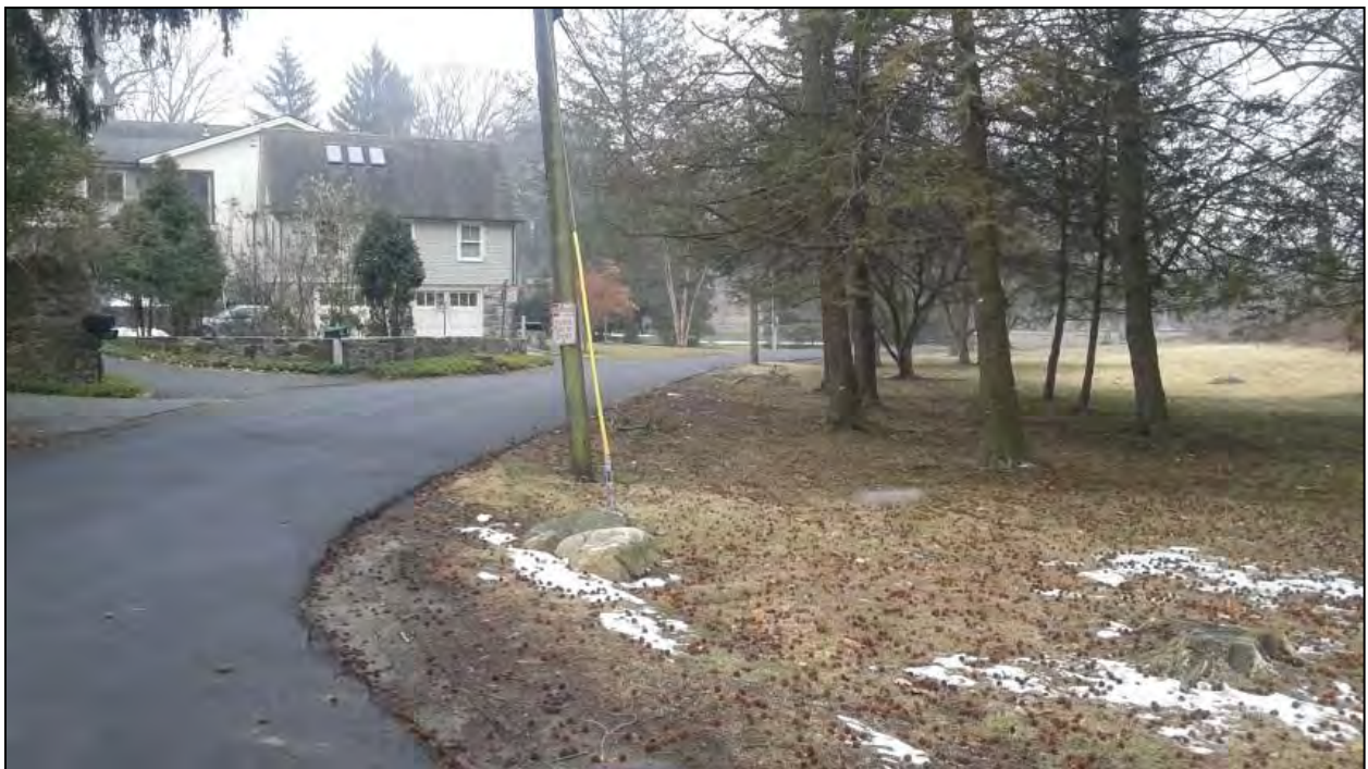
Photo 12. Overview photo of the project corridor along Kinsman Lane facing southwest.
