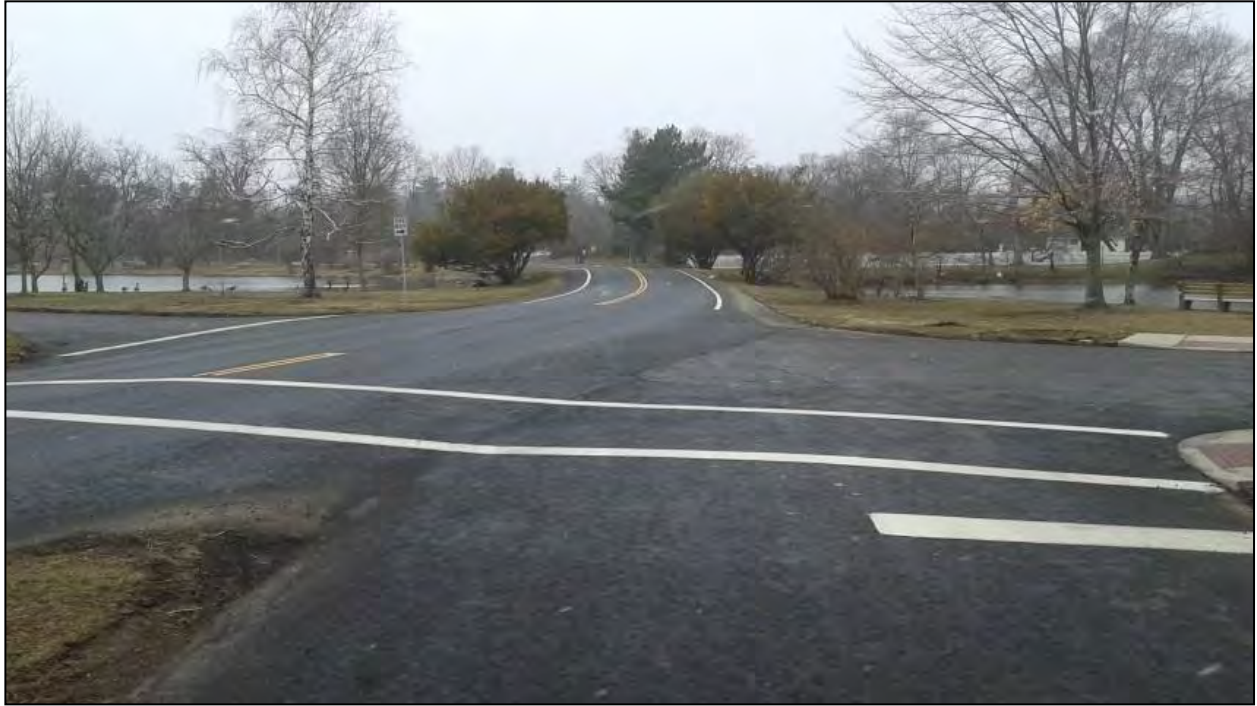
Photo 14. Overview photo of the project corridor along Davis Avenue facing southwest.
