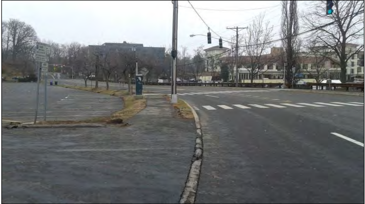
Photo 19. Overview photo of the project corridor along Arch Street facing east.
