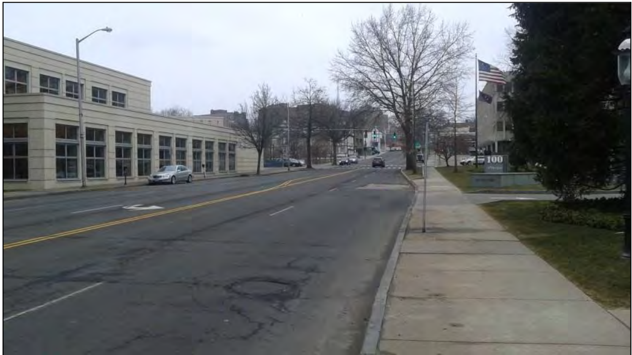
Photo 28. Overview photo of the project corridor along Field Point Road facing northeast.
