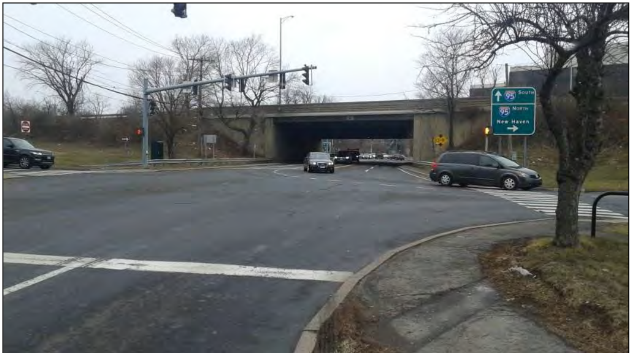
Photo 20. Overview photo of the project corridor along Arch Street facing northwest.
