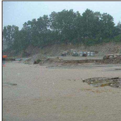
Erosion and sedimentation
