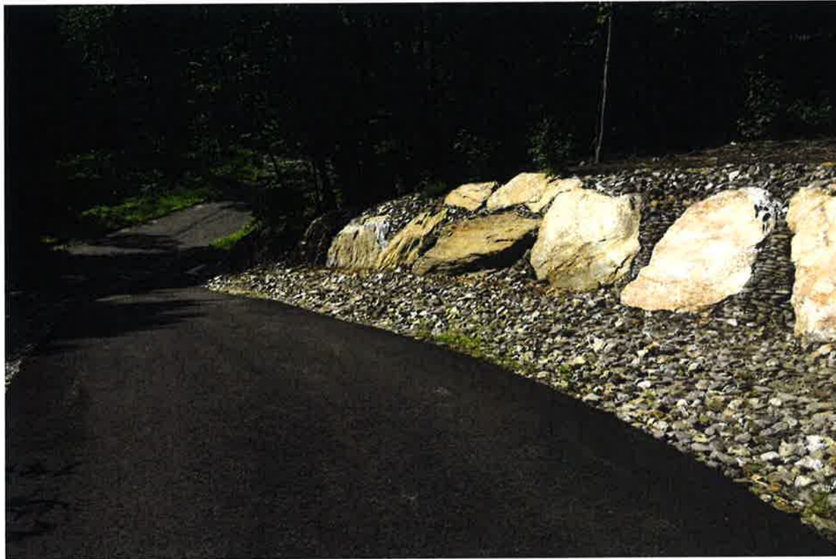
Photo 1: View of paved access road entrance looking south.
