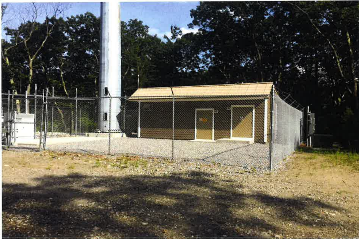
Photo 4: View of facility compound area looking northeast.
