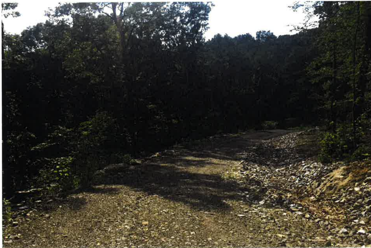
Photo 2: View of gravel access road looking south.
