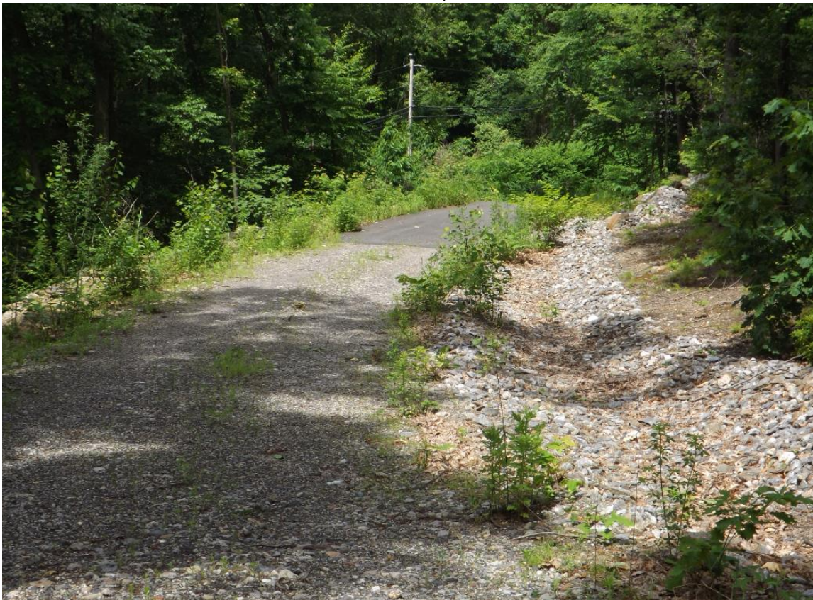
Access Drive w/Swale
