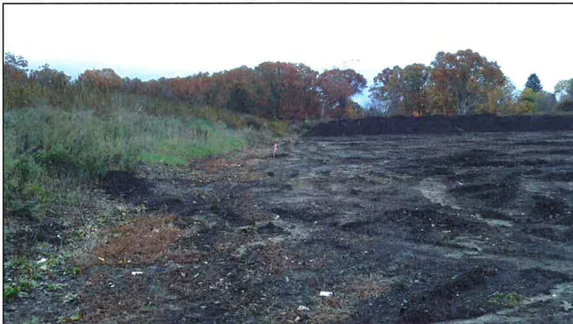
Photo 8. Overview photo of the proposed utility easement facing southeast.
