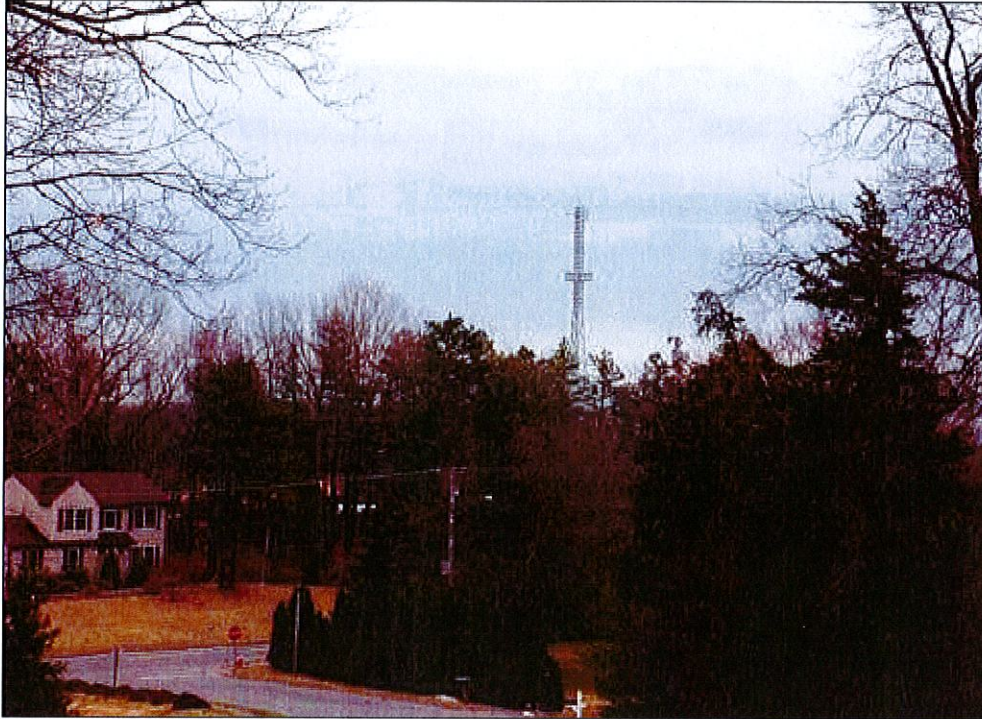
Simulation depicts AT&T antennas mounted at 140 feet above ground level. (Applicant 1, Tab 11)
