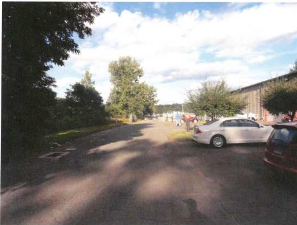
Photo 2: View of paved parking and access along north side of building, looking east.
