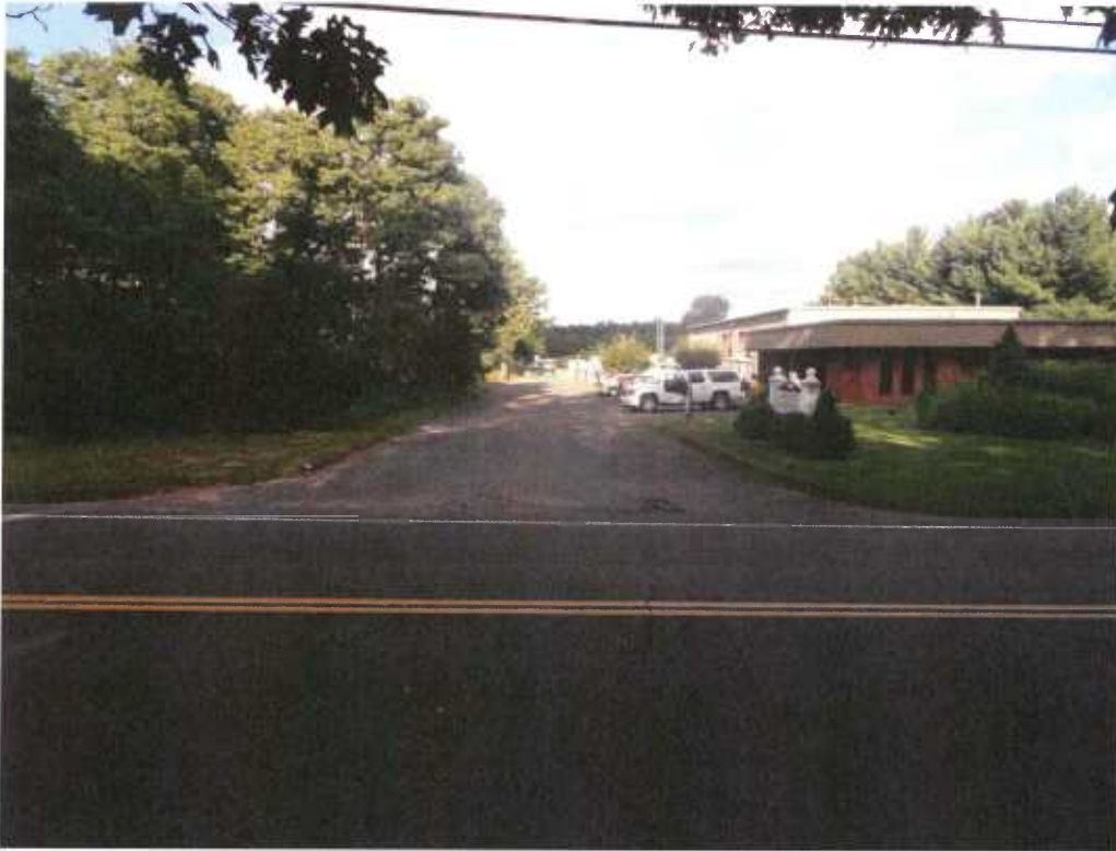
Photo 1: View of entrance to Northeast Tower's property, looking east across Brickyard Road. Northeast Tower's office/garage building in right side of photo.
