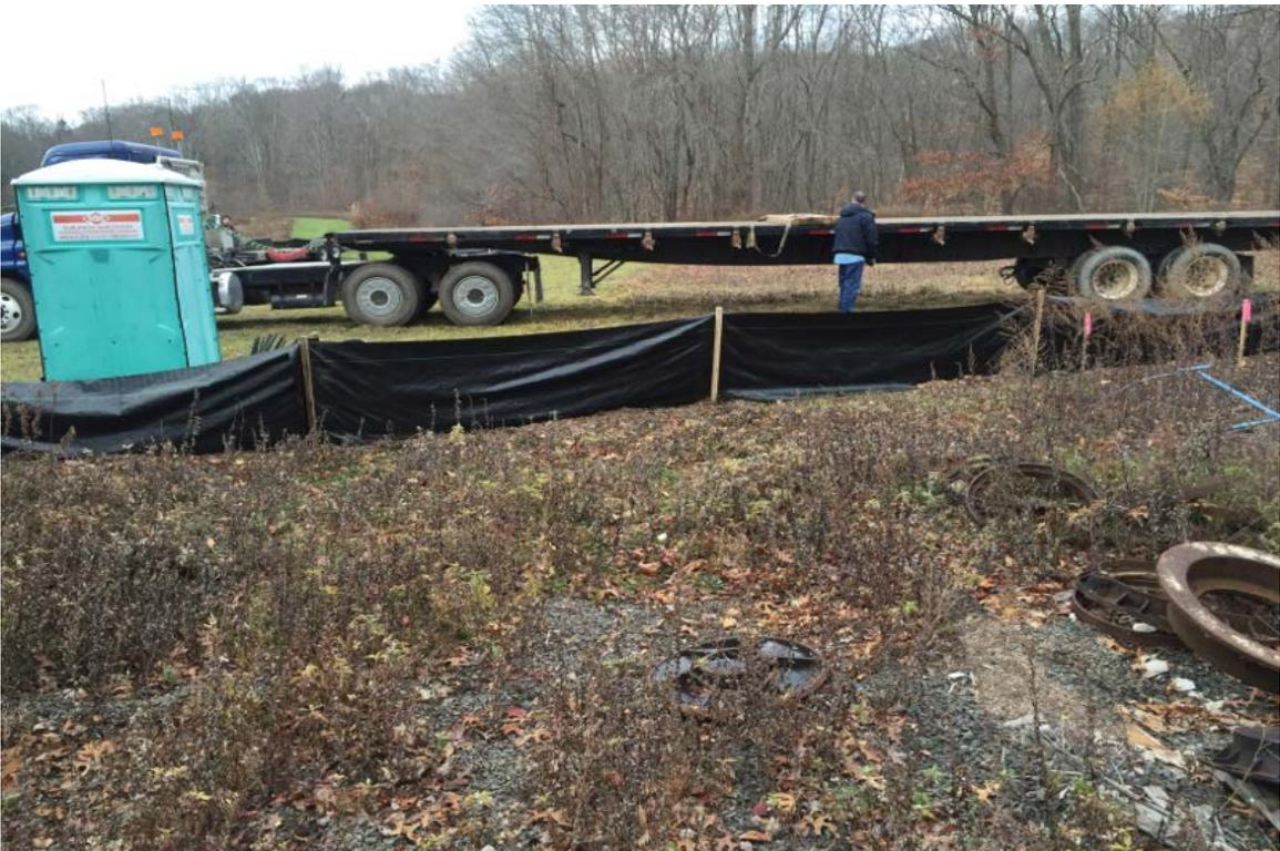
Photo 6: View of restaked silt fence (replaced broken stakes) looking west.
