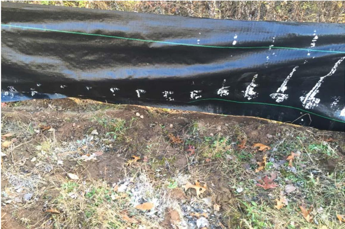
Photo 3: Corrective Area #1 - view of silt fence that needs to be trenched.
