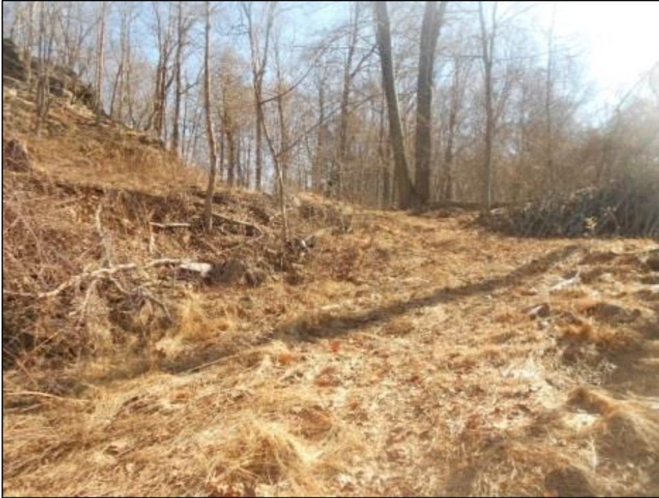
Photo 13. Overview photo of the central portion of the proposed access road facing northeast (note that the road has been cut down into the landscape at this point).
