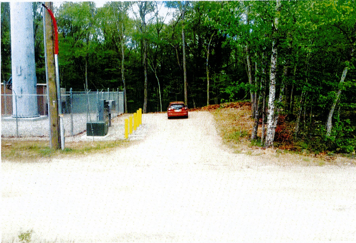
Photo 1: View of access road entrance looking northeast.
