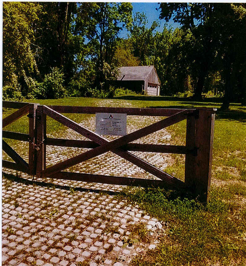
Access road wood gate and grass pavers.
