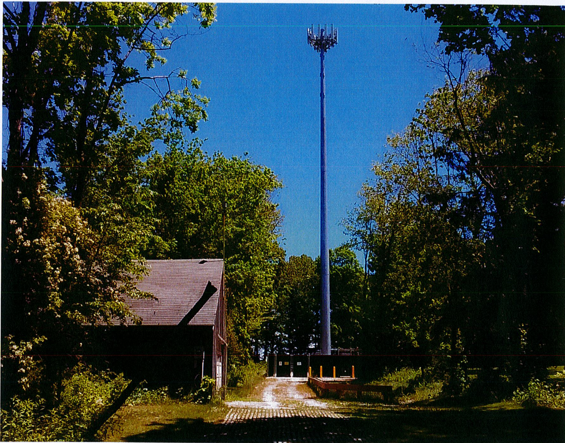
View of tower from access drive.
