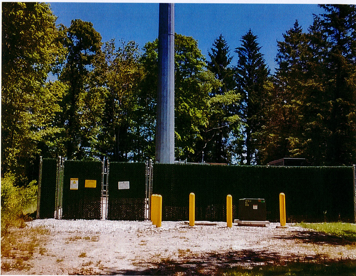
Compound entrance area.
