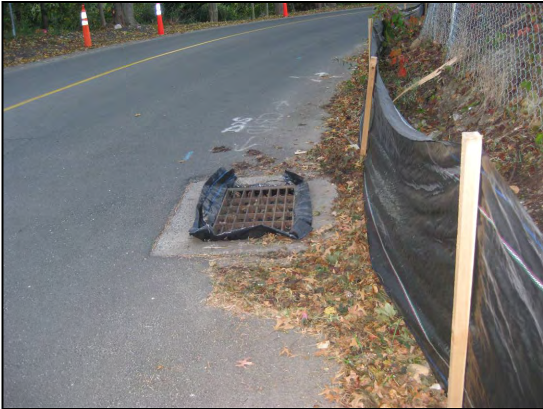
Catchbasin protected from sedimentation by filter fabric.
