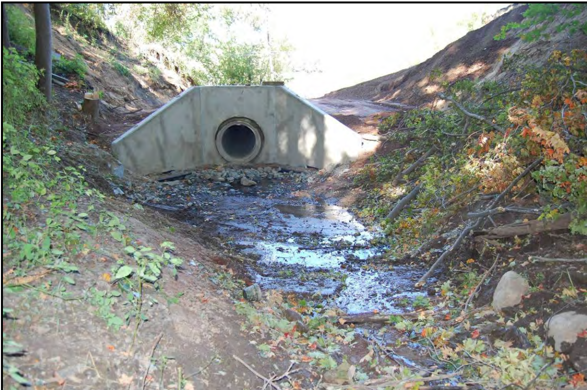
Installing a pipe culvert.
