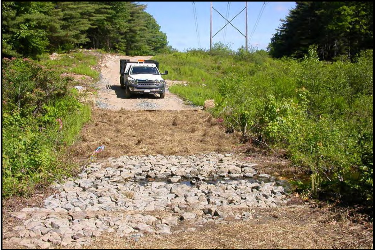
Intermittent stream crossing with angular stone.
