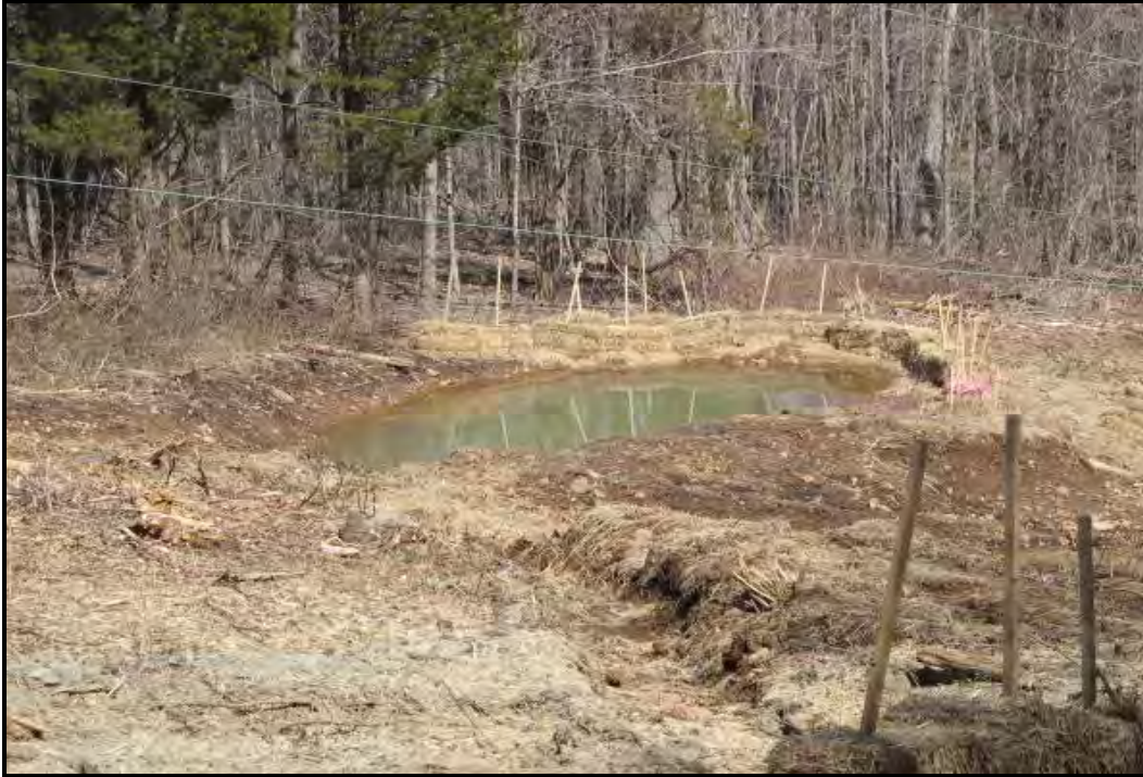
Sedimentation basin with haybale filters.
