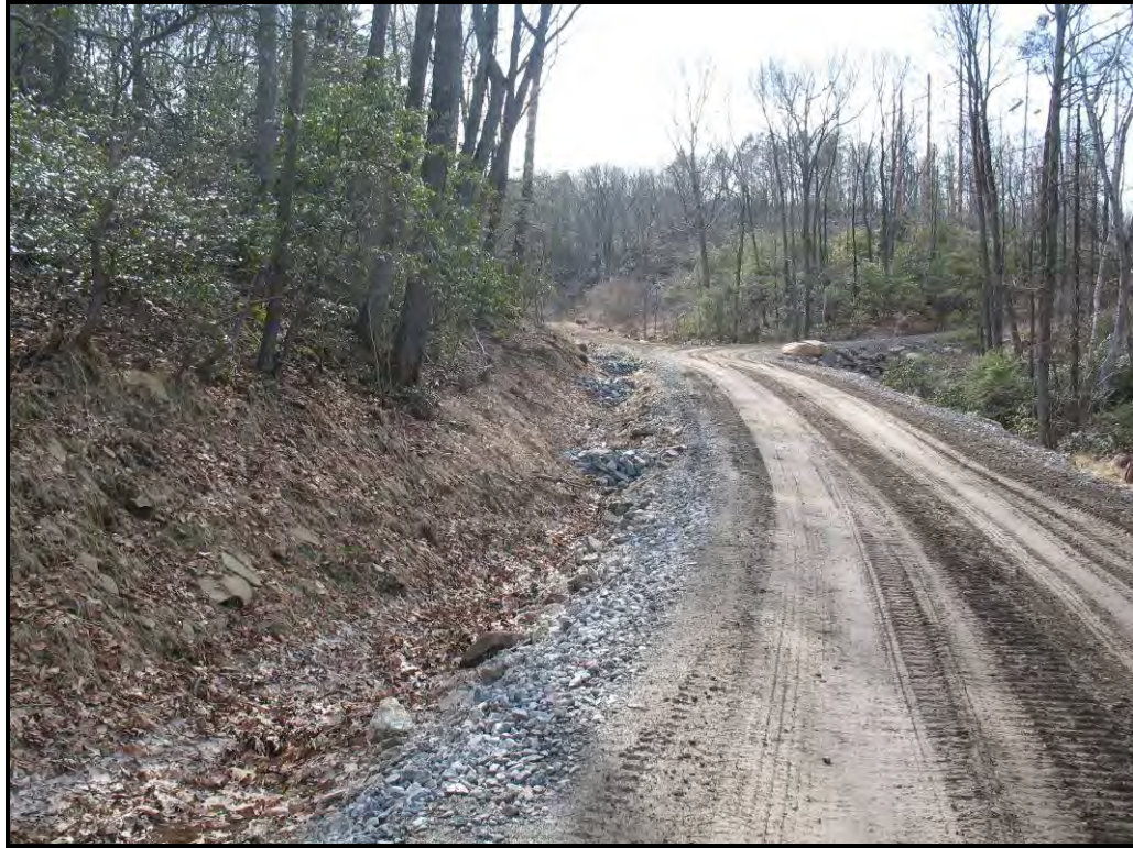
Stone check dams at construction site.
