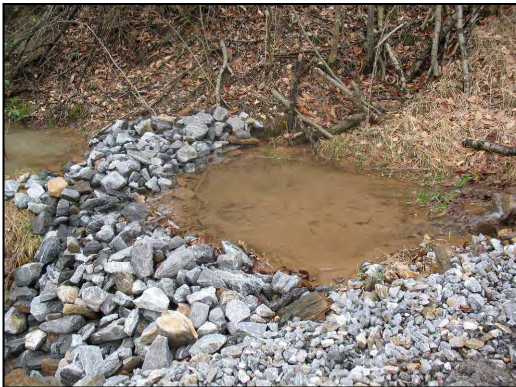
Stone check dam at construction site.
