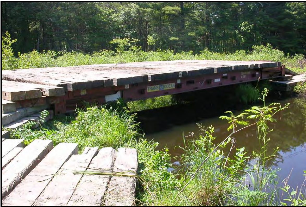
Rail car bridge crossing.
