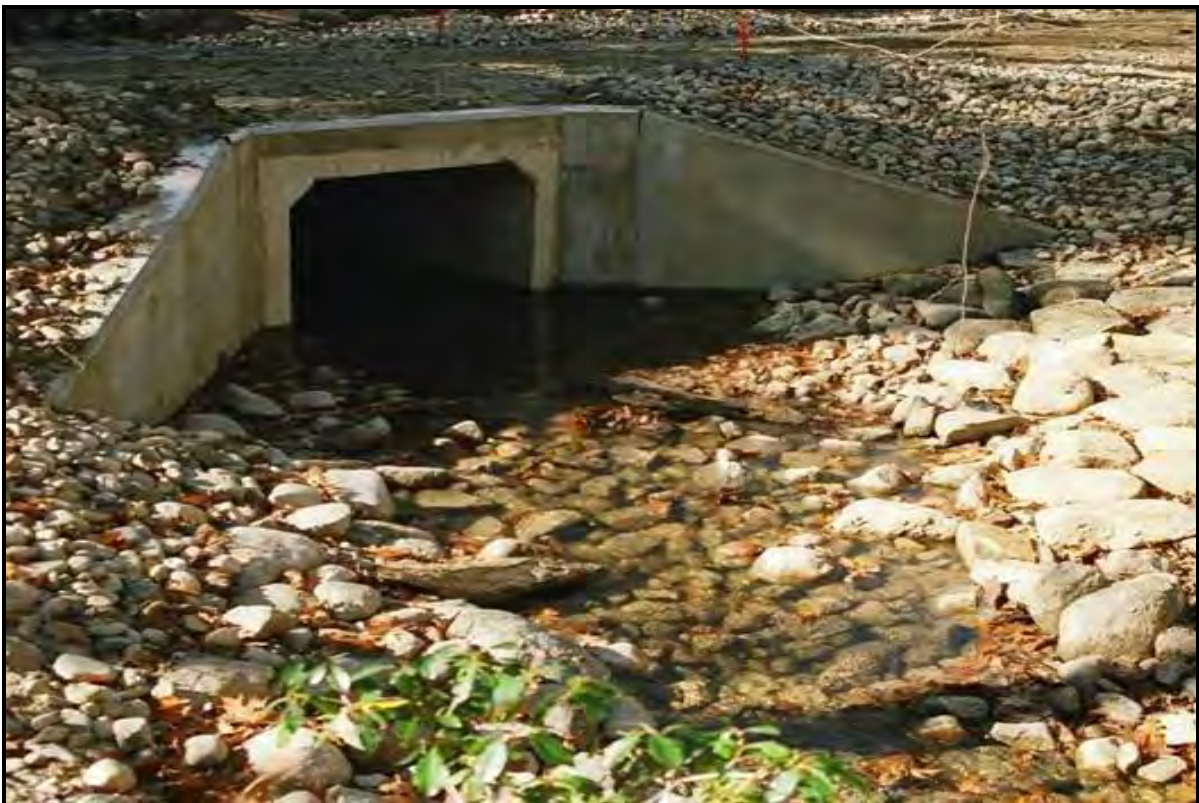
Embedded box culvert with wing walls.
