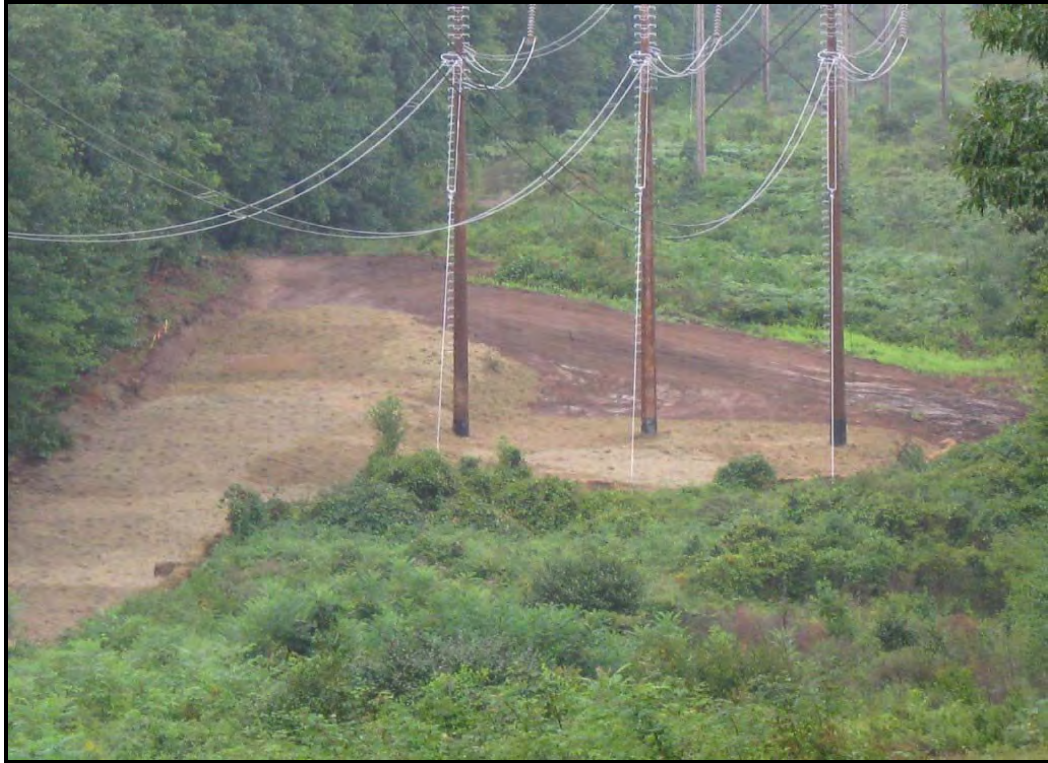
Loaming and seeding of recently disturbed right-of-way.
