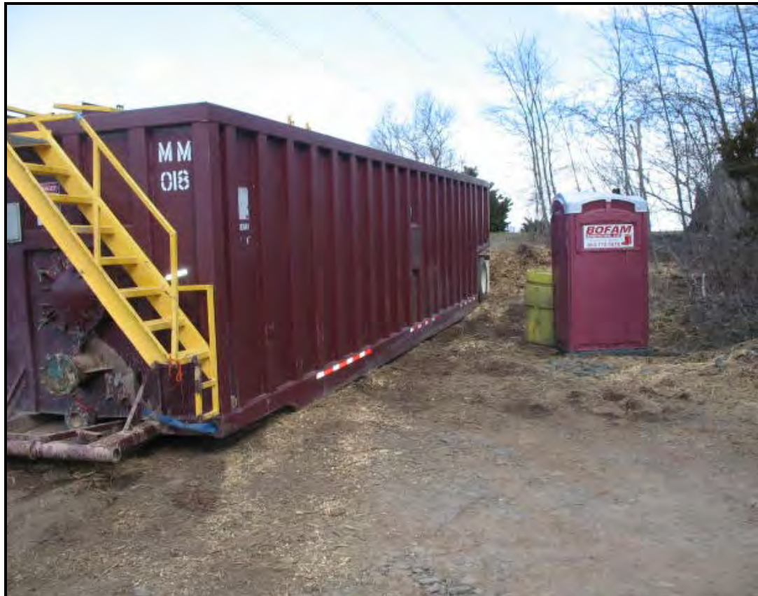
Frac tank on-site for dewatering activities.
