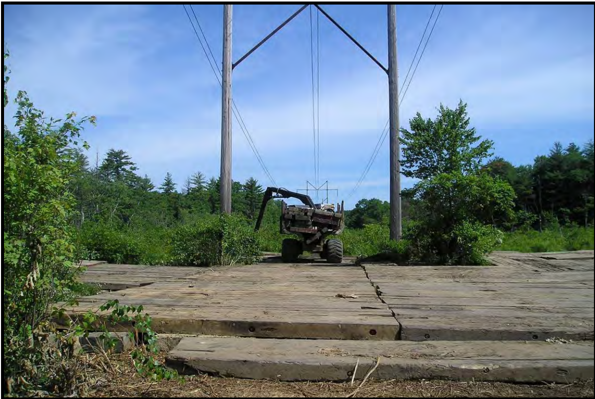
Timber mat wetland work platform.
