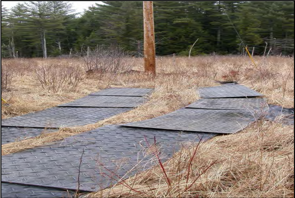
AlturnaMAT® tracks to utility pole in wetland.
