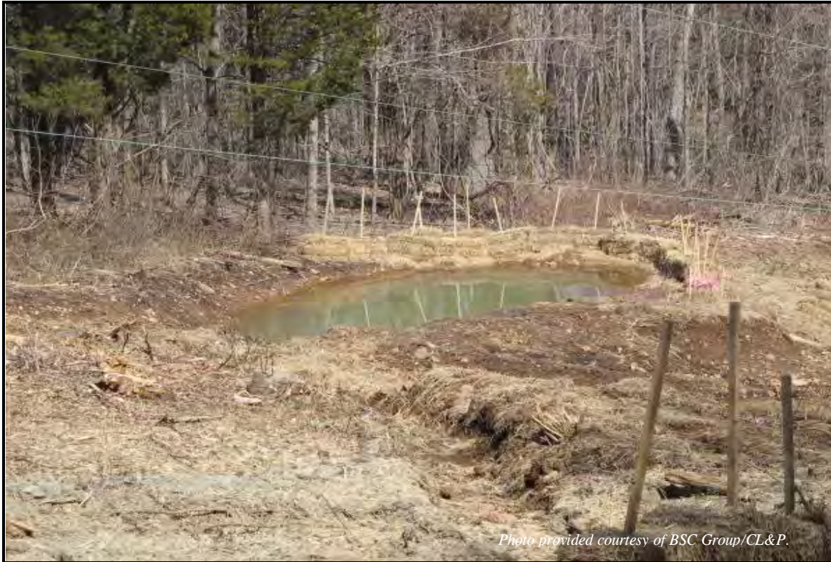
Sedimentation basin with haybale filters.
