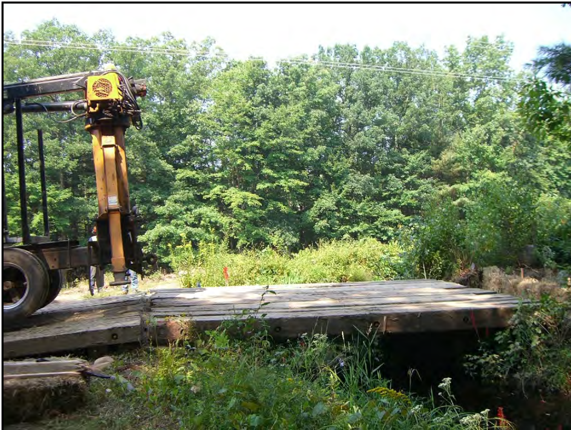
Timber mat bridge.
