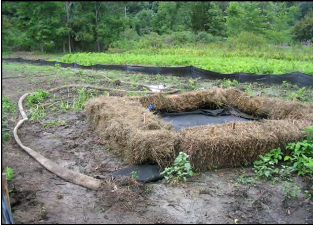
Dewatering to filter "sock" surrounded by haybales.
