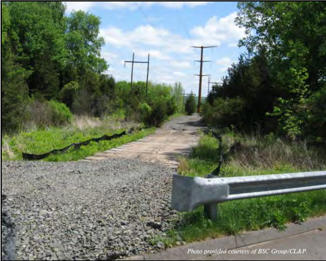
Construction entrance track pad.
