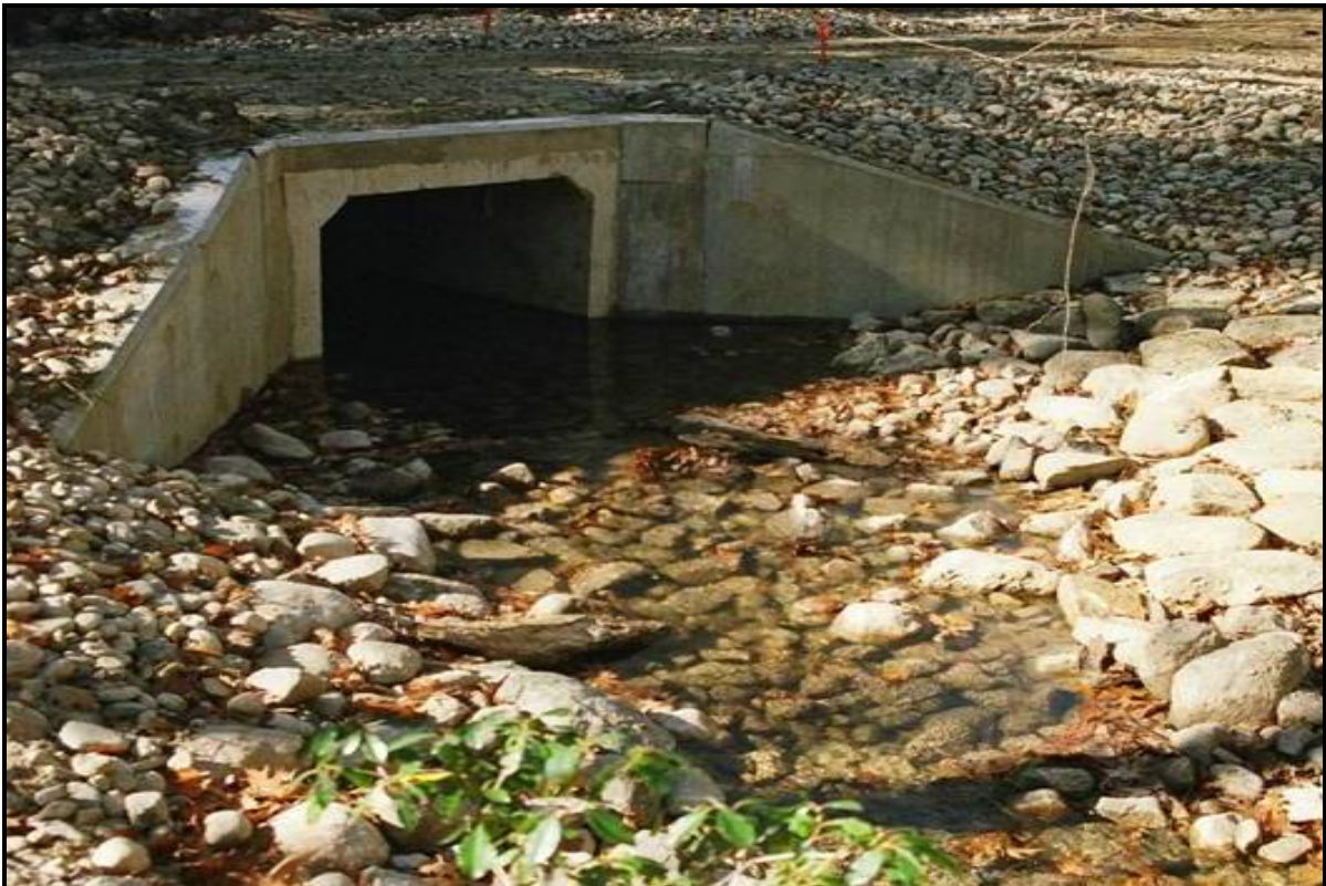
Embedded box culvert with wing walls.
