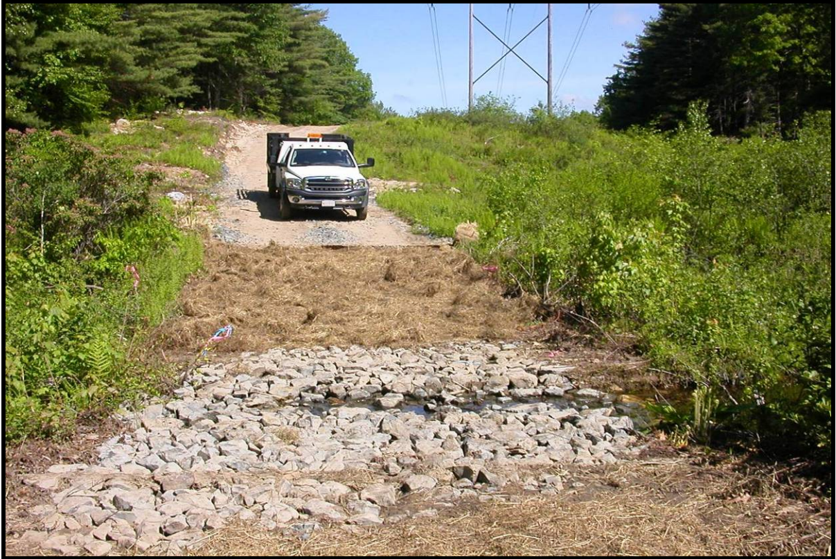
Intermittent stream crossing with angular stone.
