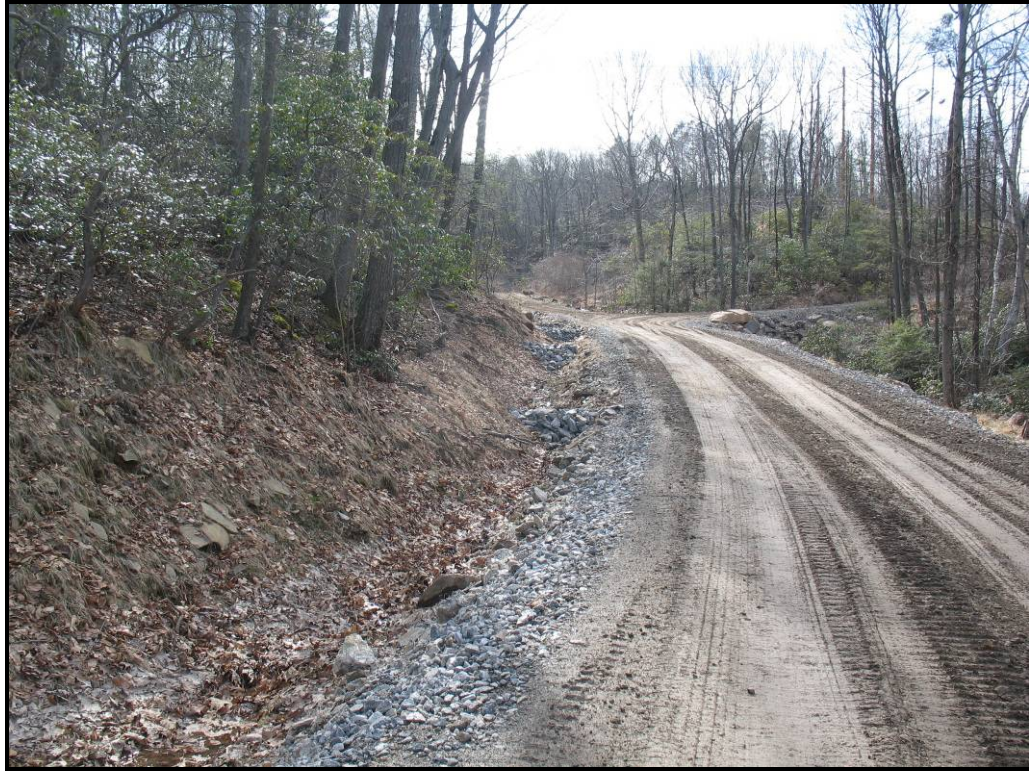
Stone check dams at construction site.
