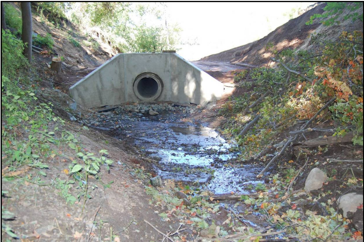
Installing a pipe culvert.
