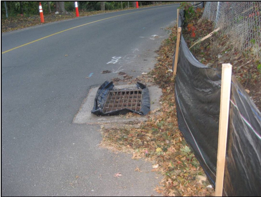
Catchbasin protected from sedimentation by filter fabric.
