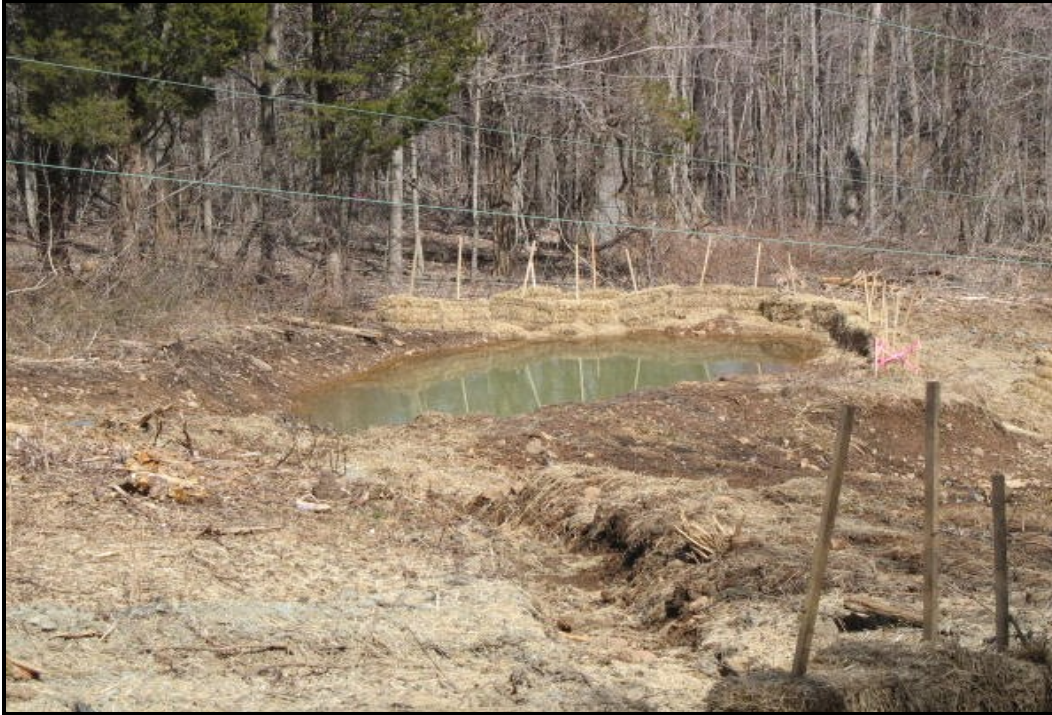
Sedimentation basin with haybale filters.
