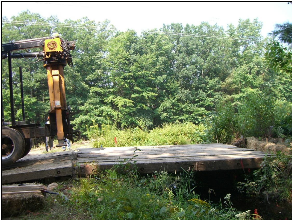
Timber mat bridge.
