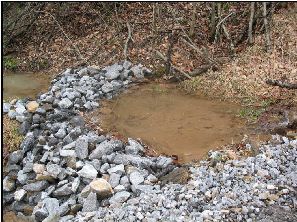
Stone check dam at construction site.
