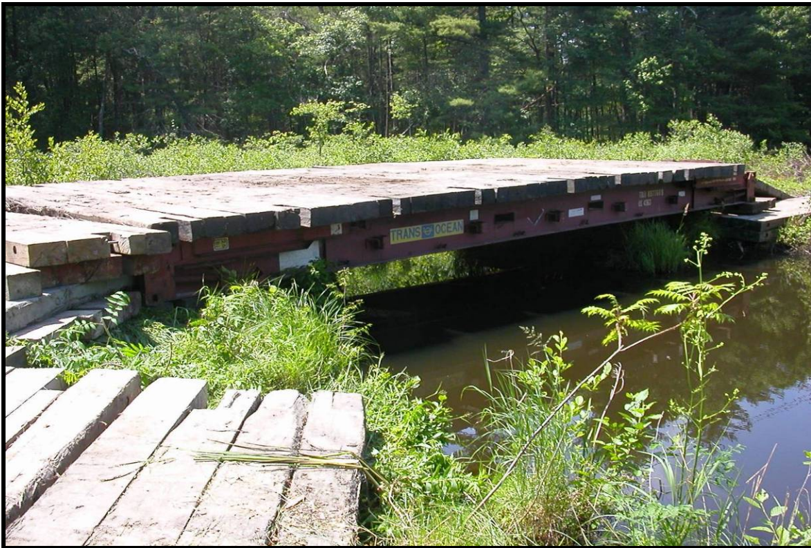
Rail car bridge crossing.
