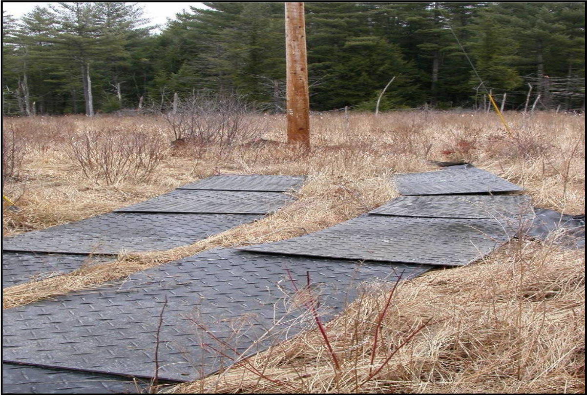
AlturnaMAT® tracks to utility pole in wetland.
