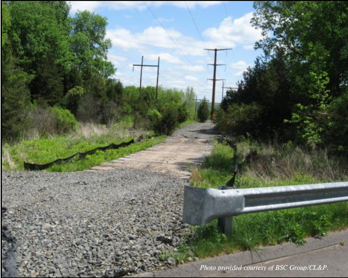
Construction entrance track pad.
