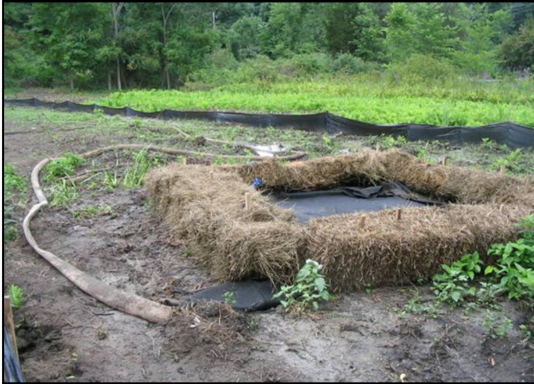
Dewatering to filter "sock" surrounded by haybales.
