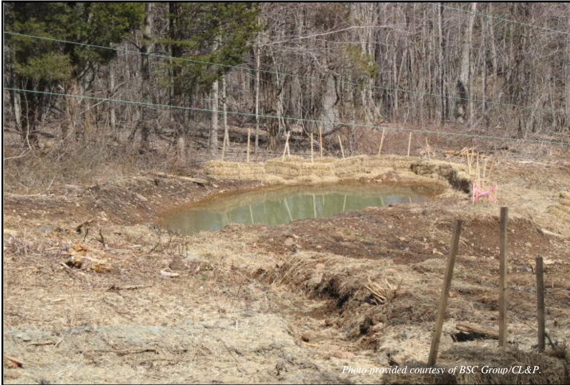
Sedimentation basin with haybale filters.
