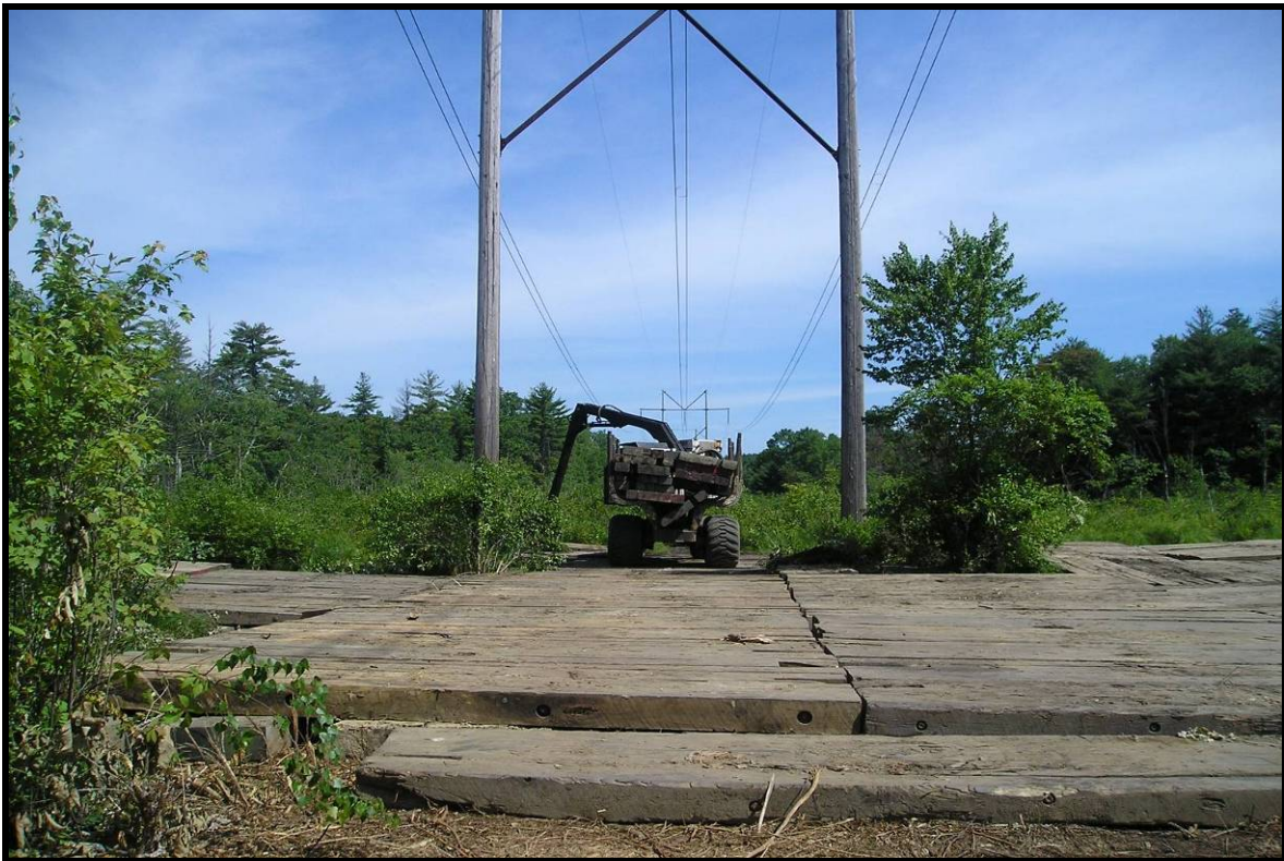
Timber mat wetland work platform.
