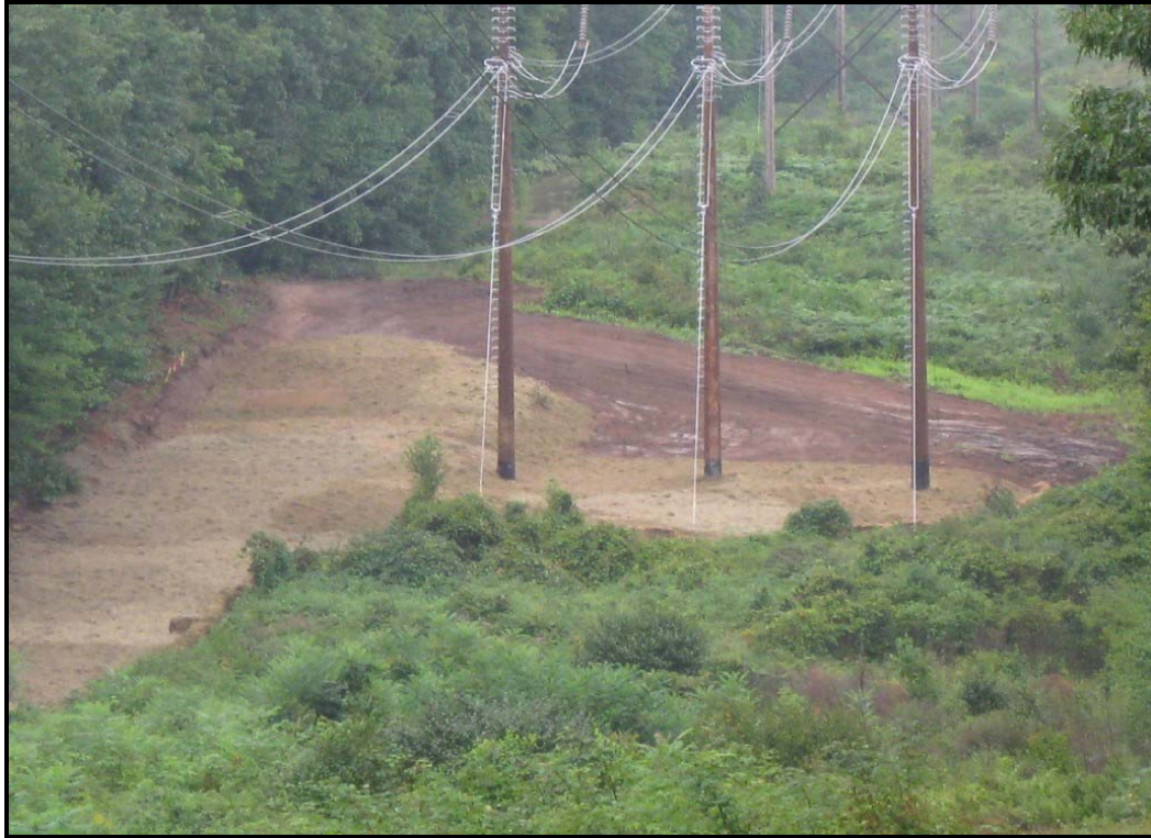
Loaming and seeding of recently disturbed right-of-way.
