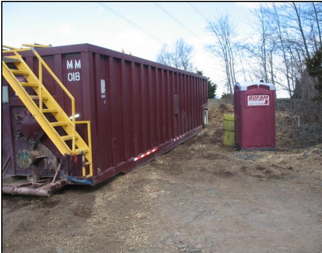
Frac tank on-site for dewatering activities.
