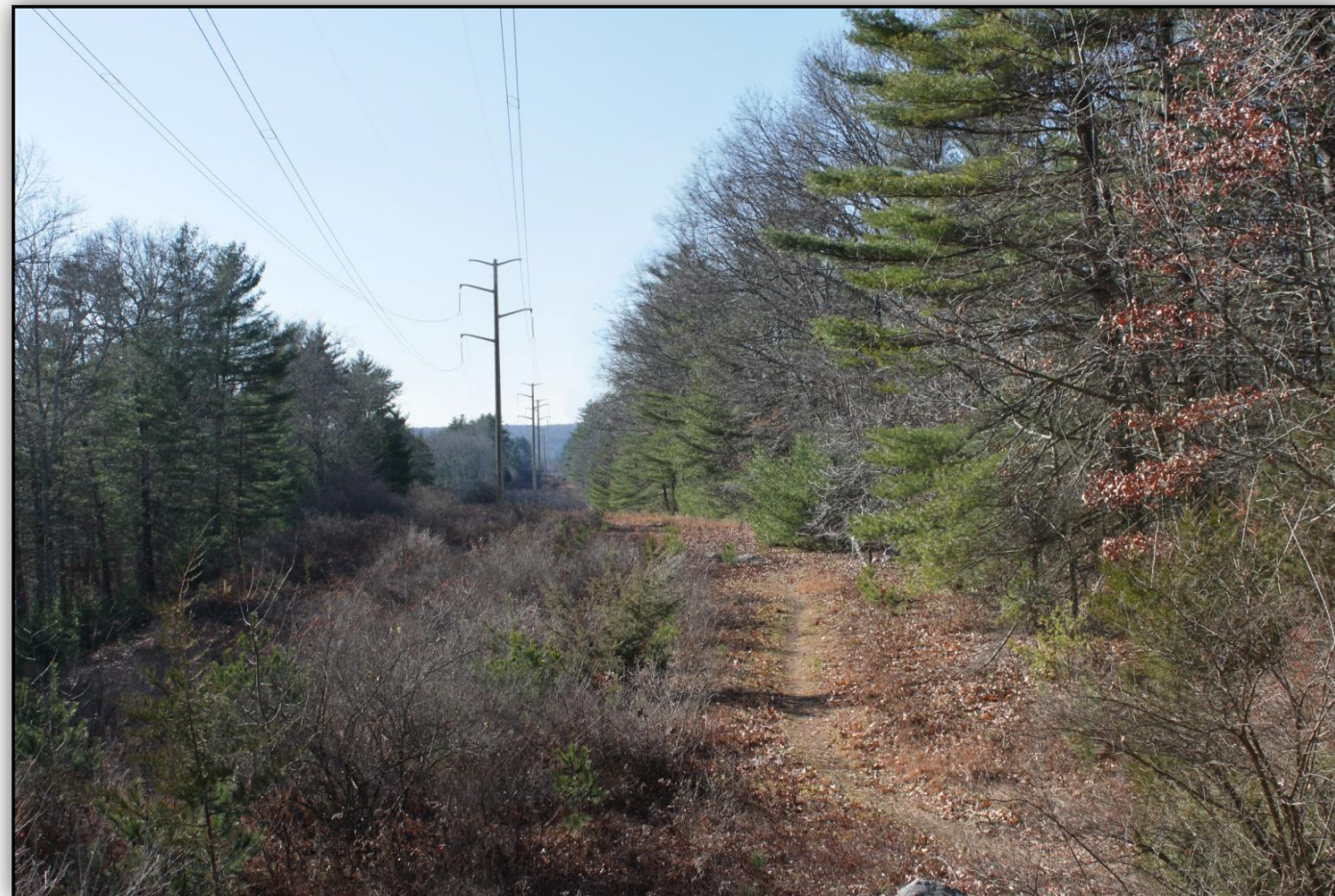
(Existing View – Leaf-off Condition)
