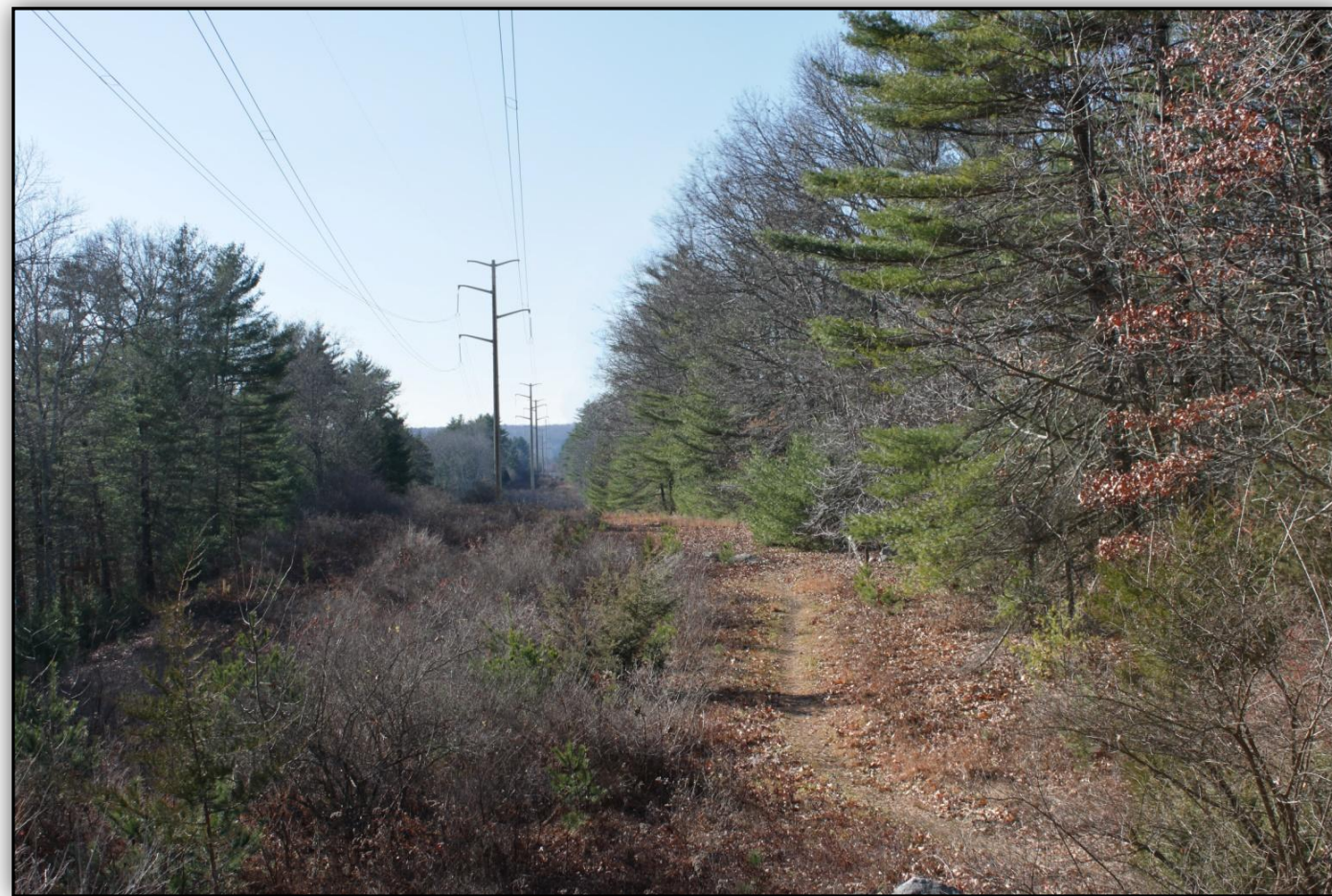
(Existing View – Leaf-off Condition)
