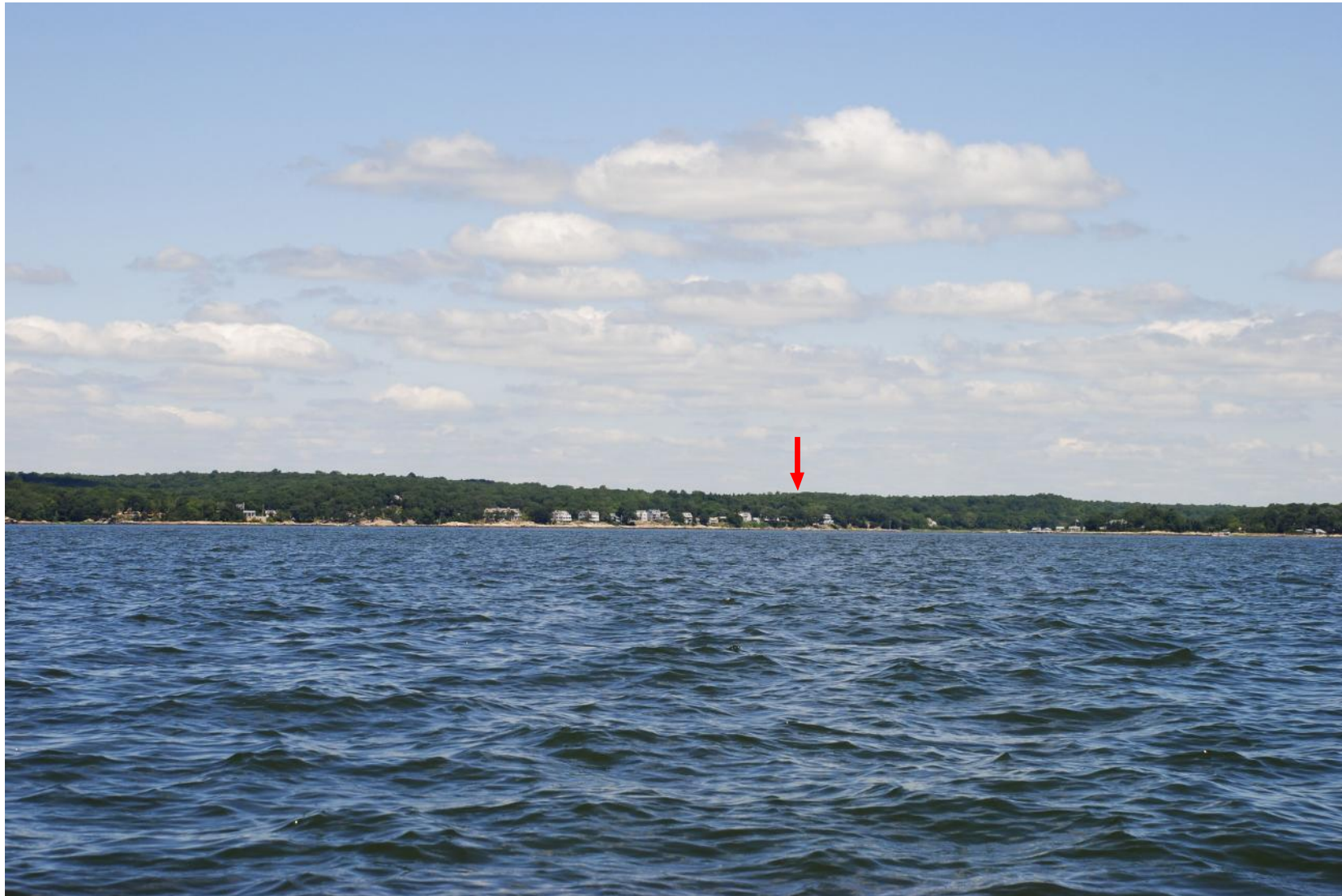
Photosim for conceptual purposes only - actual antenna & equipment locations to be determined based on final engineering design
