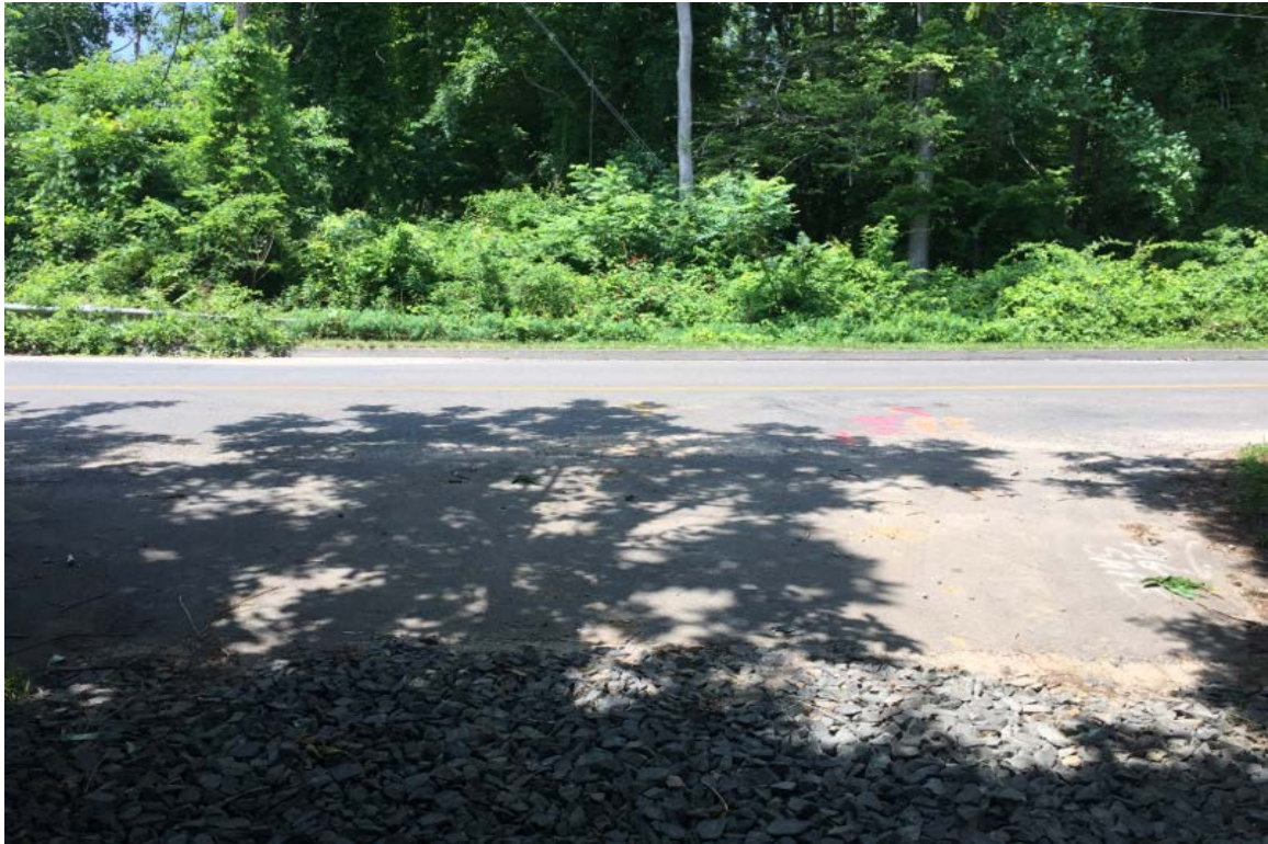
Photo 1: View of Moose Hill Road looking west.
