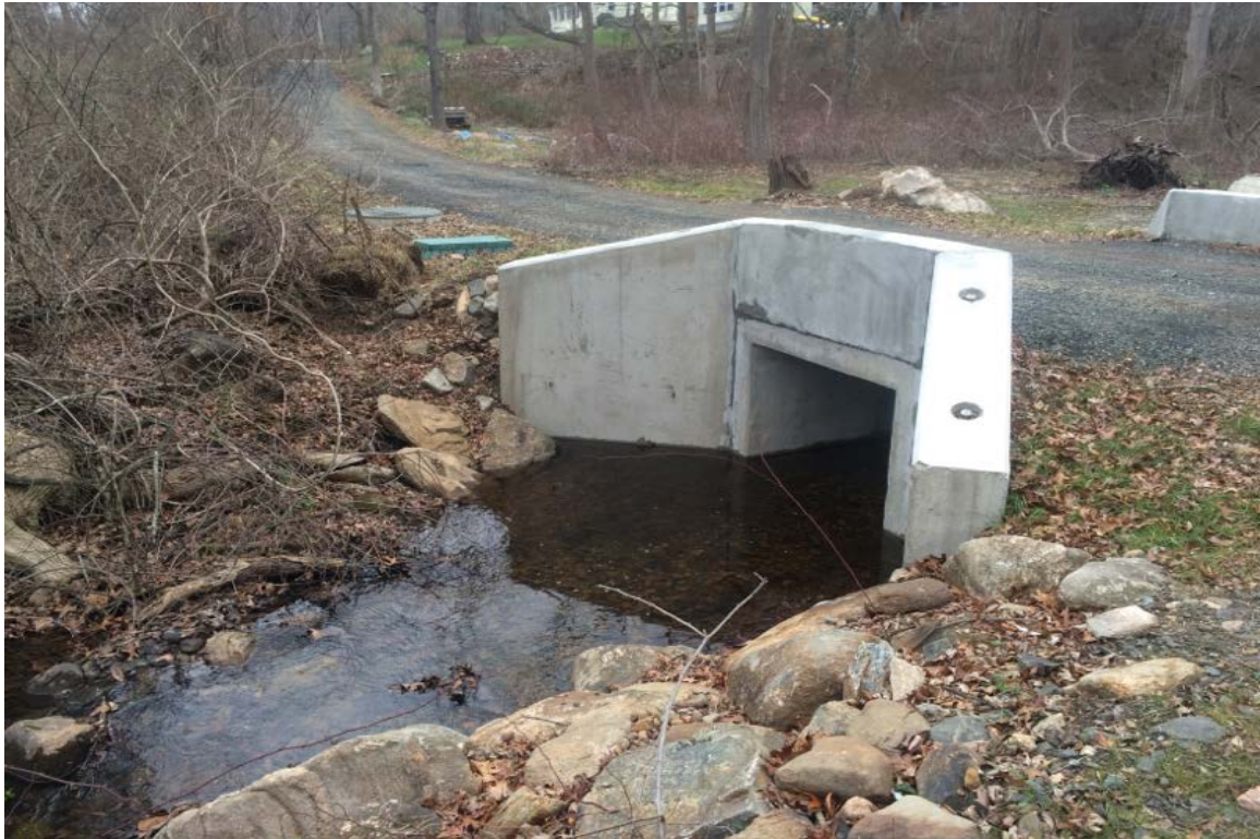
Photo 7: View of stabilized culvert crossing outlet looking west.
