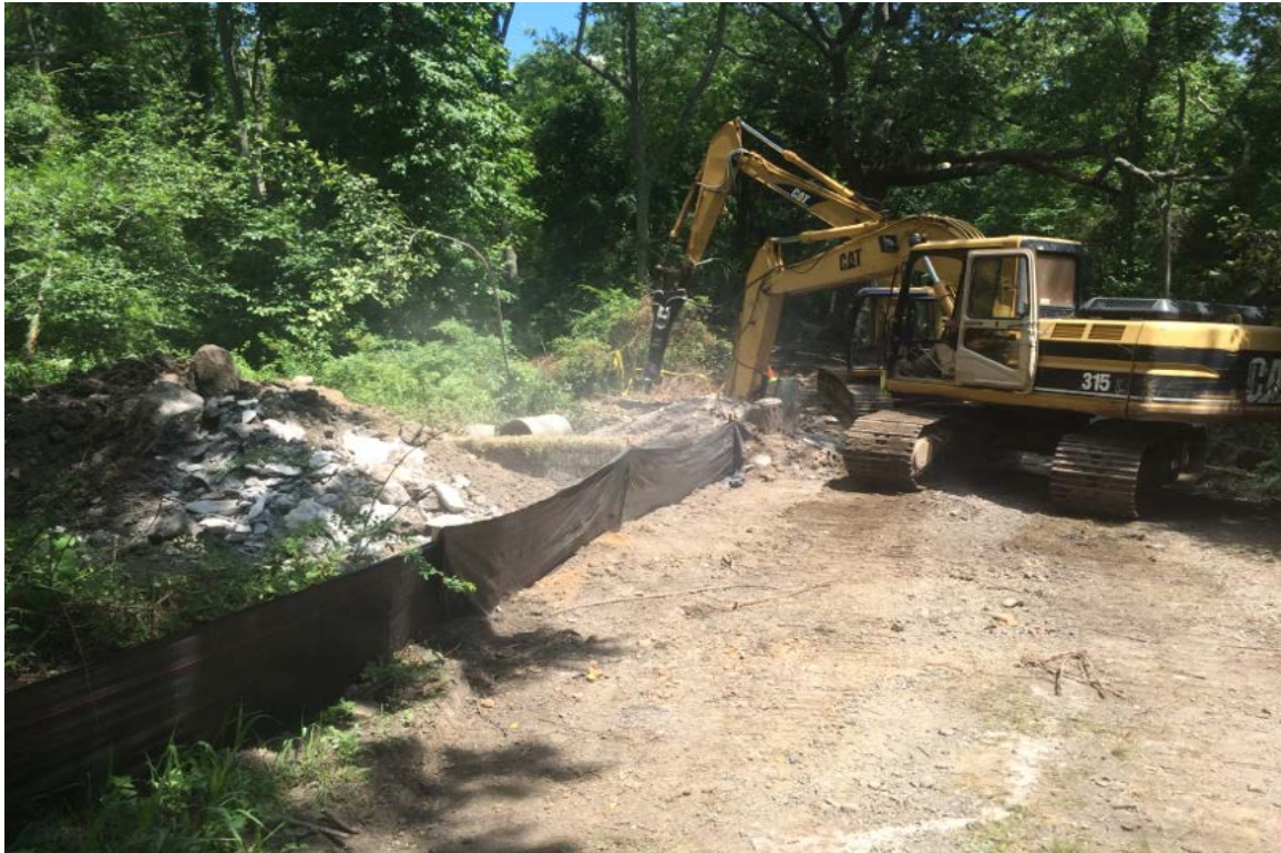
Photo 1: View of new stream crossing culvert in mid construction looking east.
