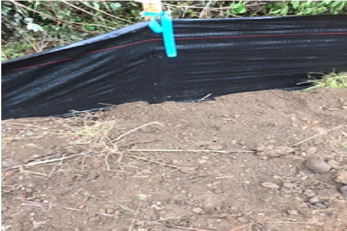
Photo 3: View of properly buried silt fence flap (typ.), looking north.
