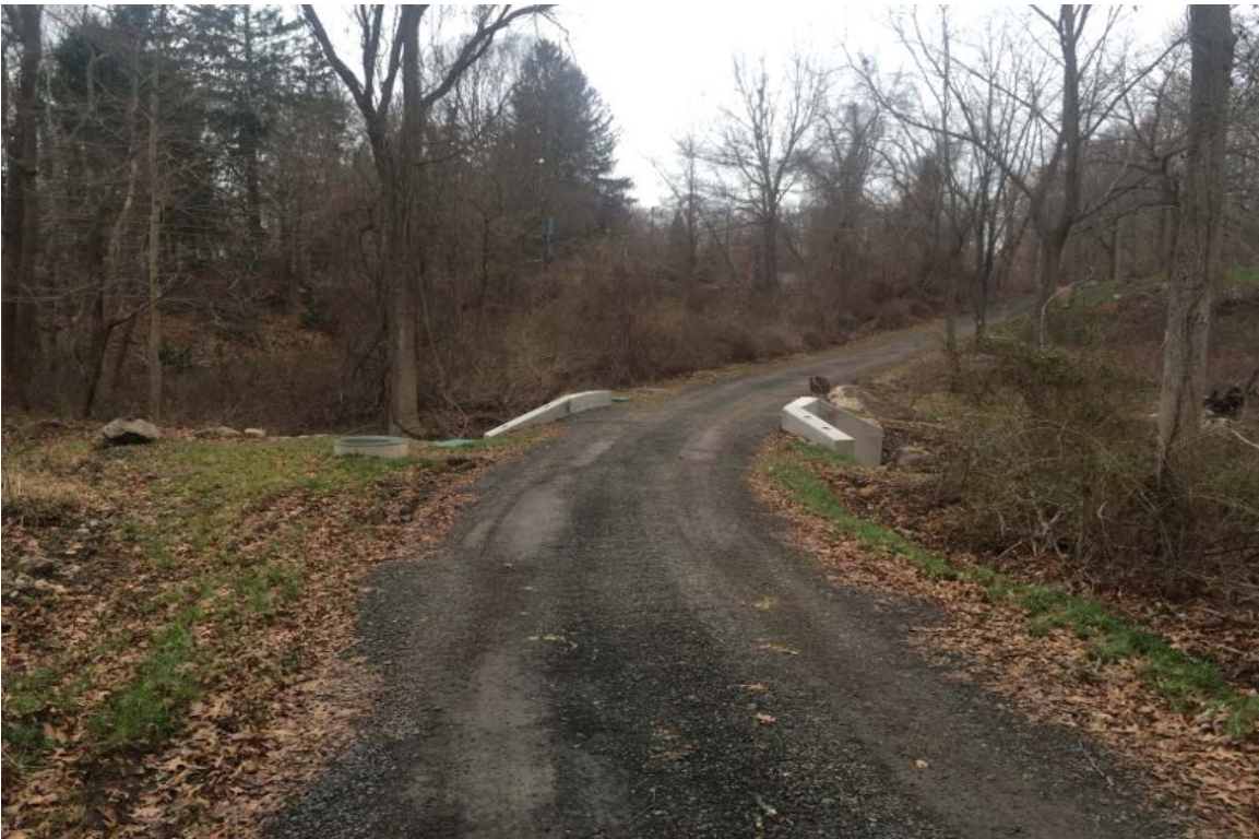
Photo 4: View of stabilized culvert crossing looking west.
