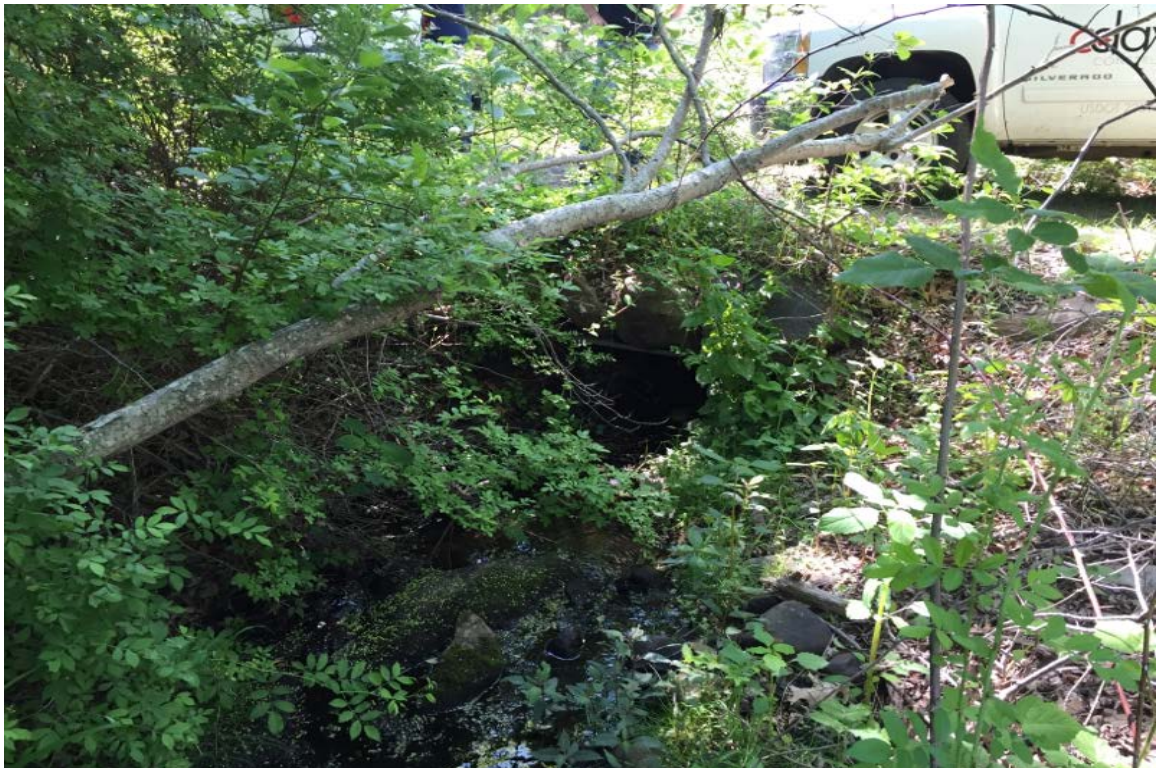
Photo 2: View of existing stream culvert crossing north side looking south.
