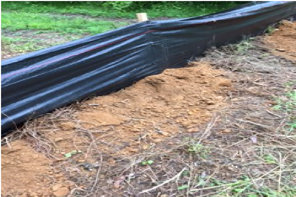
Photo 2: View of properly buried silt fence flap (typ.), looking north.
