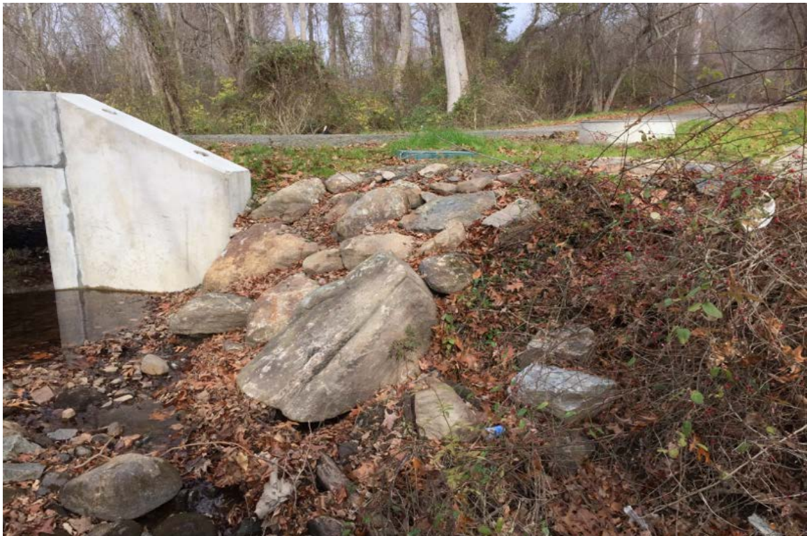
Photo 4: View of permanently stabilized southeast bank.
