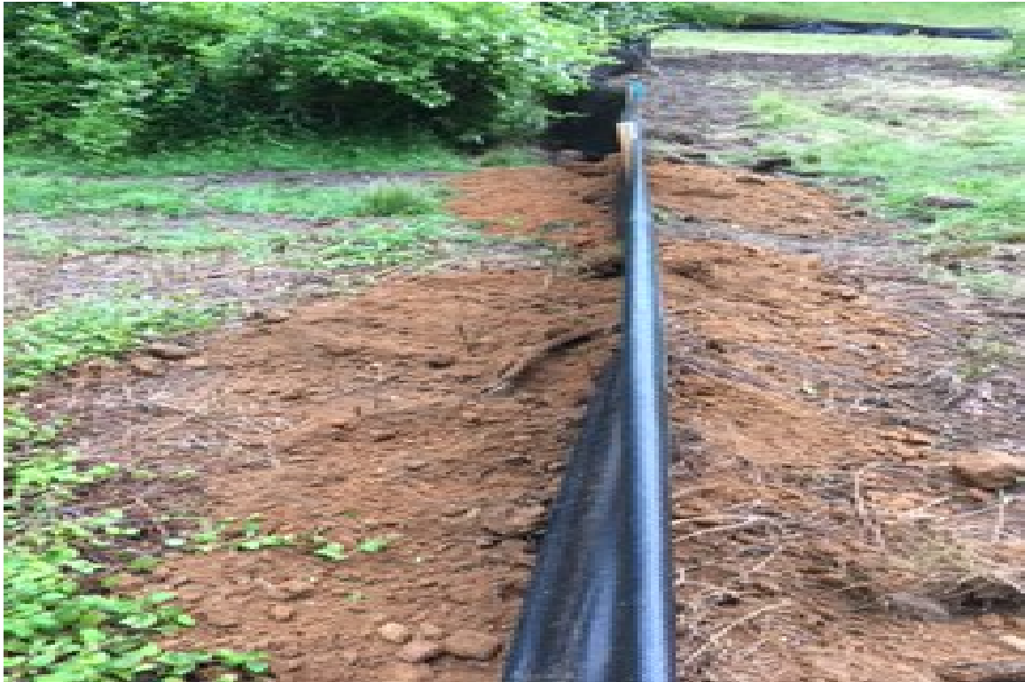
Photo 1: View of properly buried silt fence flap (typ.), looking east.
