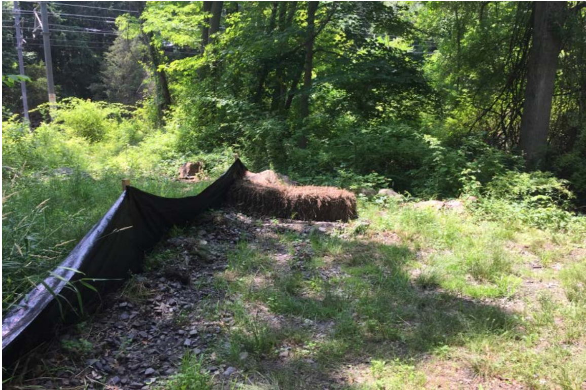
Photo 5: View of southeast side of culvert looking southwest correction area #1 bales need to be staked down.
