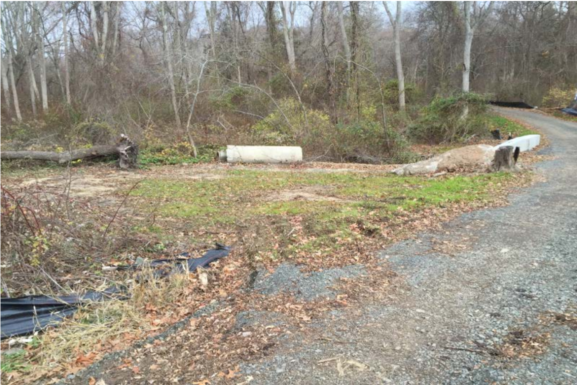
Photo 5: View of stream crossing staging area permanently stabilized looking northeast.
