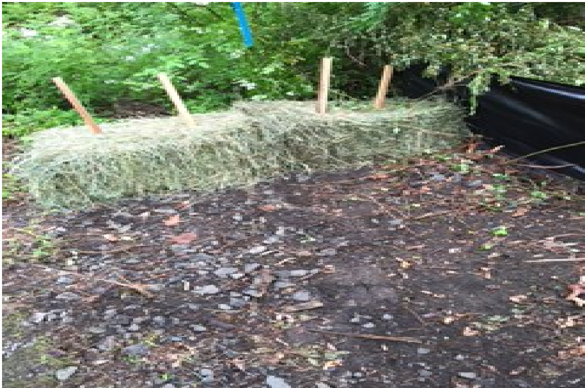
Photo 4: View of straw bales check dam near stream crossing, looking east.
