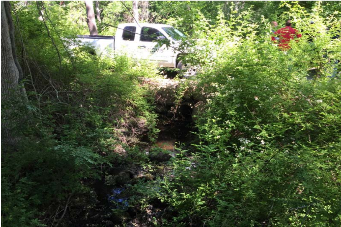
Photo 3: View of existing stream culvert crossing south side looking north.
