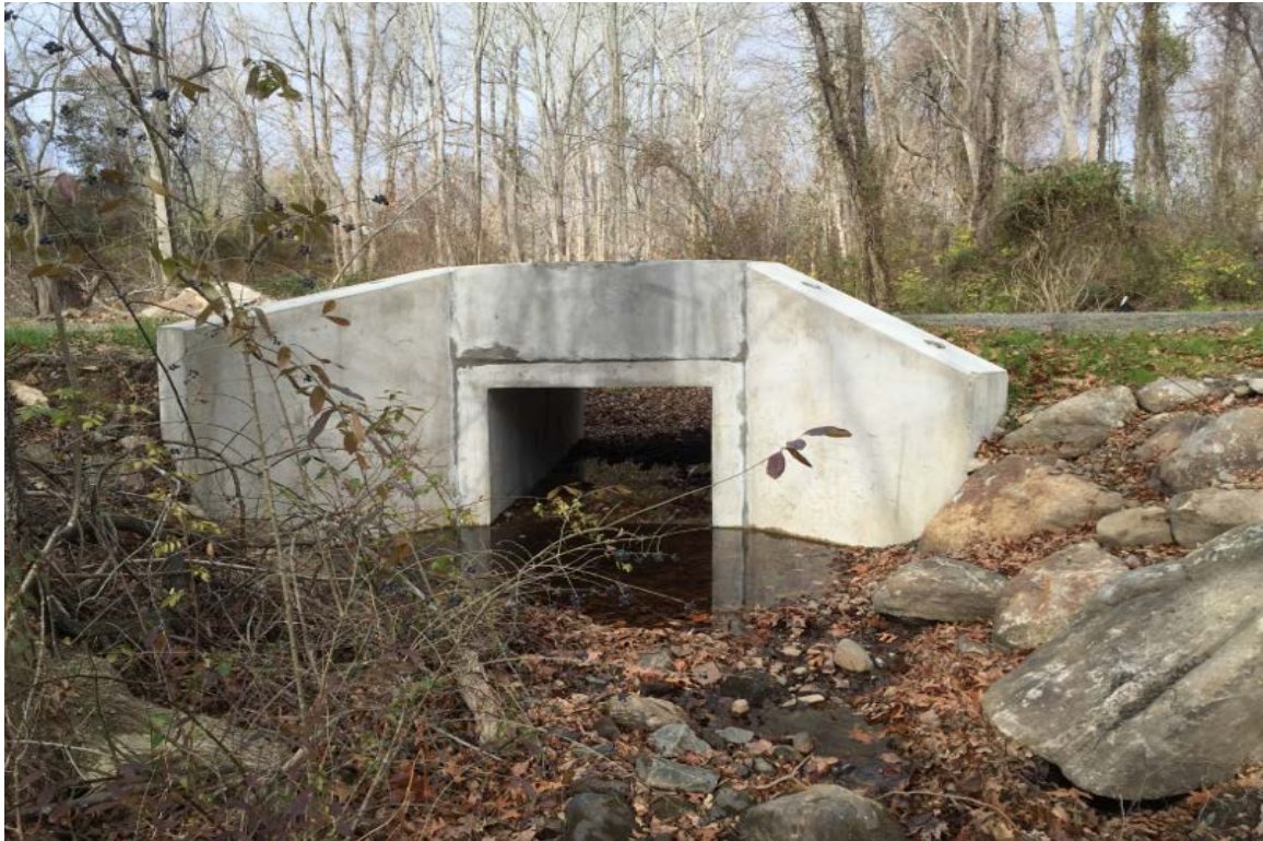
Photo 3: View of south side of stabilized culvert looking northwest.
