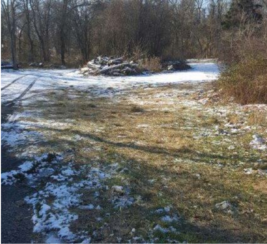
Photo 9: View of seeded and mulched construction staging area looking southwest.
