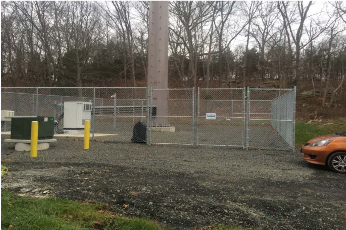
Photo 1: View of stabilized compound looking east.
