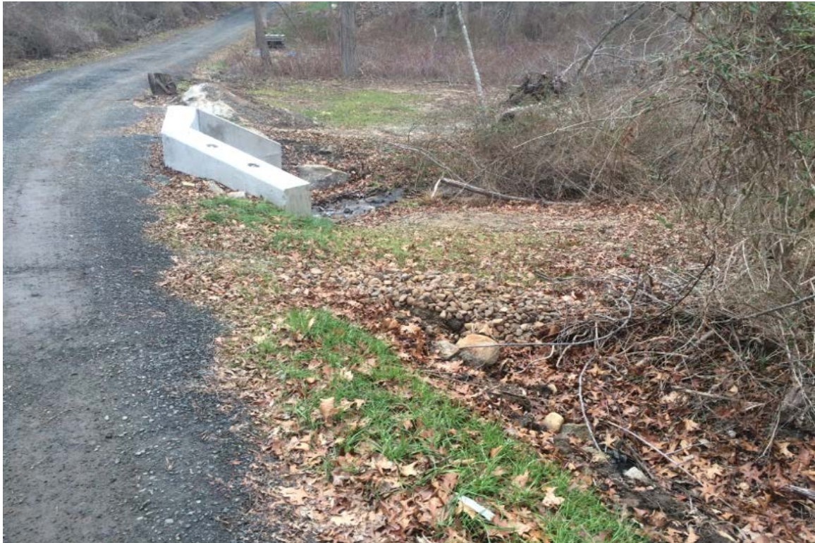
Photo 5: View of stabilized culvert crossing inlet looking west.
