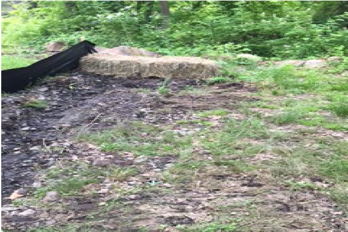
Photo 5: View of straw bales check dam near stream crossing, looking west.
