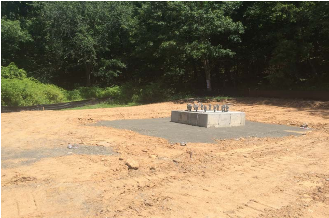
Photo 4: View of tower compound looking north.
