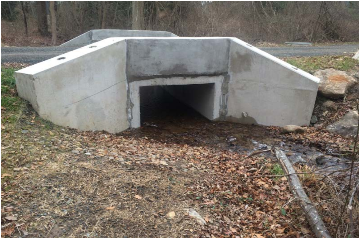
Photo 6: View of stabilized culvert crossing inlet looking north.
