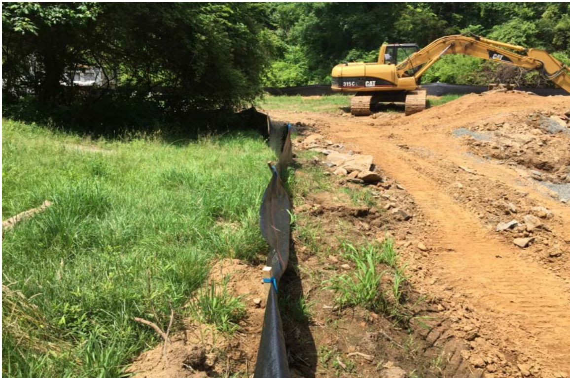
Photo 4: View of silt fence properly buried looking west.
