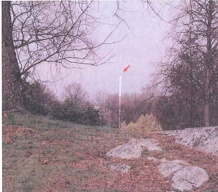
Figure 17: Photo of existing AT&T tower from Byram Park. (Cellco 1)
