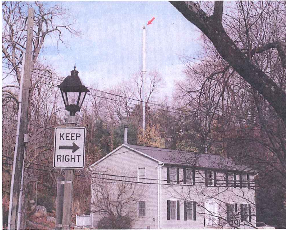
Figure 11: Photo of existing AT&T tower from Ritch Ave west of Byram Park entrance.
