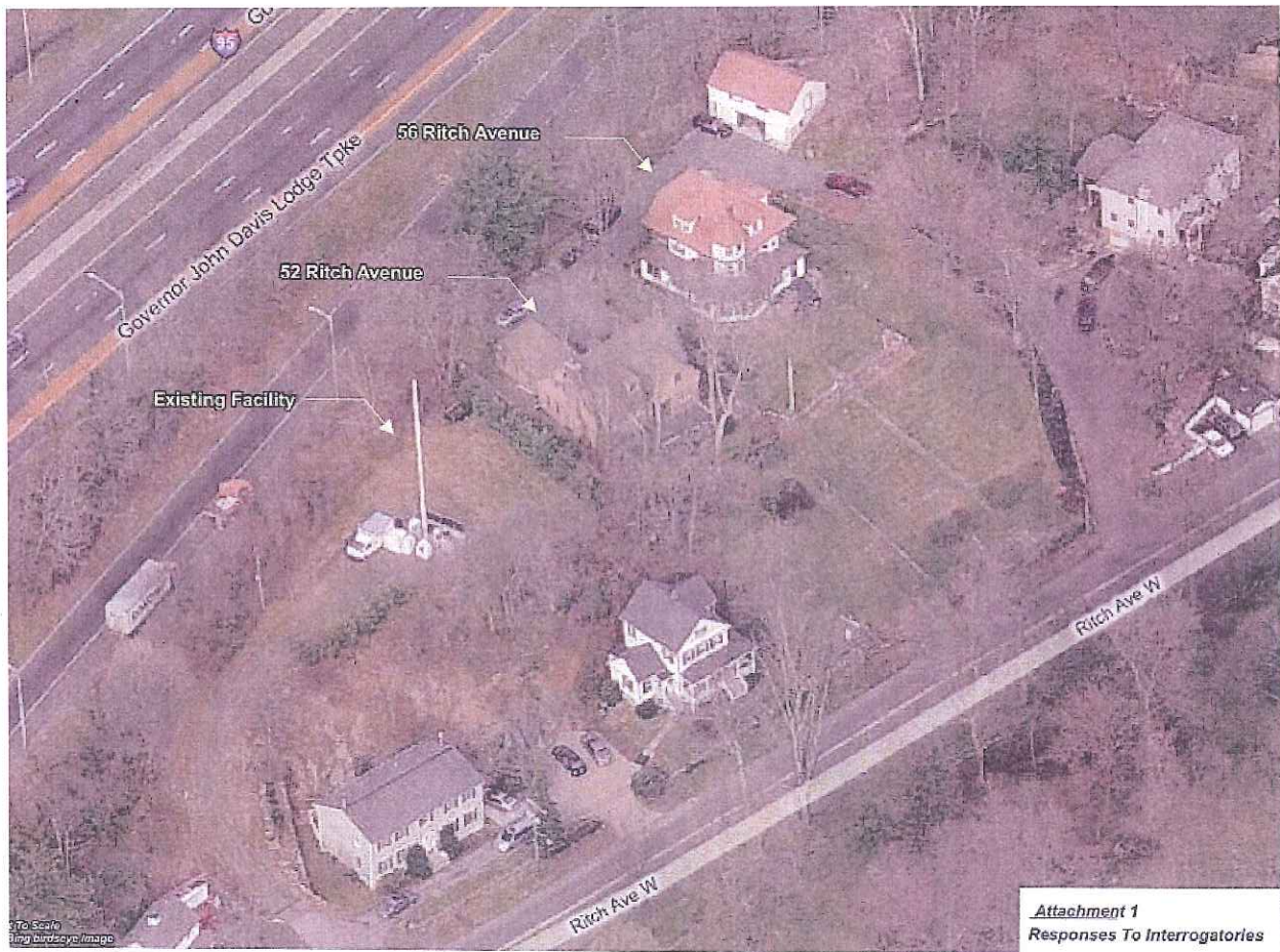
Figure 9: Site location showing existing AT&T tower. (Cellco 4, Attachment 1)
