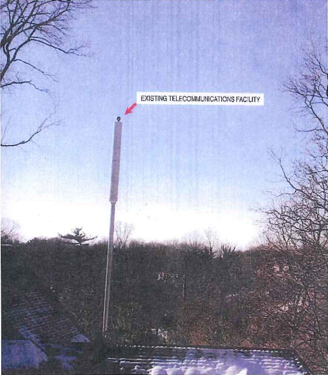
Figure 15: Photo of existing AT&T tower from second floor of 56 Ritch Ave.
