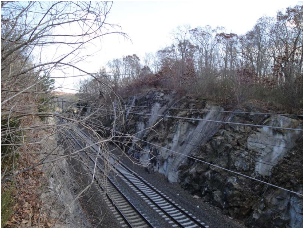
Photo 8: View of Amtrak rail line near proposed Facility, looking east.
