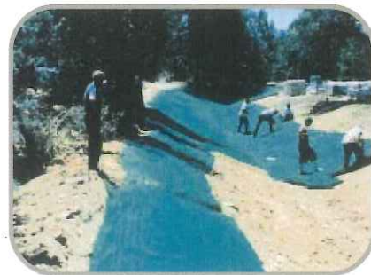
June, 1995 Installation of Landlok® TRM 450
