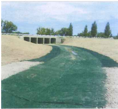
FIG.1: PYRAMAT & LANDLOK 450 INSTALLED
