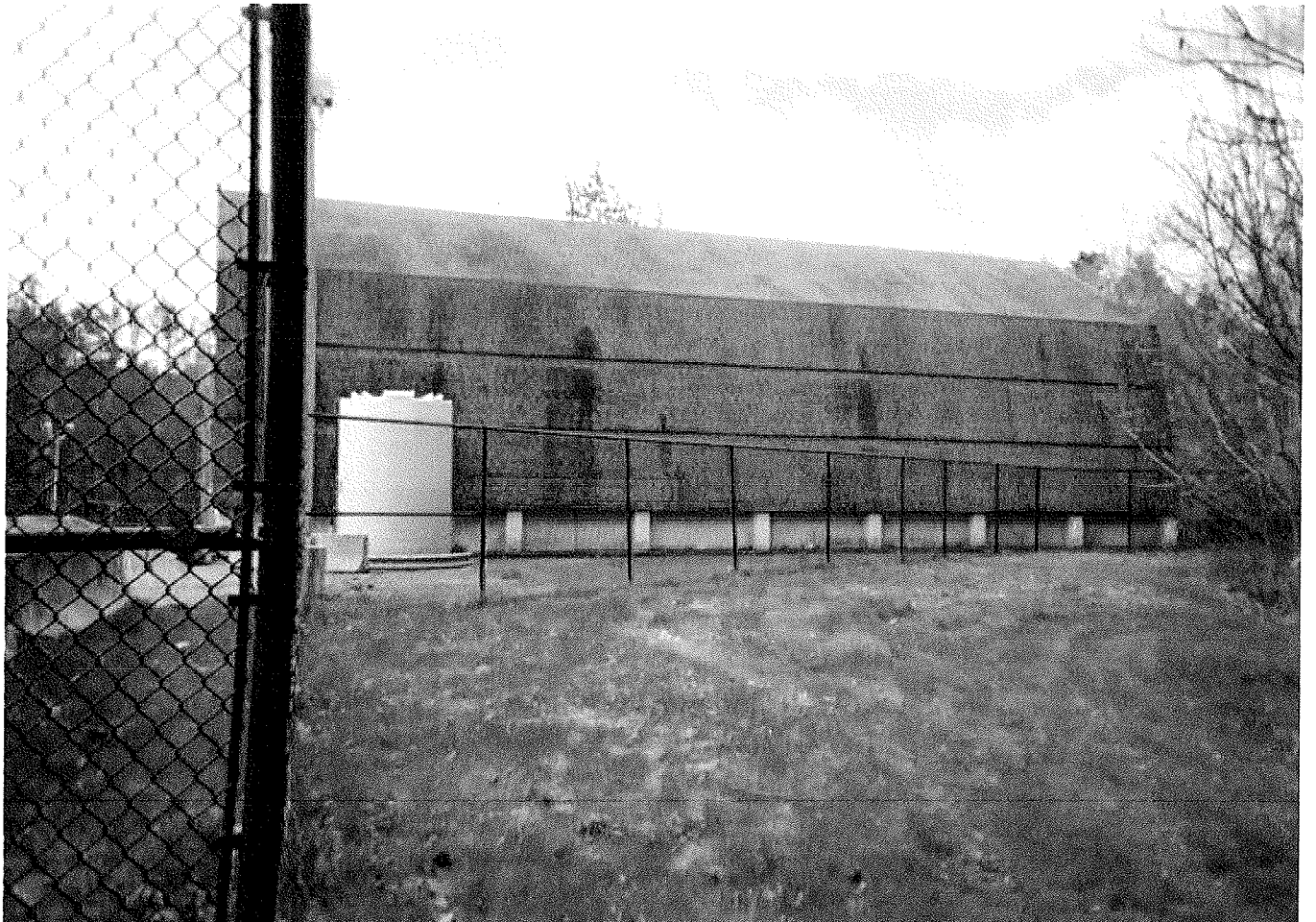
Connecticut Department of Transportation Salt Garage
