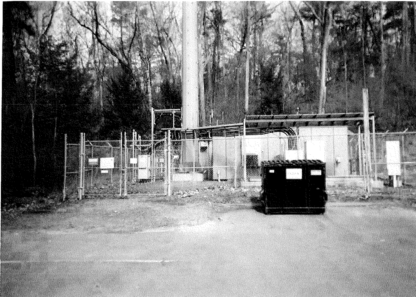
Granby Center Tower
