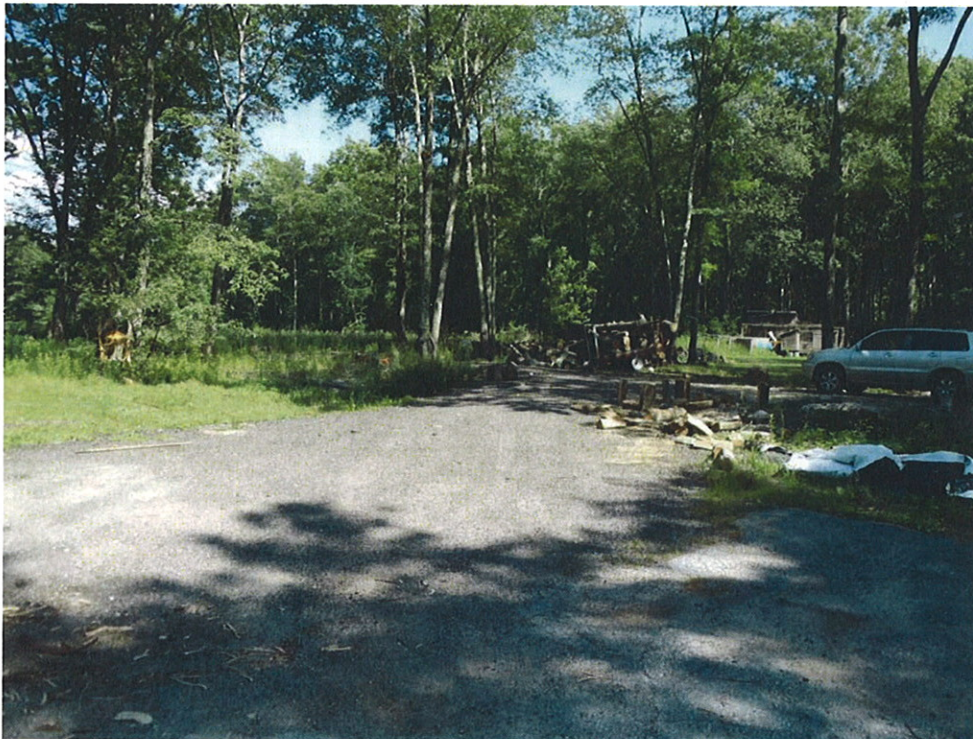
Photo 2: View of proposed access/existing gravel drive where it diverges from existing paved driveway, looking southeast.
