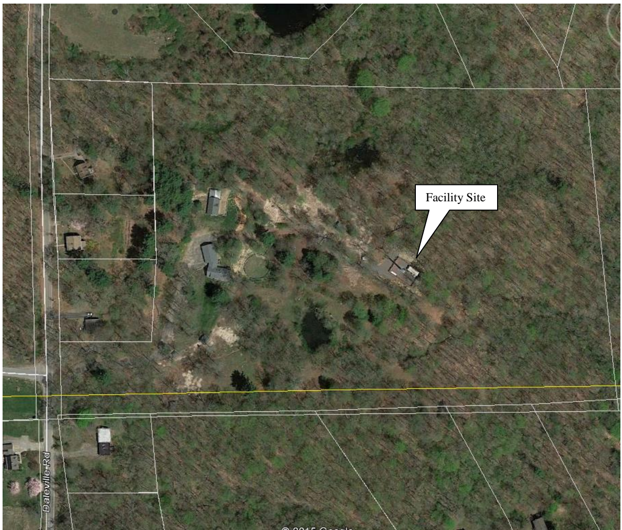
Site - 343 Daleville Road, Willington. 105-foot monopole. (May 2015 google earth image)
