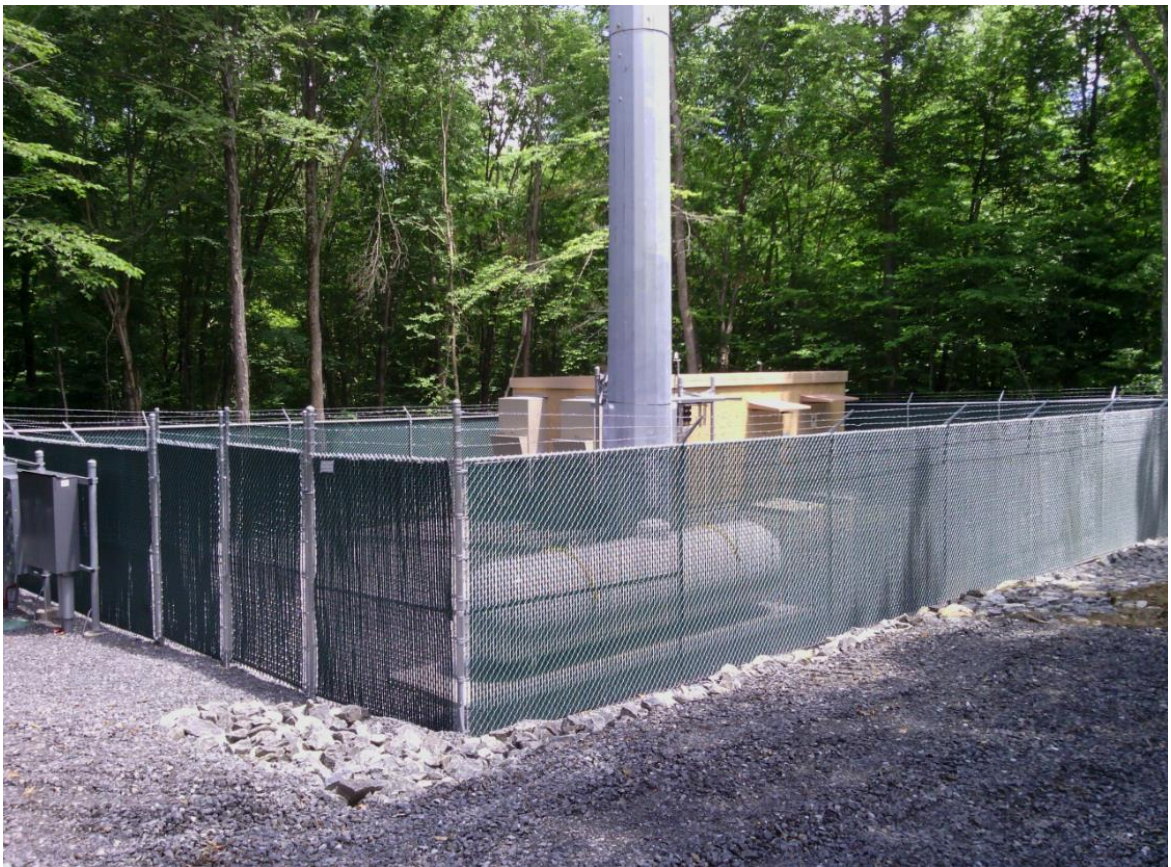
Compound area, west corner.
