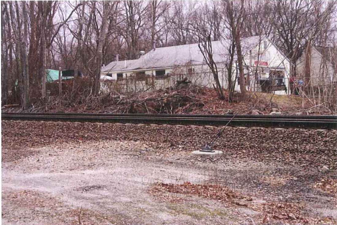
Photo 3: Close view of laundromat building, looking northwest.
