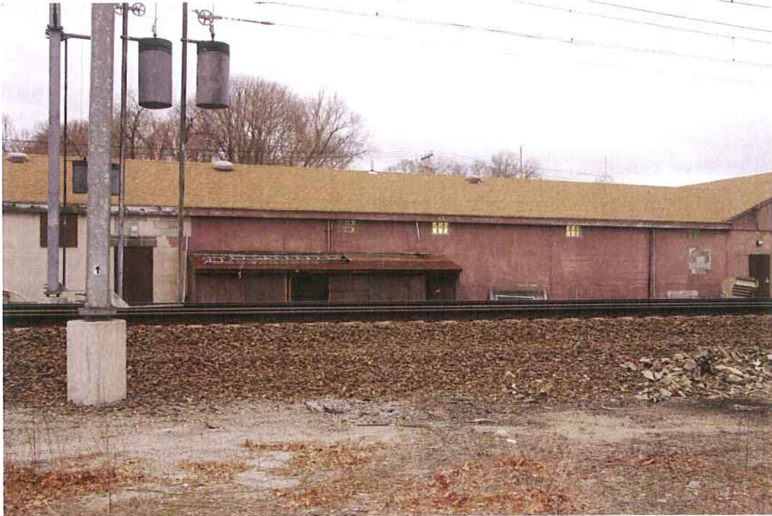
Photo 5: View of central portion of adjoining commercial building east of laundromat building, looking north.
