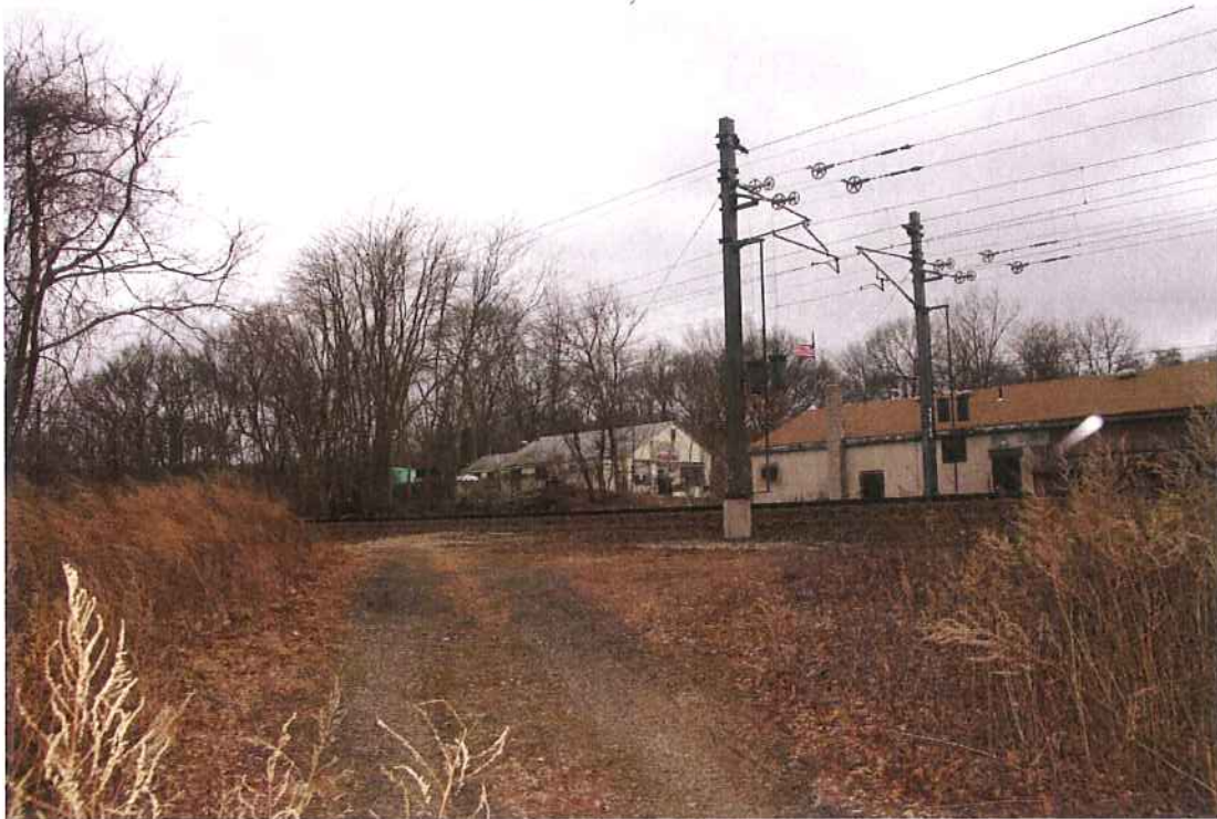
Photo 1: Overview of Laundromat Site (building to the left across railroad tracks), looking northwest from railroad maintenance access.
