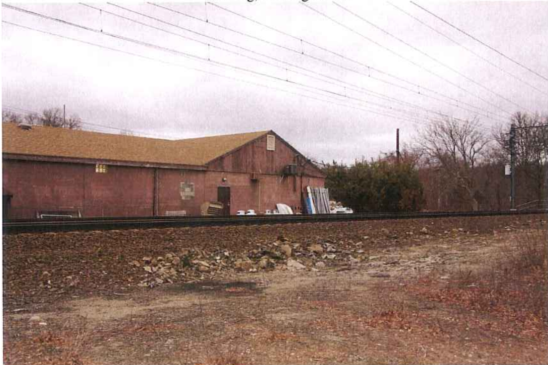
Photo 6: View of east end of adjoining commercial building east of laundromat building, looking north.
