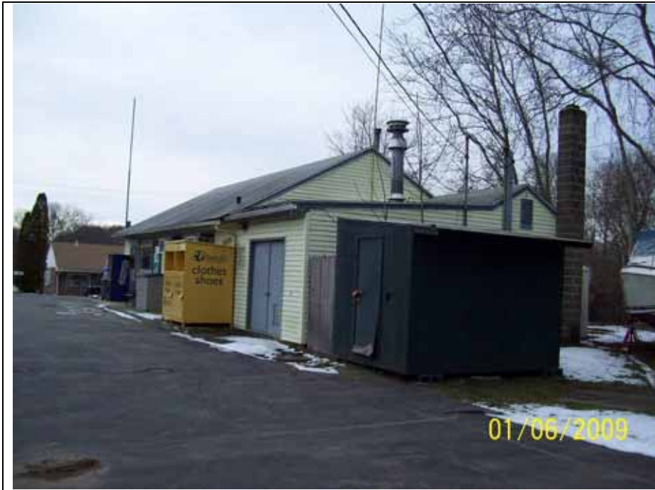
21. Facing east to Subject Property building
