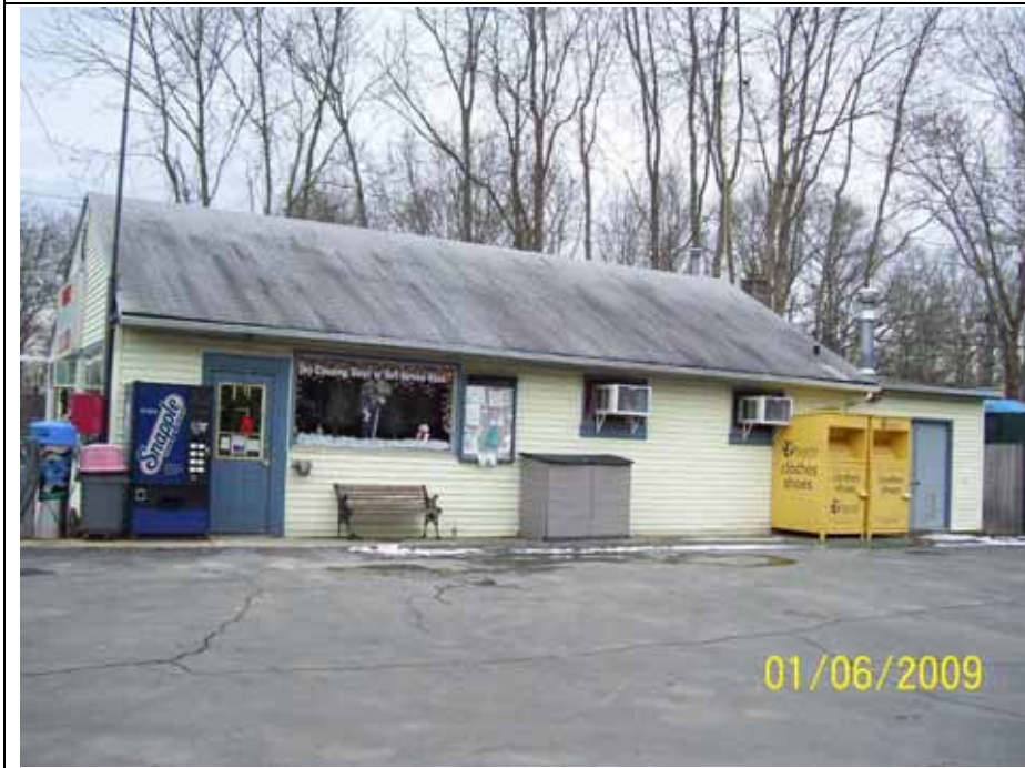
22. Facing south to Subject Property building
