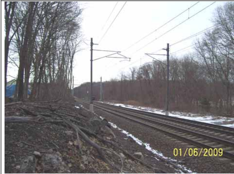
12. Facing east to railroad
