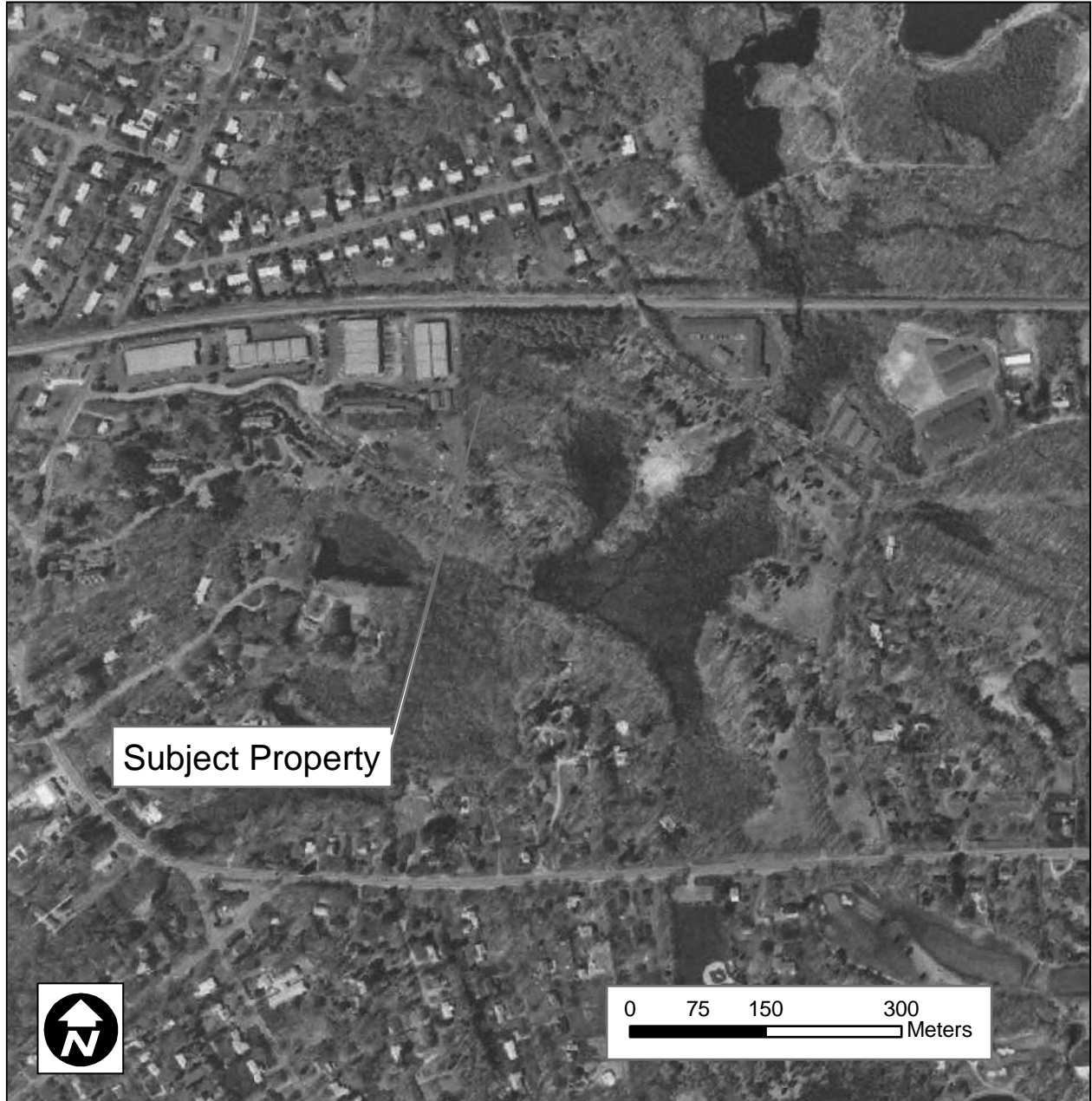
Figure 10. Excerpt from a 1995 aerial photograph depicting the Area of Potential Effect in Madison, Connecticut.
