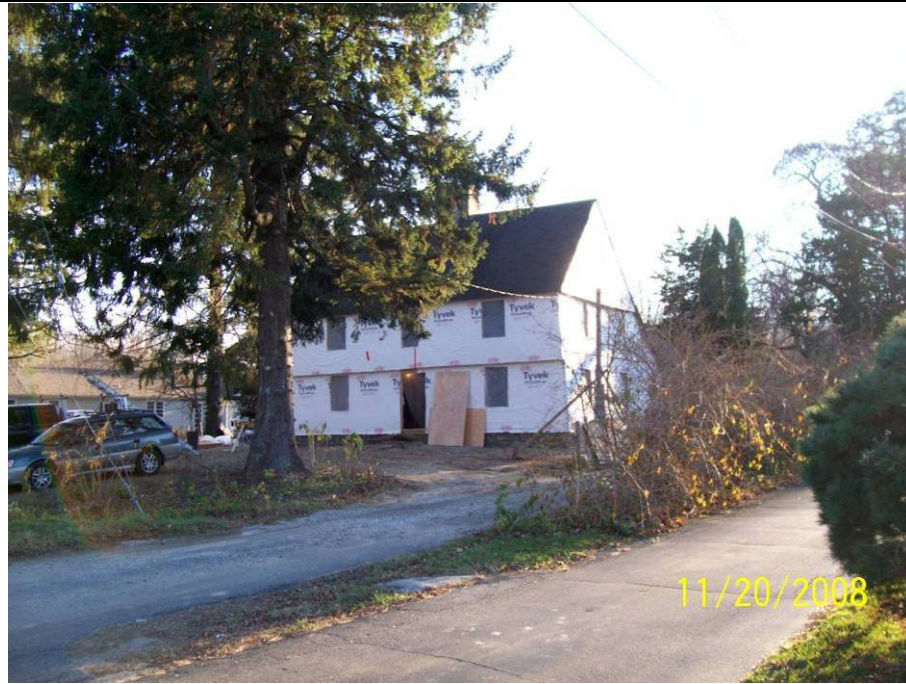
19. View of the Shelley House (248 Boston Post Road) looking south.
