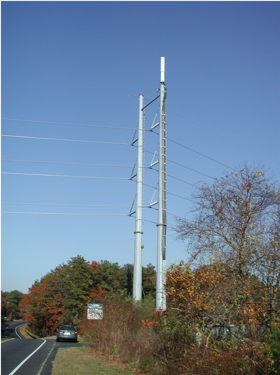
Three-Sector Wireless Antenna Canister, Barnstable Massachusetts
