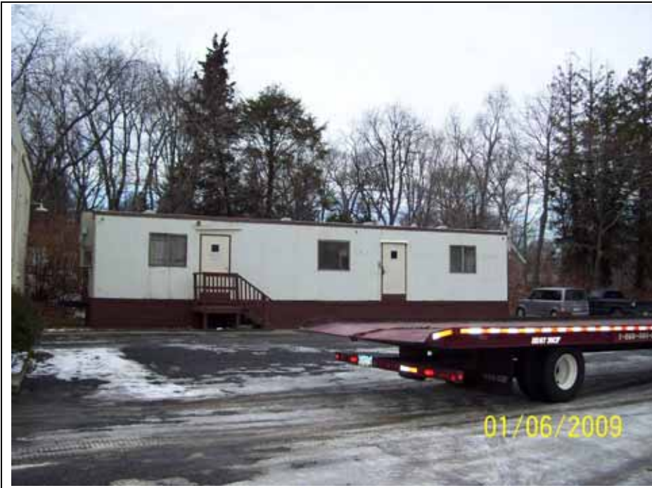
15. Facing northwest to Subject Property building
