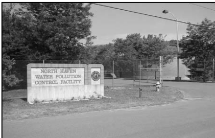
North Haven Water Pollution Control Facility
