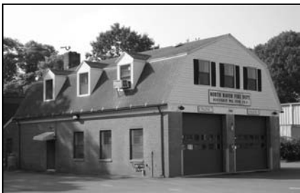
Northeast Fire Station (Company 4)
