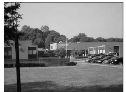
Clintonville Elementary School
