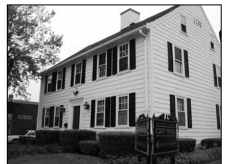
Converted Office Space
