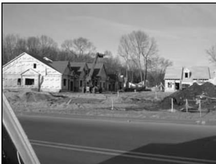
New Housing Construction
