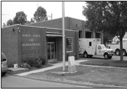
North Haven Fire Department Headquarters (Company 1)
