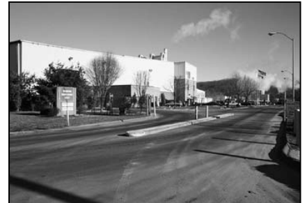
Wallingford Resource Recovery Facility
