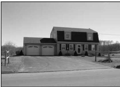
Recent Single Family Construction, Sugar Hill Road
