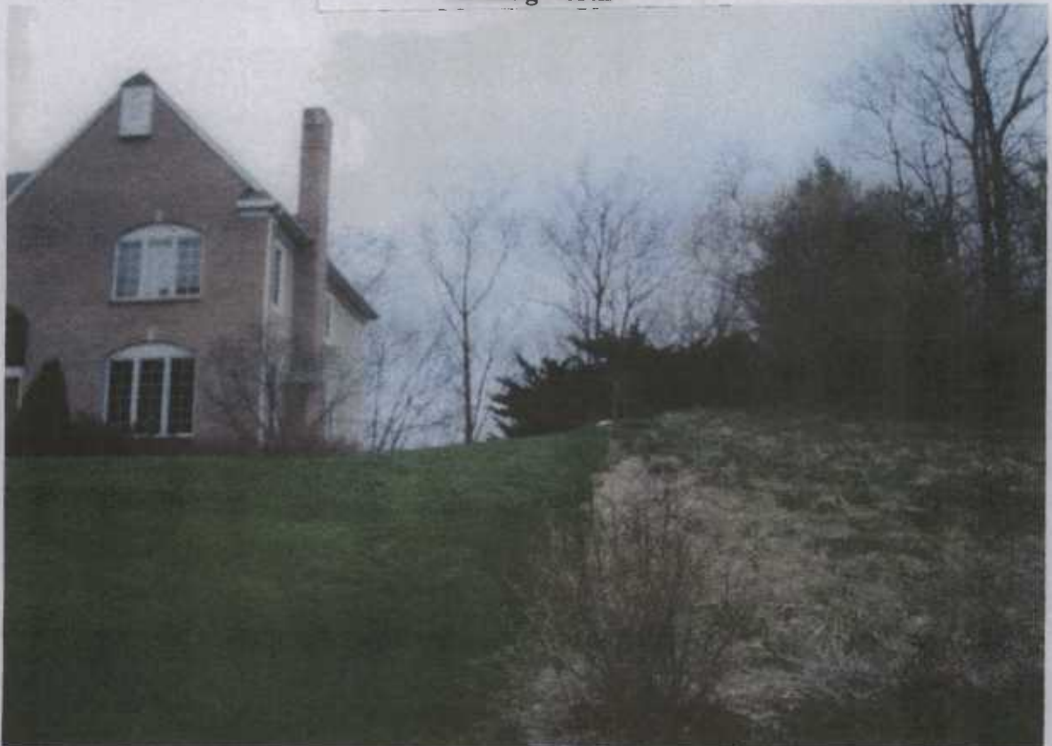
From Access Drive & Brian Rd. Looking East
