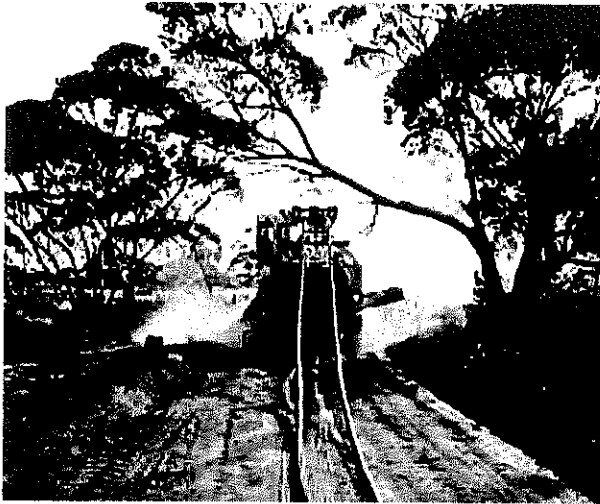
Construction of Murraylink HVDC Light® (Australia).
